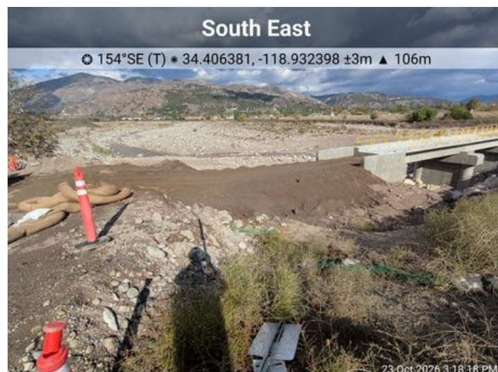
Figure 1. Image of Sespe Overflow Railroad Bridge West Abutment on Oct. 23, 2026
