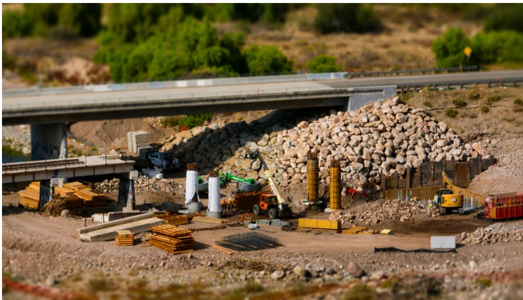
Figure 1. Aerial Image of Sespe Overflow Railroad Bridge on August 26, 2026
