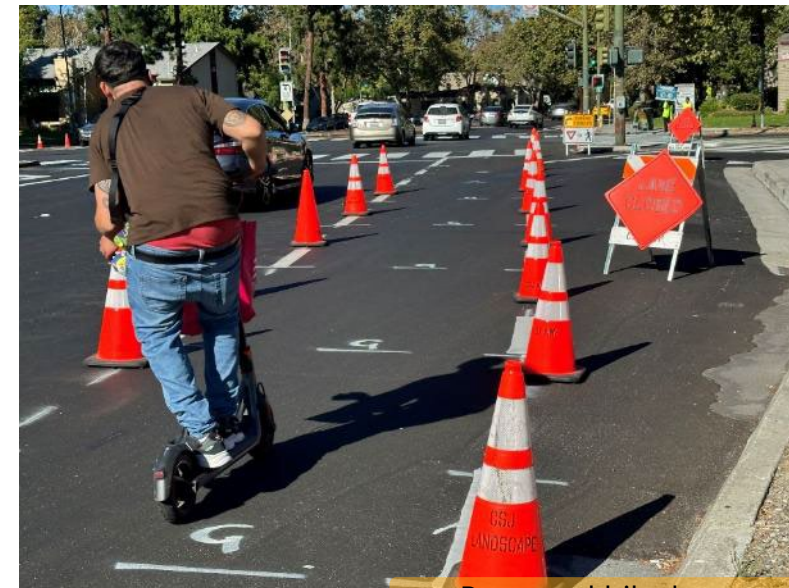
Protected bike lane
