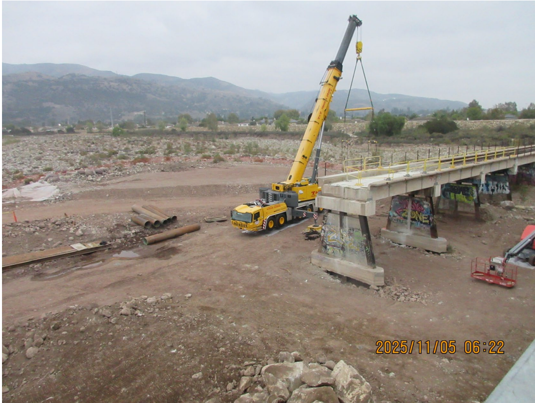
Before: 11/5 – Pier Demo & Girder Removal
