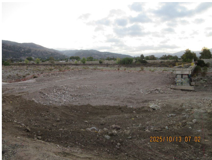
Figure 1 – Sespe Creek Overflow After Water Diversion Installed and Fish Protection Plan Implemented
