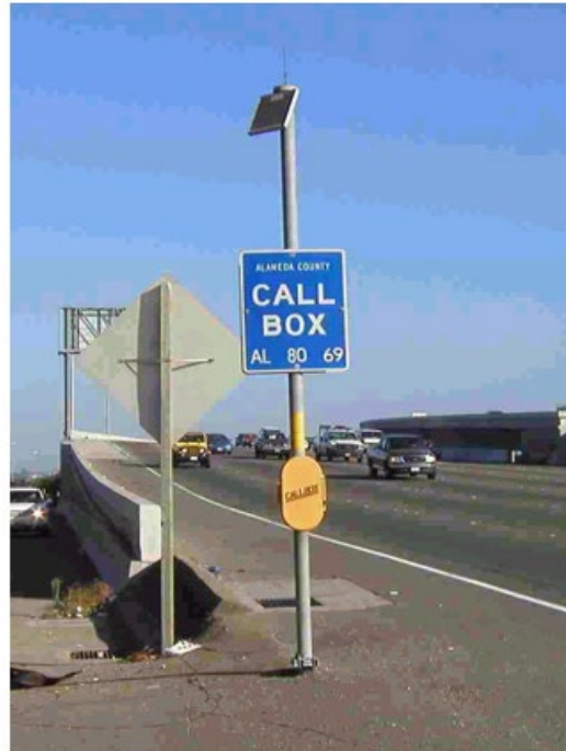
Site Type G – installed at-grade, in concrete.
