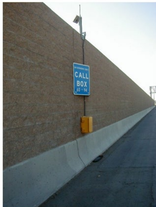
Site Type D – mounted on a soundwall.
