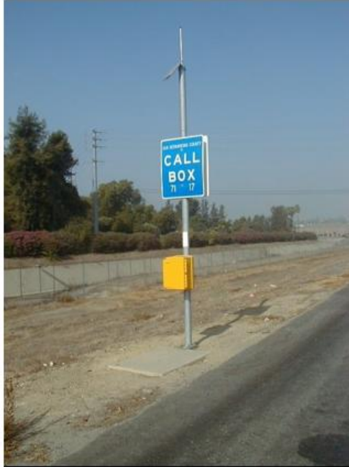
Site Type A – installed at-grade, in soil.
