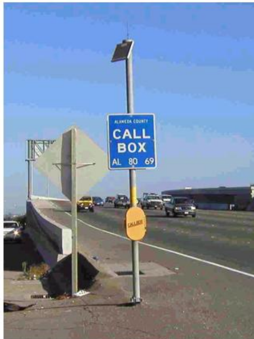
Site Type G – installed at-grade, in concrete.
