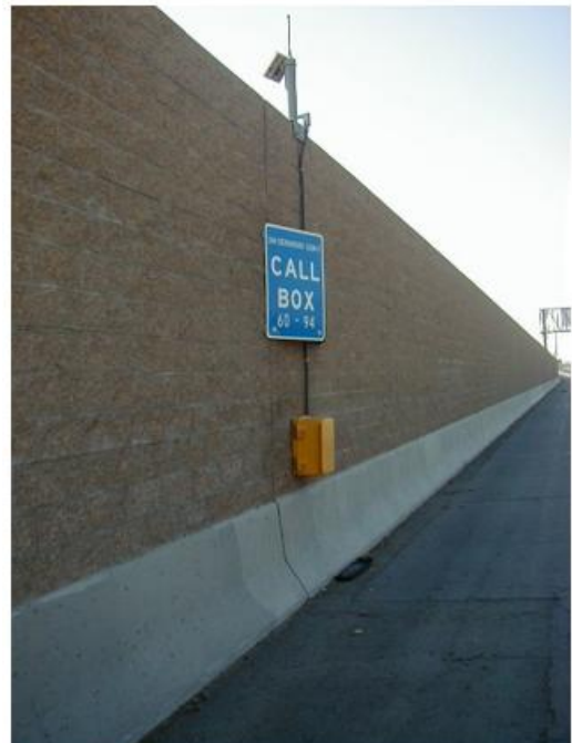
Site Type D – mounted on a soundwall.
