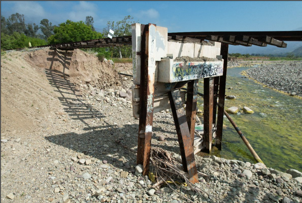
Photo #3. View of damaged abutment and newly replaced Old Telegraph Road Embankment on the left.
