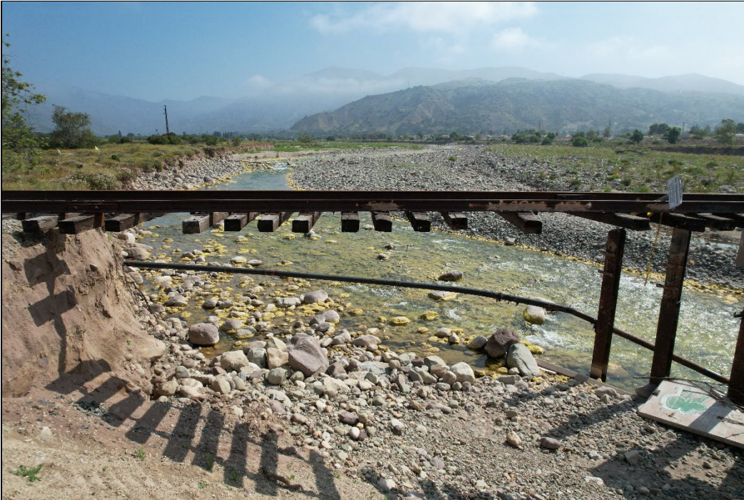
Photo. #2 View facing east at the 50+ feet of embankment behind the abutment that will be replaced to align with the Old Telegraph Road immediately behind this photograph.
