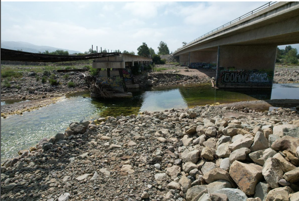
Photo #5 View looking south at the damaged piers and existing spans proposed to be reused in the final bridge repair. Rock rip rap will be buried around these two bents in order to support them during winter storms.
