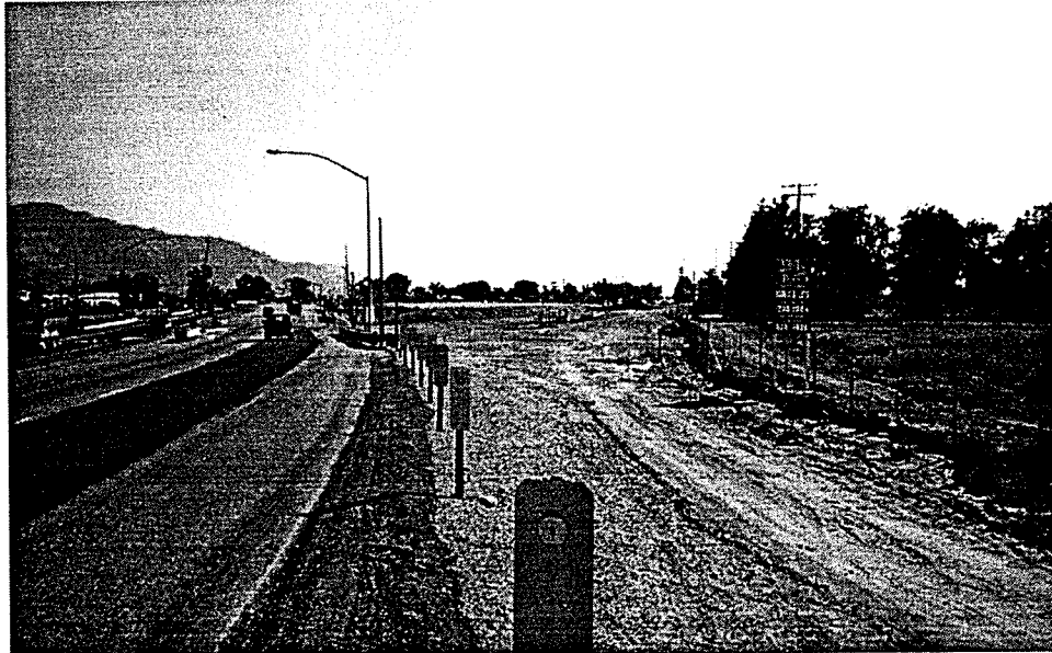
Figure 95. Existing Highway 126/Haun Creek Crossing
