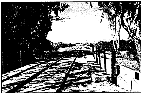
Existing Physical Trail Characteristic, Largo Lane Area
