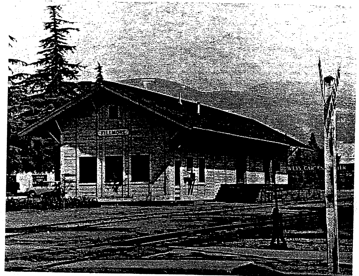
FILLMORE DEPOT, ORIGINAL LOCATION, SOUTH SIDE, c 1970
