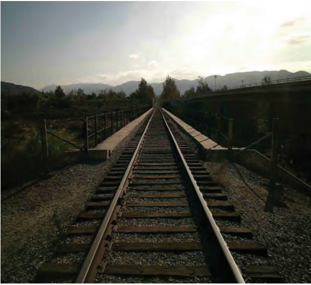
Bridge 423.44 Deck View
