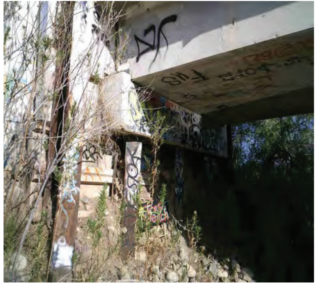
Bridge 423.44 Dump Bent
