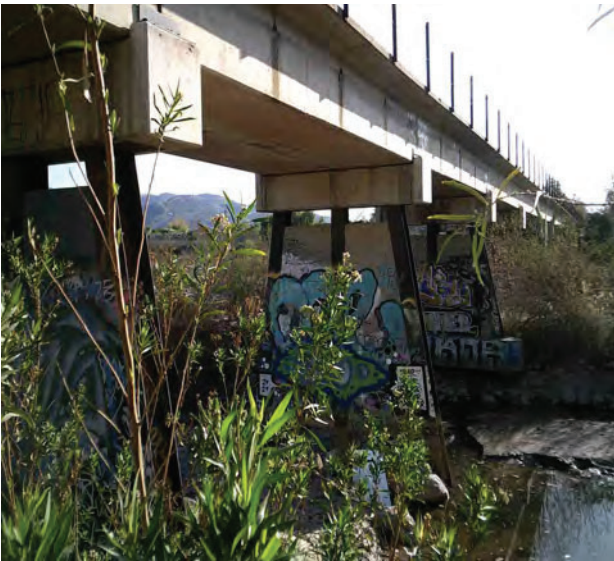
Bridge 423.44 Typical Bent
