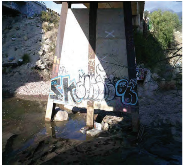
Bridge 423.44 Typical Concrete between Piles
