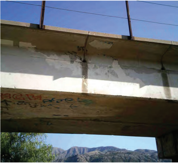
Bridge 423.44 Typical Span
