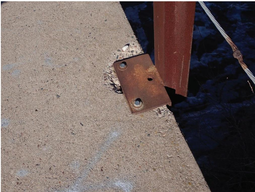
**423.44 Handrail embed failed. Post held with bolts, Span 3, 4 and 15**
