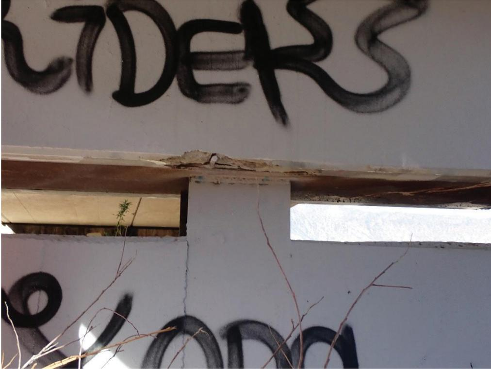
**423.44 Spall with exposed rebar – Pier 14 East side**
