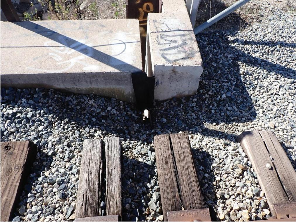
**423.44 Ballast leaking onto bearing seats, Abutment 1**
