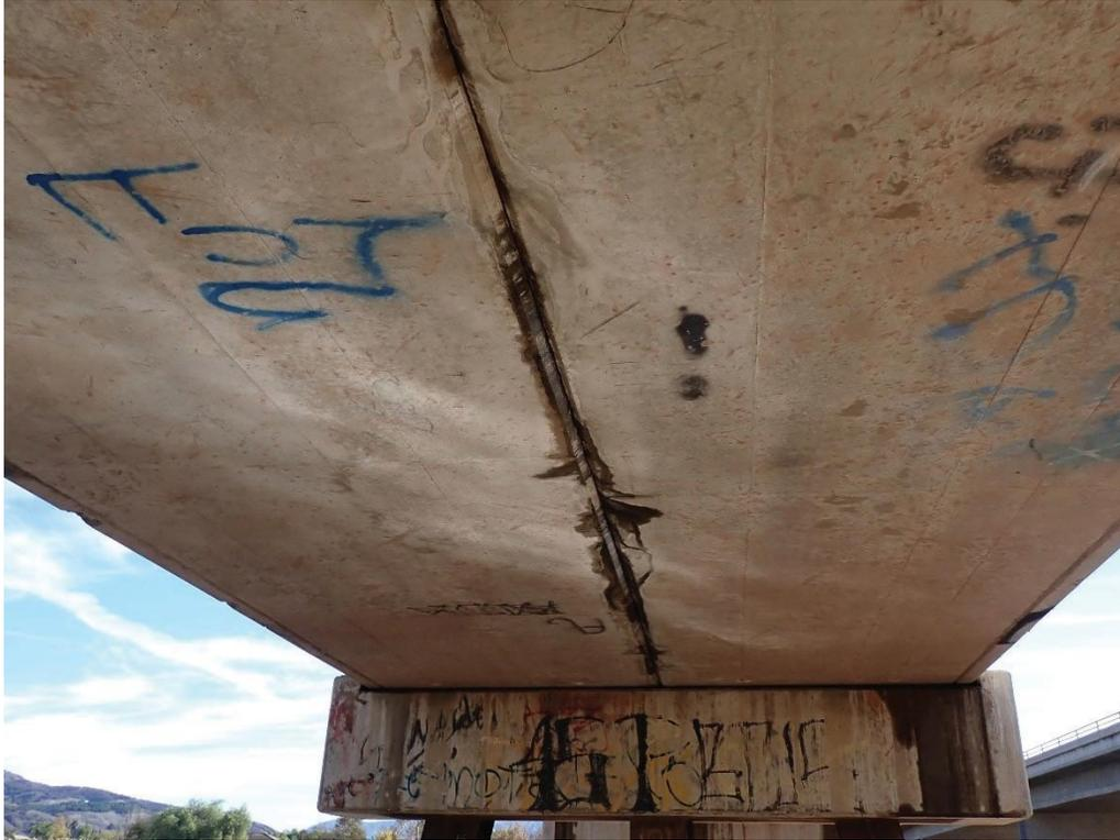
**423.44 Spall with exposed rebar between Girder 1 and 2, Span 1**
