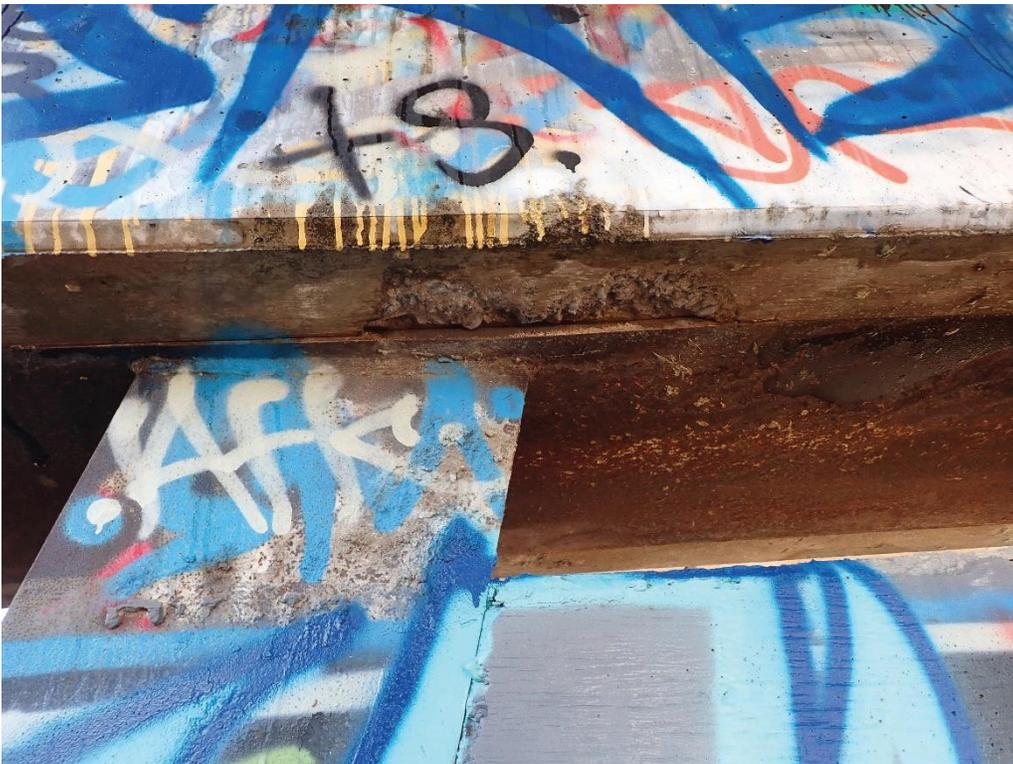
**423.44 Small spalls on the underside of cap at Pier 7**
