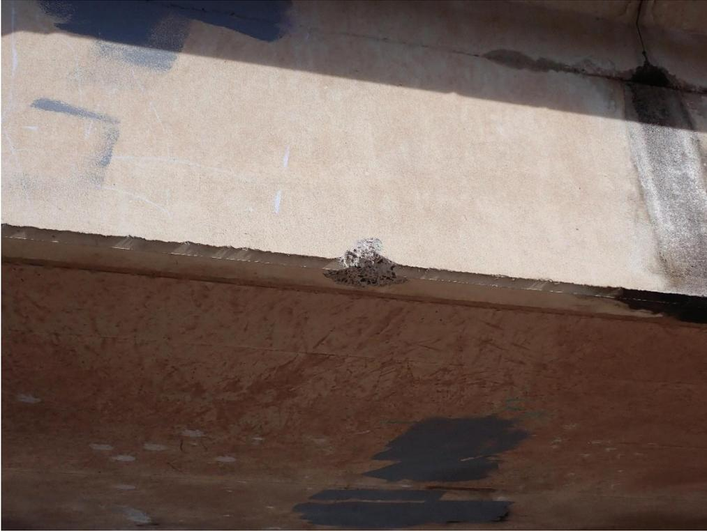
**423.44 Minor spall midspan, Span 11**
