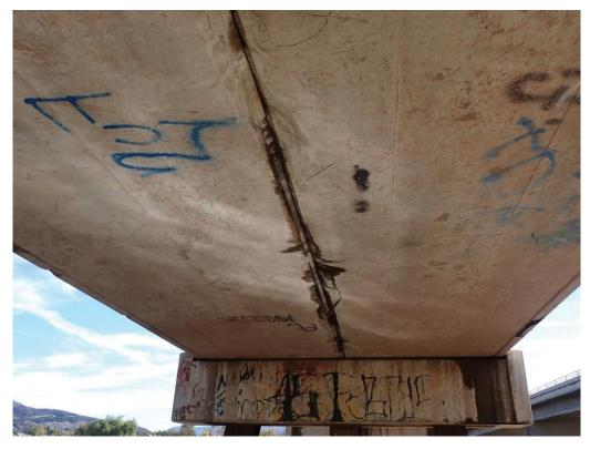
423.44 Spall with exposed rebar between Girder 1 and 2, Span 1
