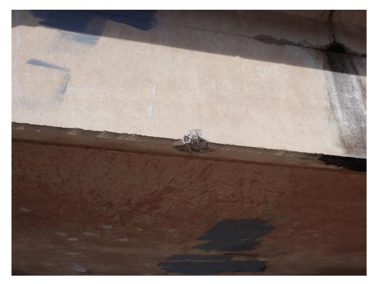
423.44 Minor spall midspan, Span 11
