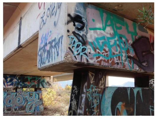
423.44 Minor spall on bottom corner of pier cap, Pier 6
