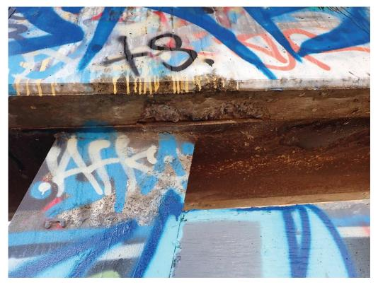
423.44 Small spalls on the underside of cap at Pier 7
