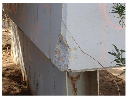
423.44 Spall NE bottom corner of cap, Pier 14
