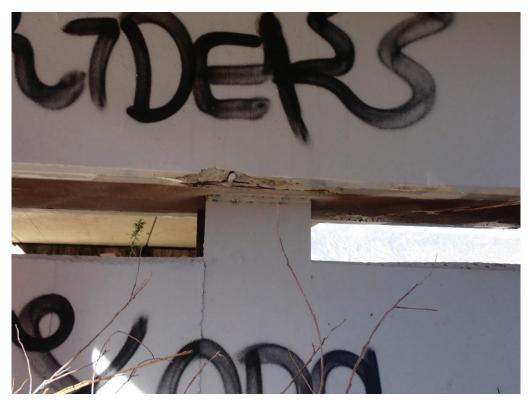
423.44 Spall with exposed rebar – Pier 14 East side
