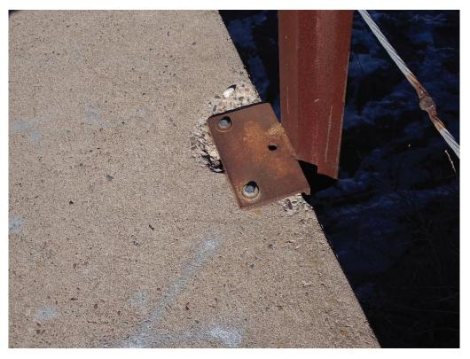
423.44 Handrail embed failed. Post held with bolts, Span 3, 4 and 15
