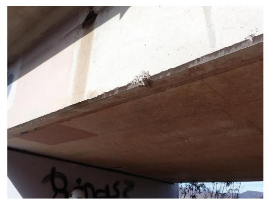
423.44 Span 15 impact damage
