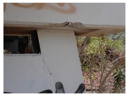
423.44 Spall along underside of cap with exposed rebar – West side Pier 15
