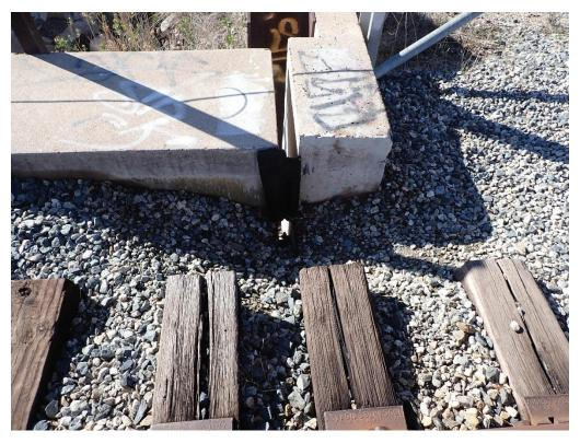
423.44 Ballast leaking onto bearing seats, Abutment 1
