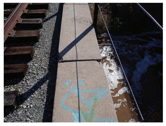
423.44 Walkway spall on Span 2 and multiple locations
