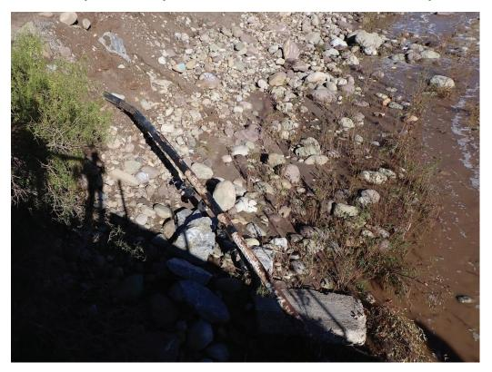
423.44 Deep erosion from heavy water on Northwest slope
