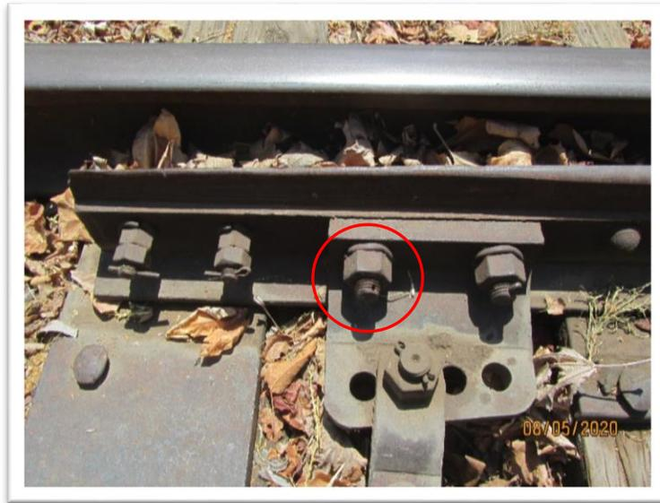
Image 99. Switch 3860 Missing Cotter Pin
