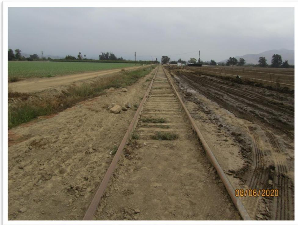
*Image 6. MP 408.3 Erosion / Poor Ballast*
