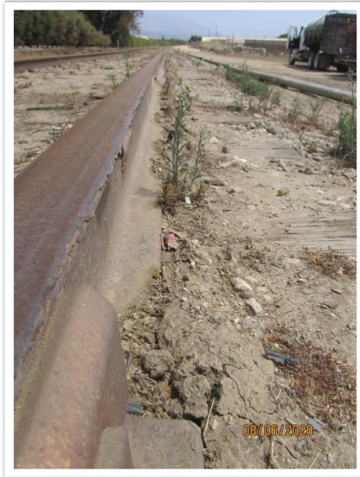
*Image 13. Rail Opposite Gauge Side Shell Showing Parent Metal Decay, MP 411.10*
