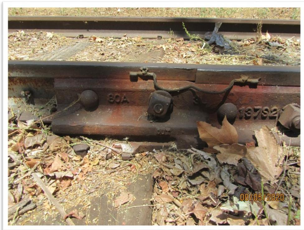
*Image 15. Rail joint matching rail sizes, MP 408.0*
