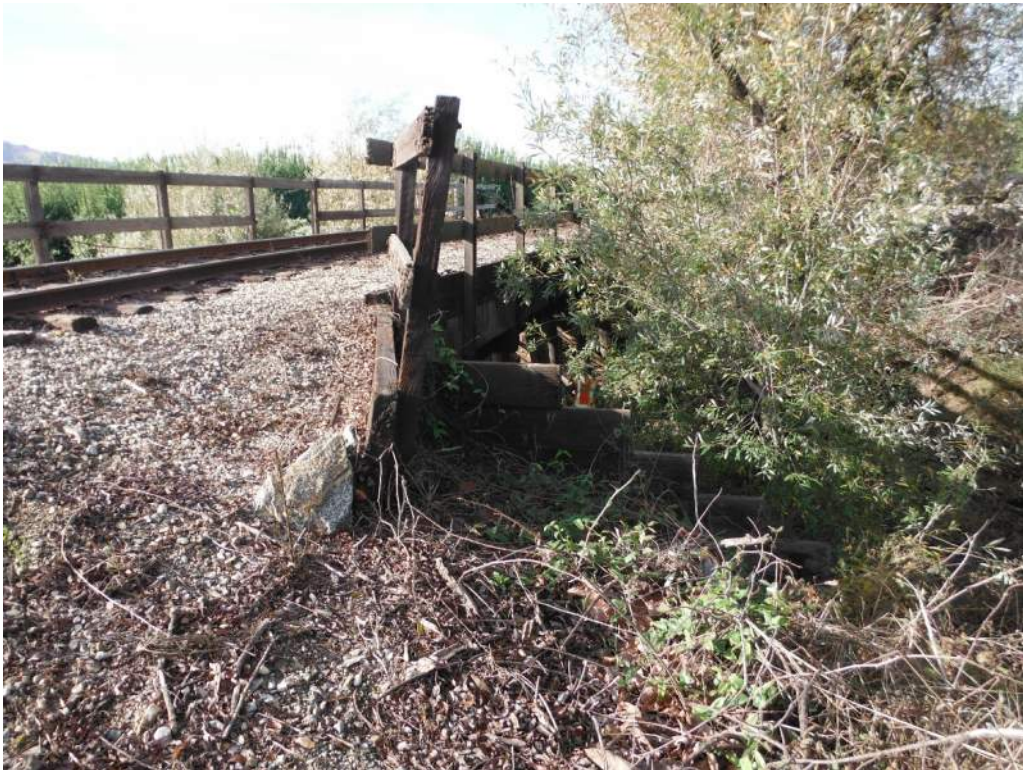
417.24 Handrail leaning with gap at end of bridge
