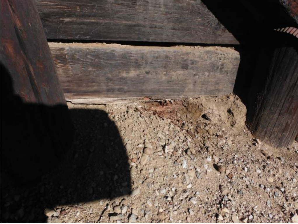
420.20 Abutment 5 rotten backwall
