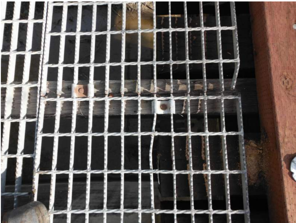
410.40 Grating causing tripping hazard
