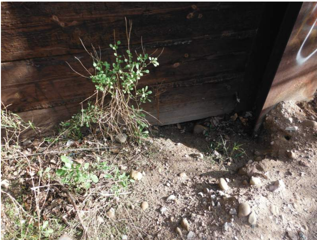
408.84 Abutment 6 Southeast Backwall undermining
