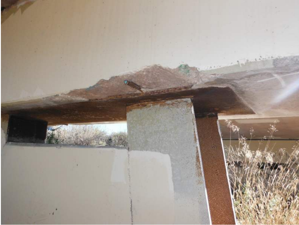
423.44 Spall along underside of cap with exposed rebar – west side Pier 14
