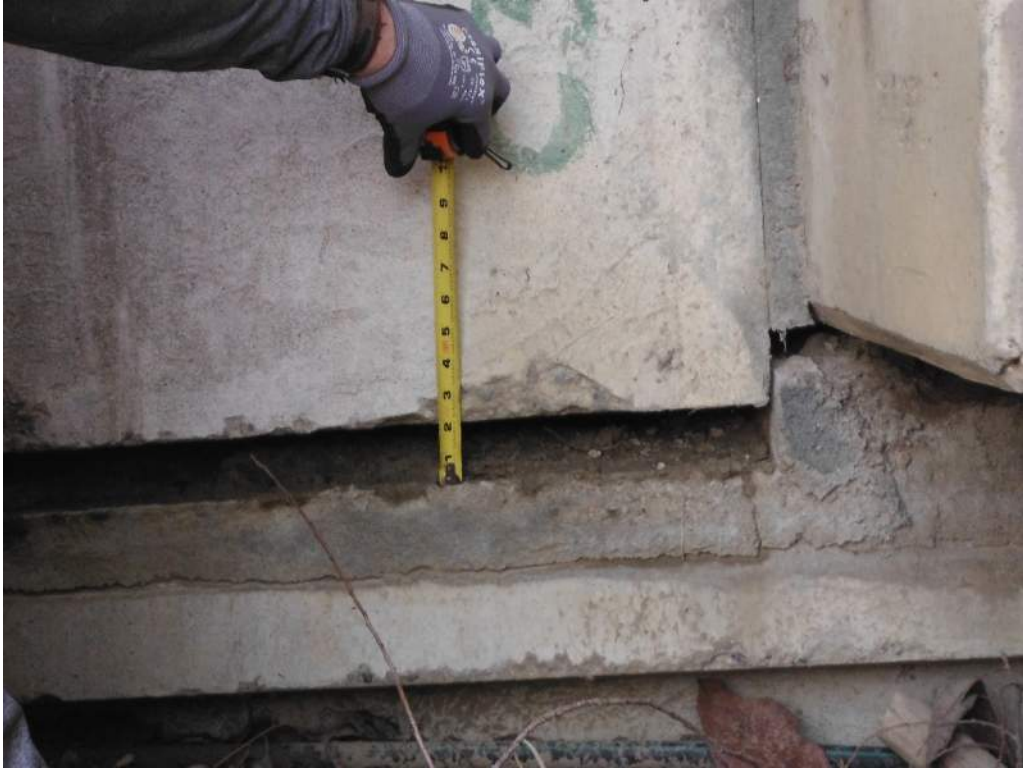
411.97 2" gap between Abutment 1 and wingwall
