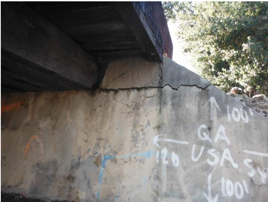
421.05 Abutment stringer retainer cracked – typical all 4 corners
