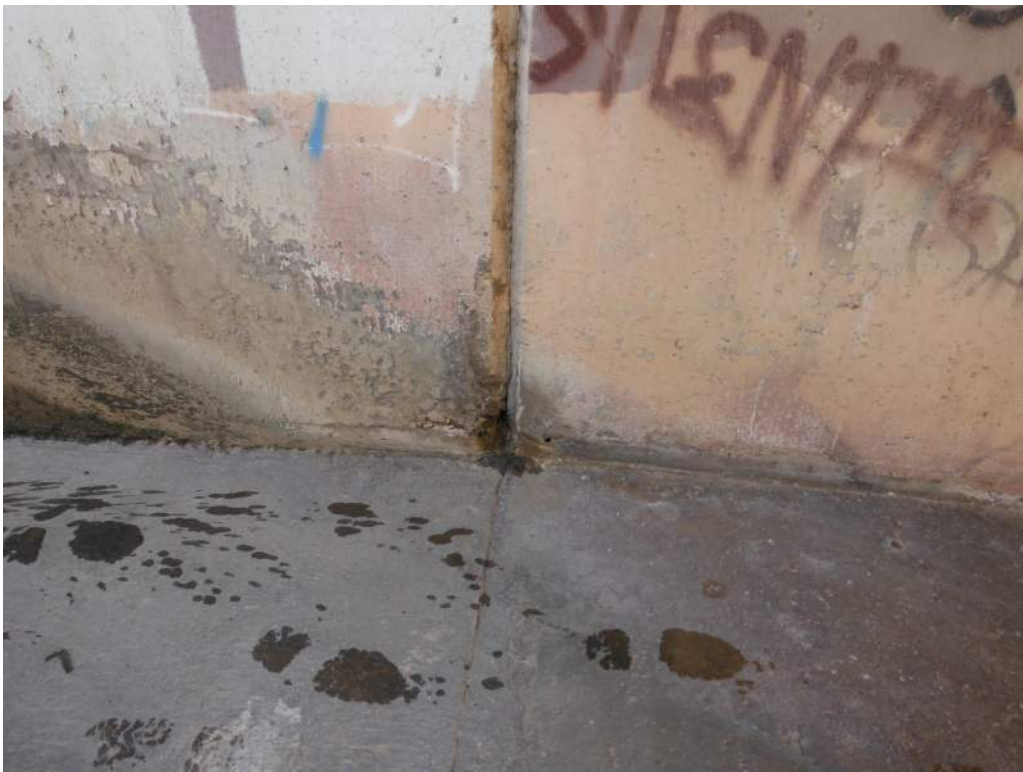
408.02 Spall at NE wingwall
