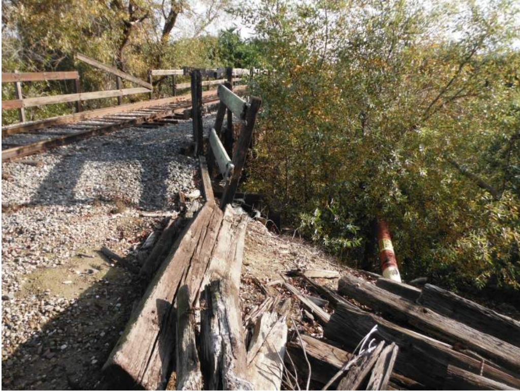
417.24 Southwest ballast retainer leaning – ballast leaking
