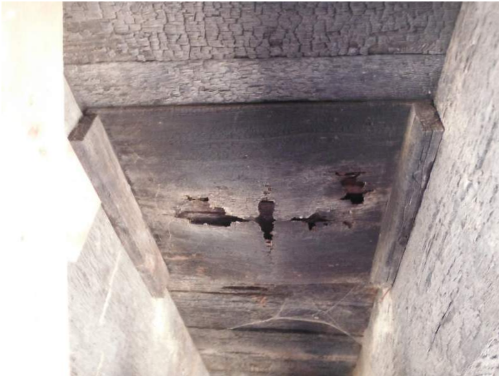
420.20 Failing Deck Plank – Span 4
