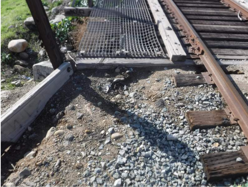
415.32 Hole in Ballast, SE Corner
