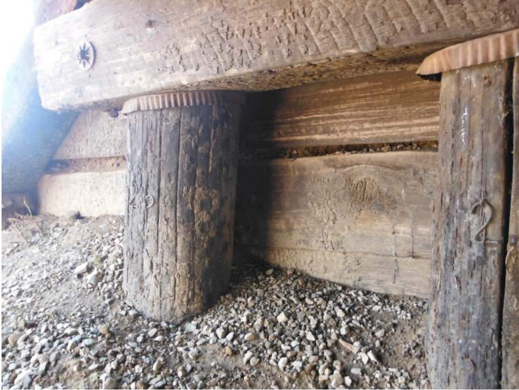
420.20 Abutment 1 rotten backwall
