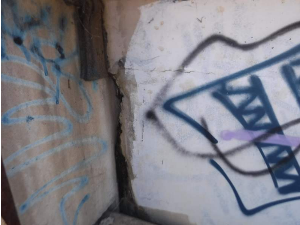
425.15 Crack and spall in girder near Abutment 3 north side
