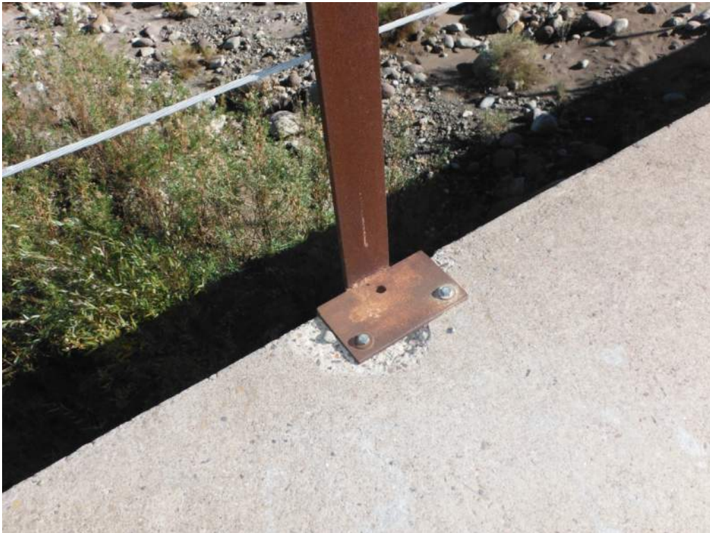
423.44 Handrail embed failed. Post held with bolts, Span 3 and 4
