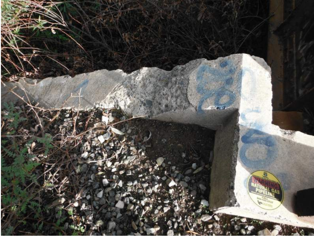
412.25 Spalling on wingwall – see report for locations
