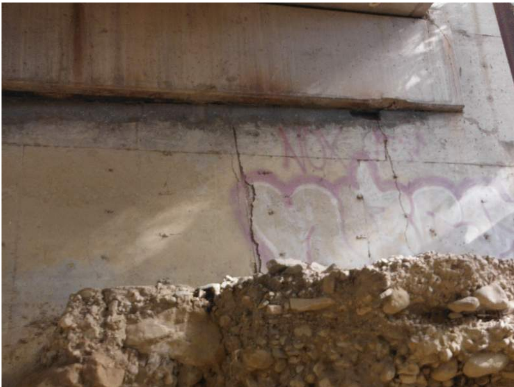
419.42 Cracking and spall with exposed rebar - Abutment 2
