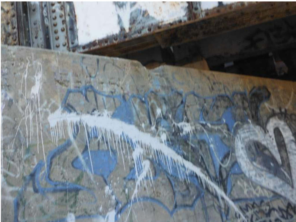
429.79 Spall under bearing – Pier 2
