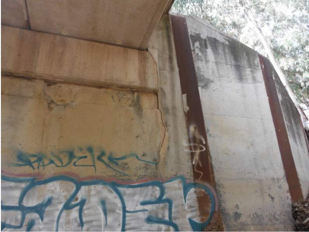
419.42 Abutment 1 crack and keeper block cracked – North edge of cap
