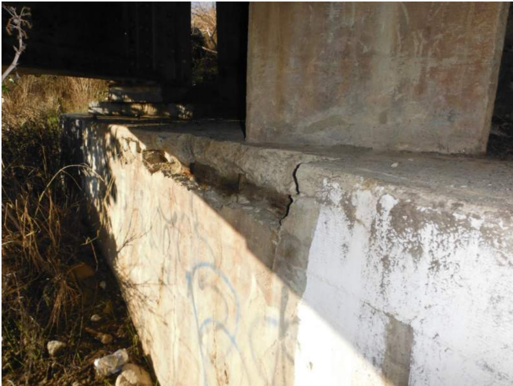
429.79 Spall - Abutment 1
