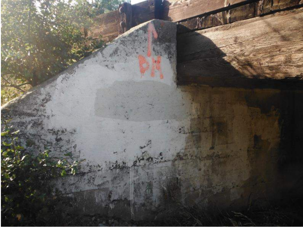
415.69 Cracks in Southwest Wingwall
