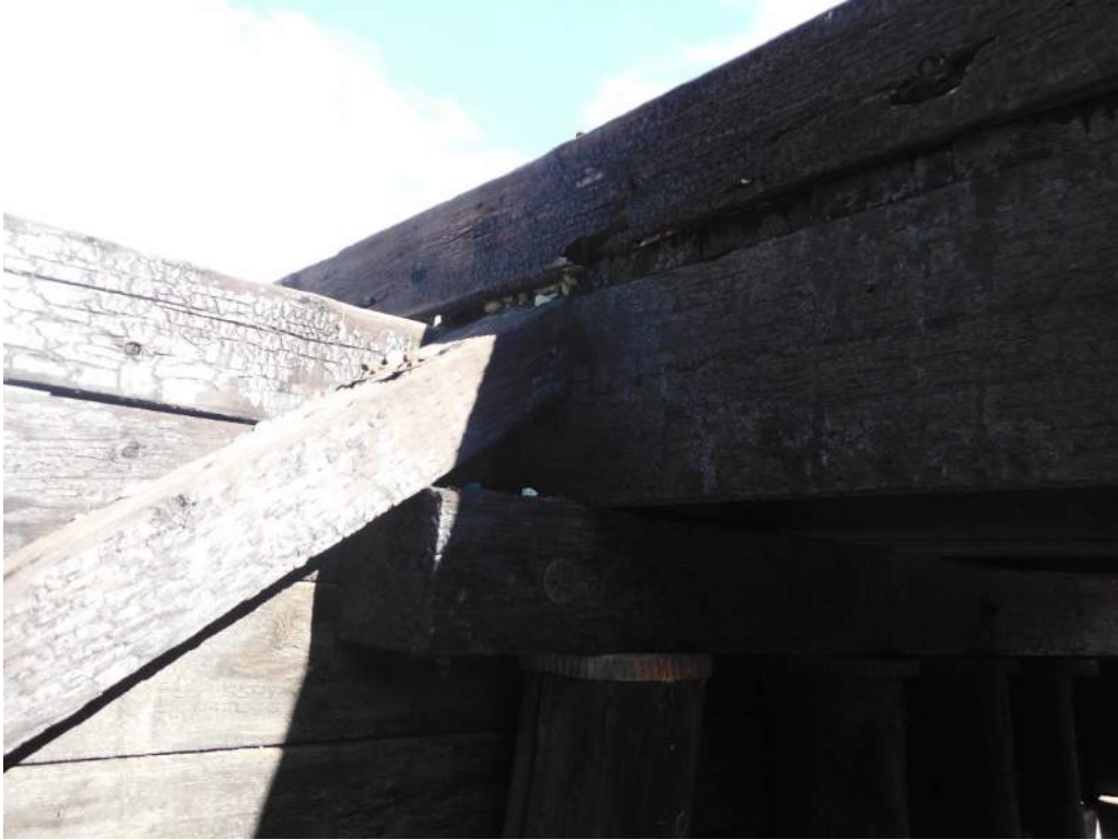
420.20 Ballast boards failing at Abutment 5
