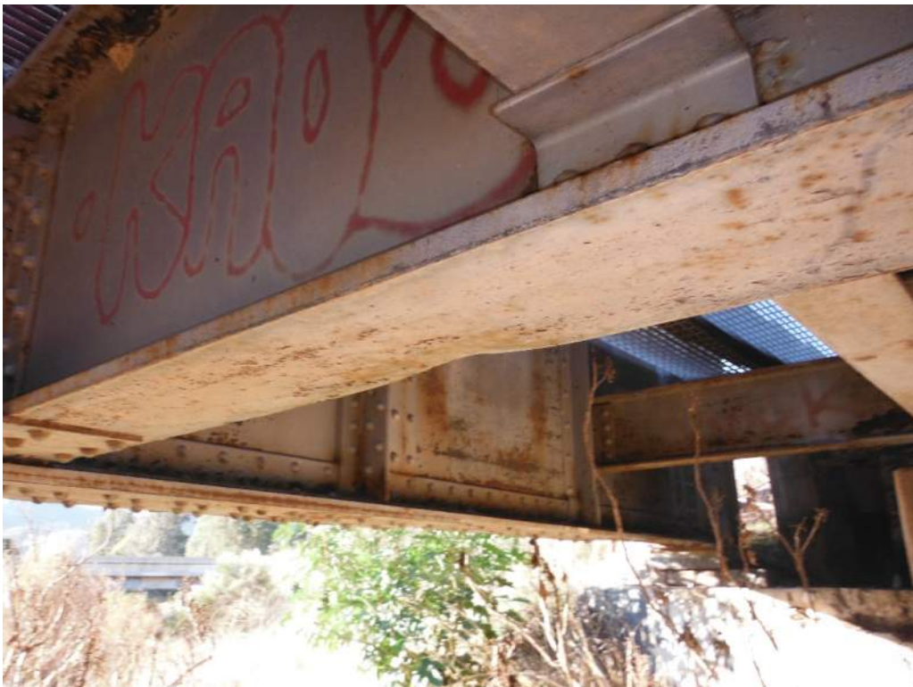
429.79 Impact damage to bottom flange floor beam 1 – Span 1
