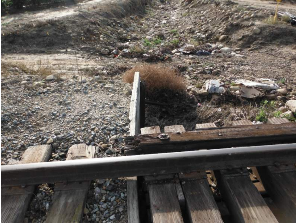
416.63 Backwall leaning - Abutment 1 & 2
