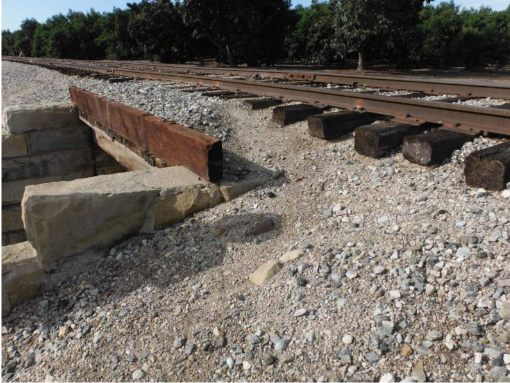
418.02 Low shoulder ballast at SE approach
