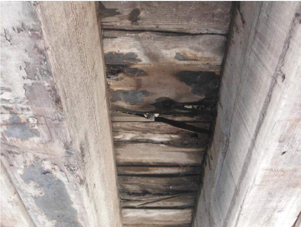
415.69 Decay of deck ballast plank. Mid-span, Span 3
