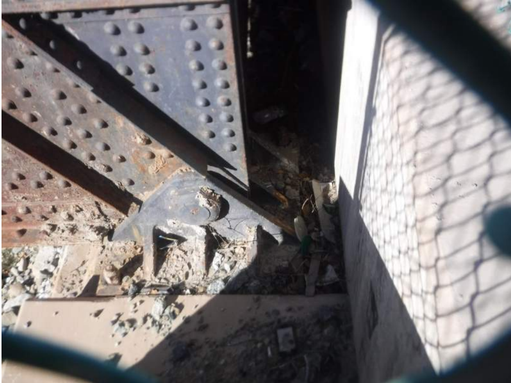
415.59 Debris at SE Bearing
