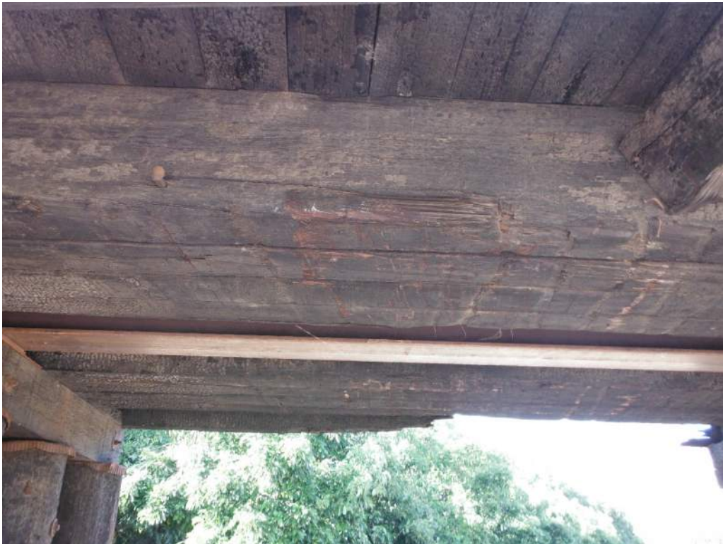
420.20 Impact Damage – Span 3
