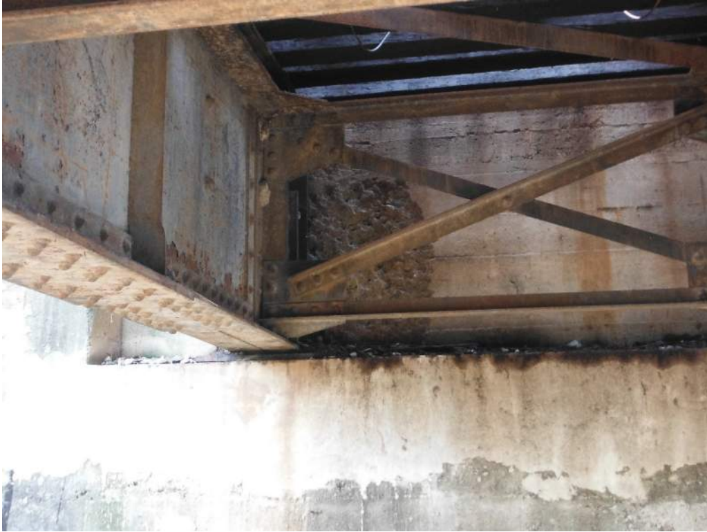
410.40 Backwall spall – Abutment 1
