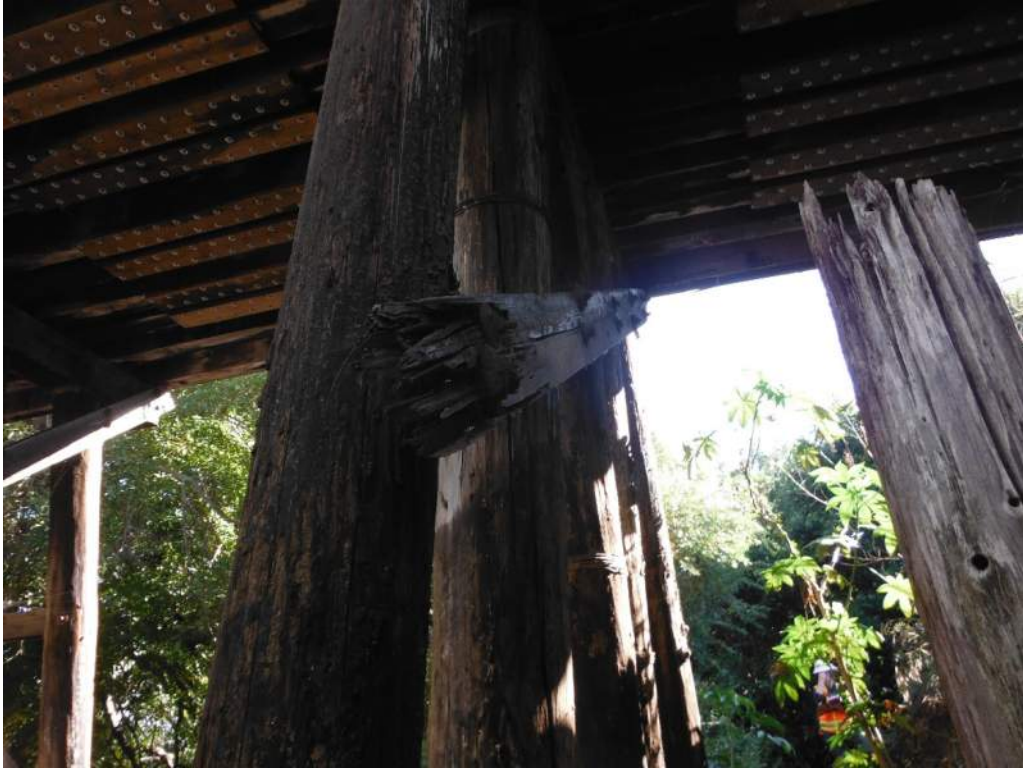
419.92 Sway bracing rotten - Bent 2
