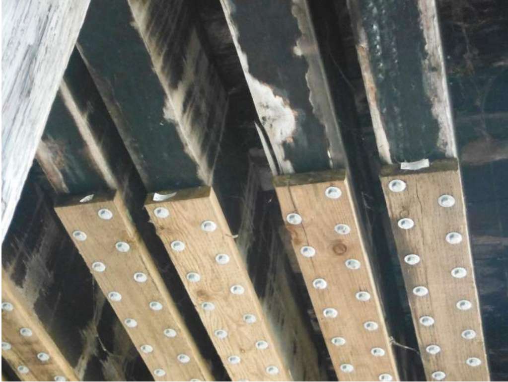
419.92 Stringer 4 split at ends of repair locations - Bent 4
