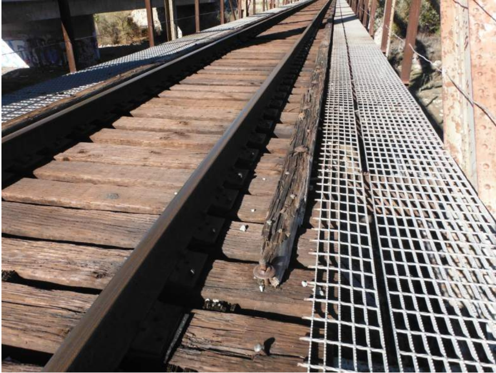
423.28 Damaged timber curb west and east side, typ
