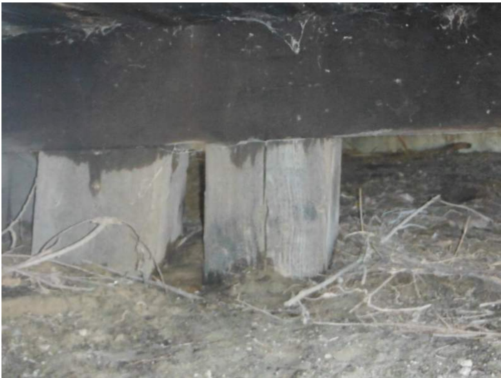
421.23 Pile #4 Splitting, Bent 2
