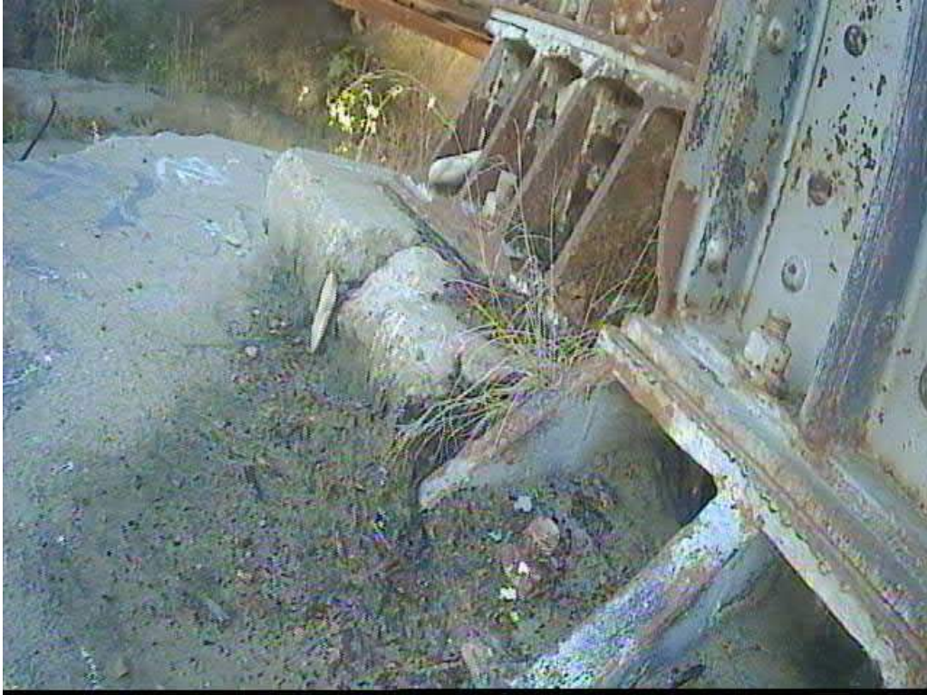
429.79 Spalling under bearing - Pier 2
