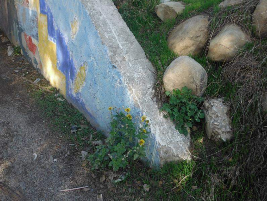
415.69 Spall on wingwall at abutment 4
