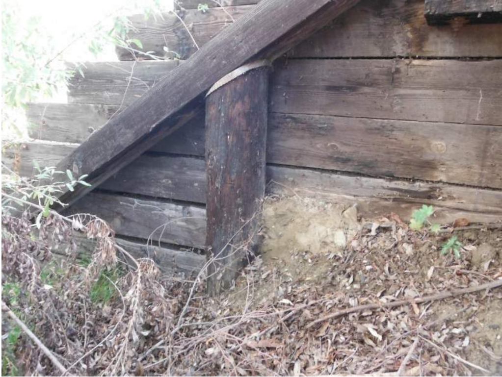
417.24 Abutment 6 backwall rotten at bottom
