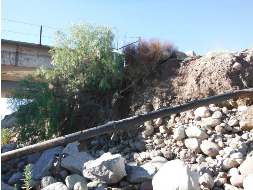
423.44 Deep erosion from heavy water on North slope
