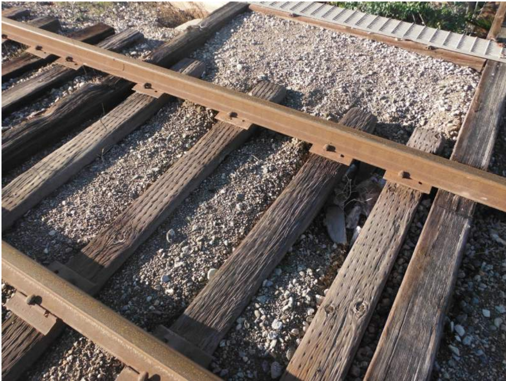
415.92 Ballast leak – Span 2 north side
