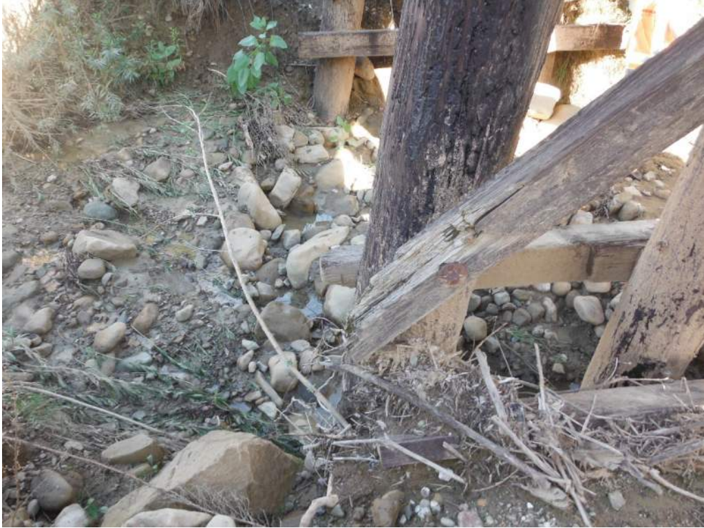
420.46 Span 2 & Bent 3, tier 1 sash brace is broken on left side
