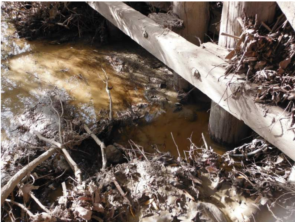
417.24 Scour hole between bent 3 & 4 – approximately 4'
