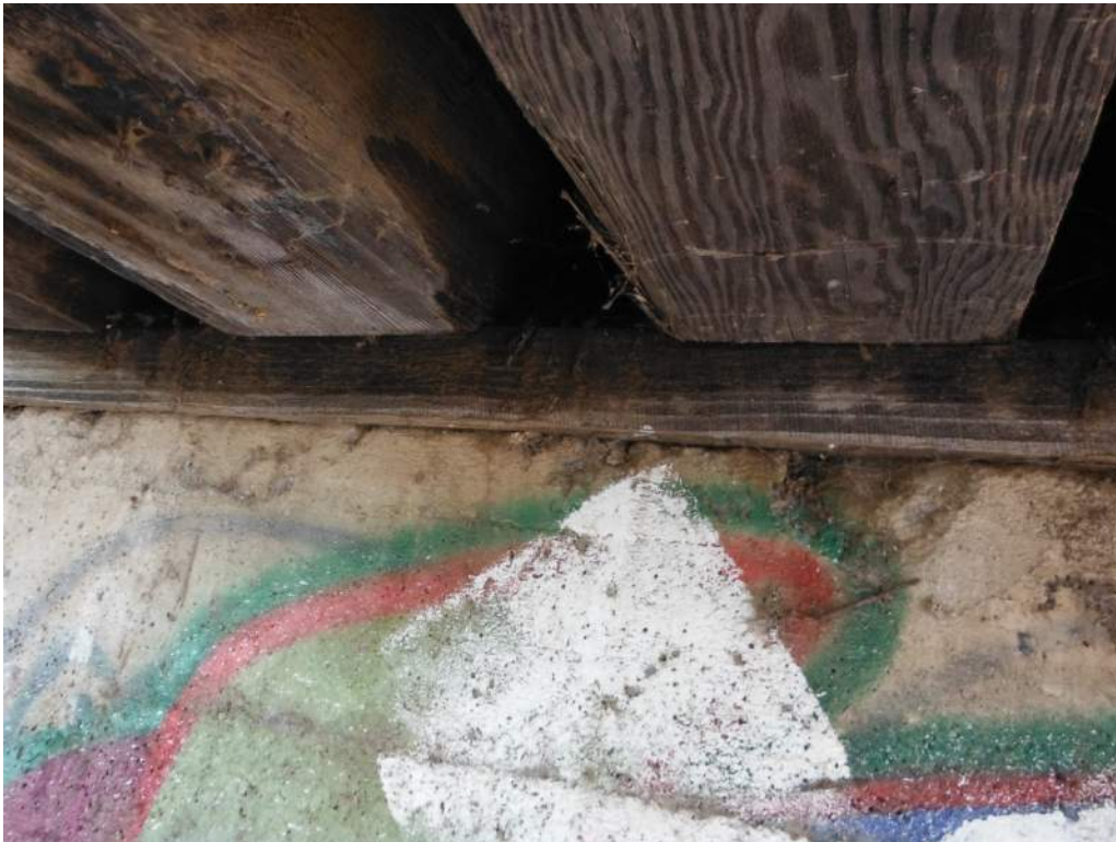
407.48 Stringers crushing \frac{1}{4} " at Abutment 3
