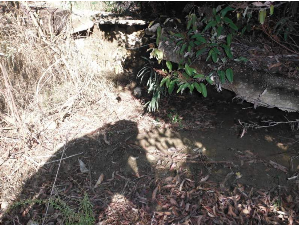
420.46 Slope paving undermining downstream of Bent 4
