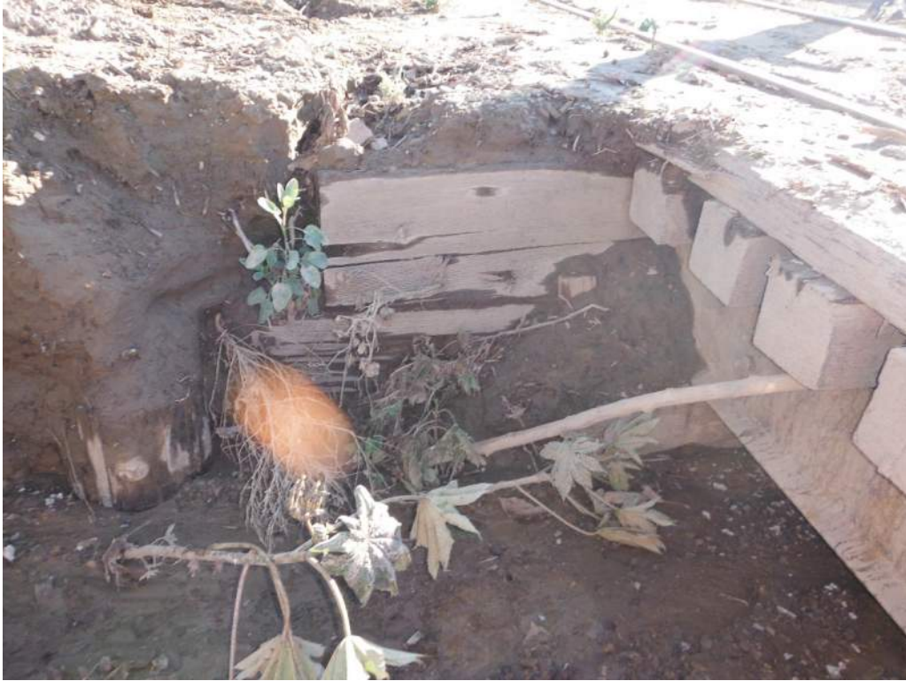
427.64 Backwall failing – Abutment 2
