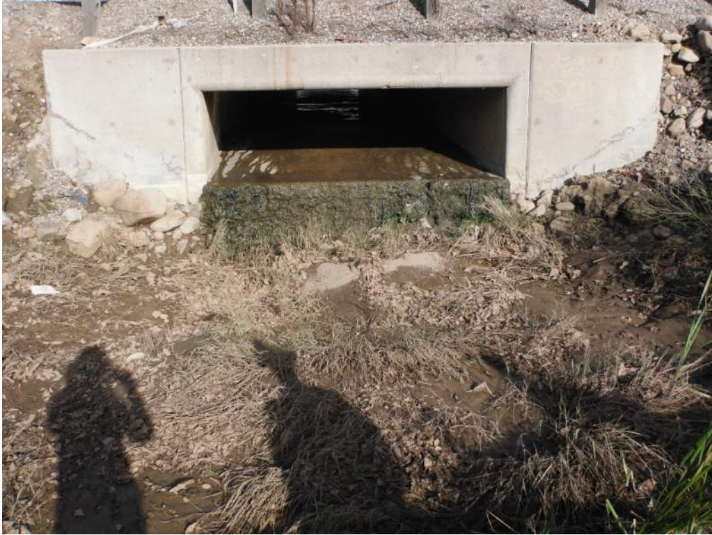
416.63 2' Scour at upstream culvert
