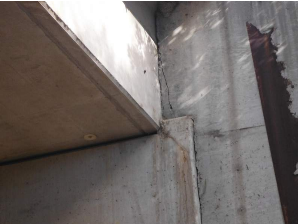
419.42 Crack in backwall, and crack and spall on south keeper – Abutment 2
