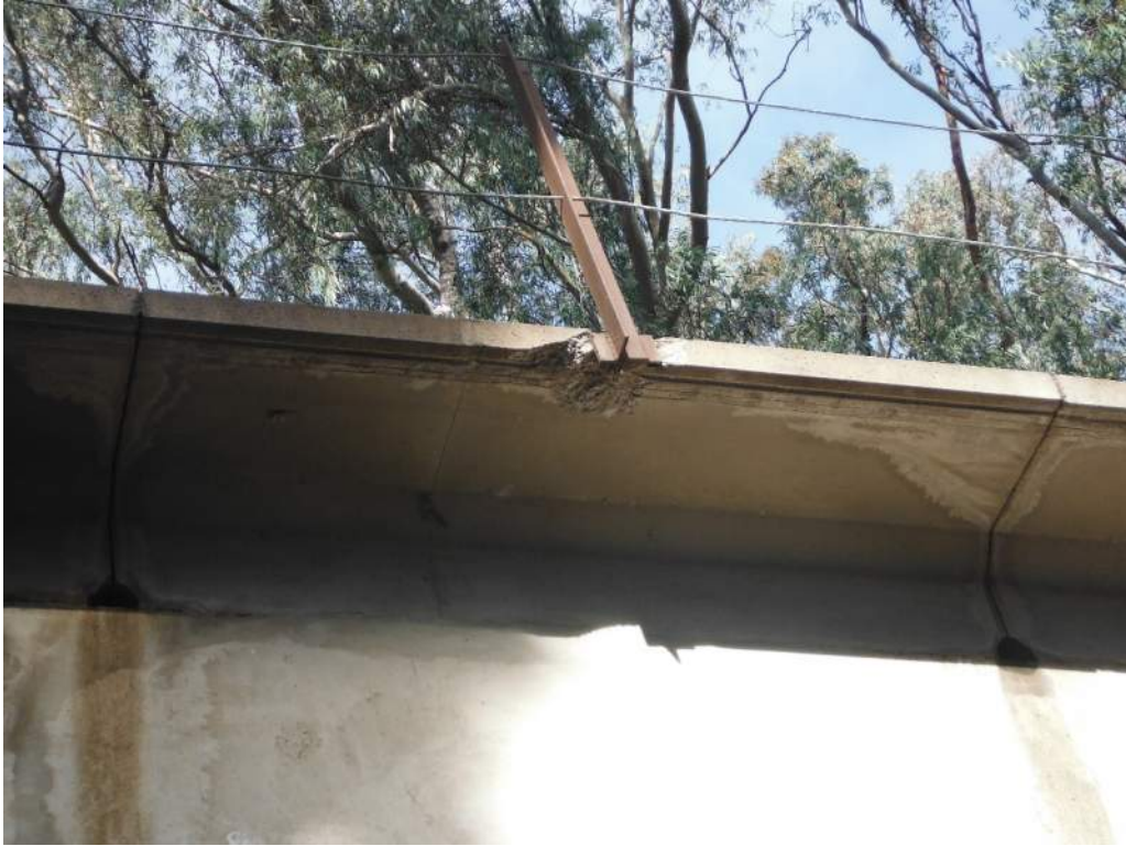
419.42 Spall on South walkway
