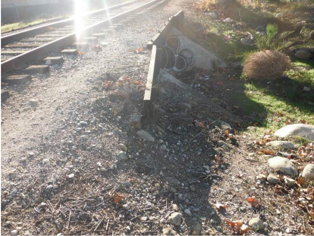
415.82 North ballast retainer leaning
