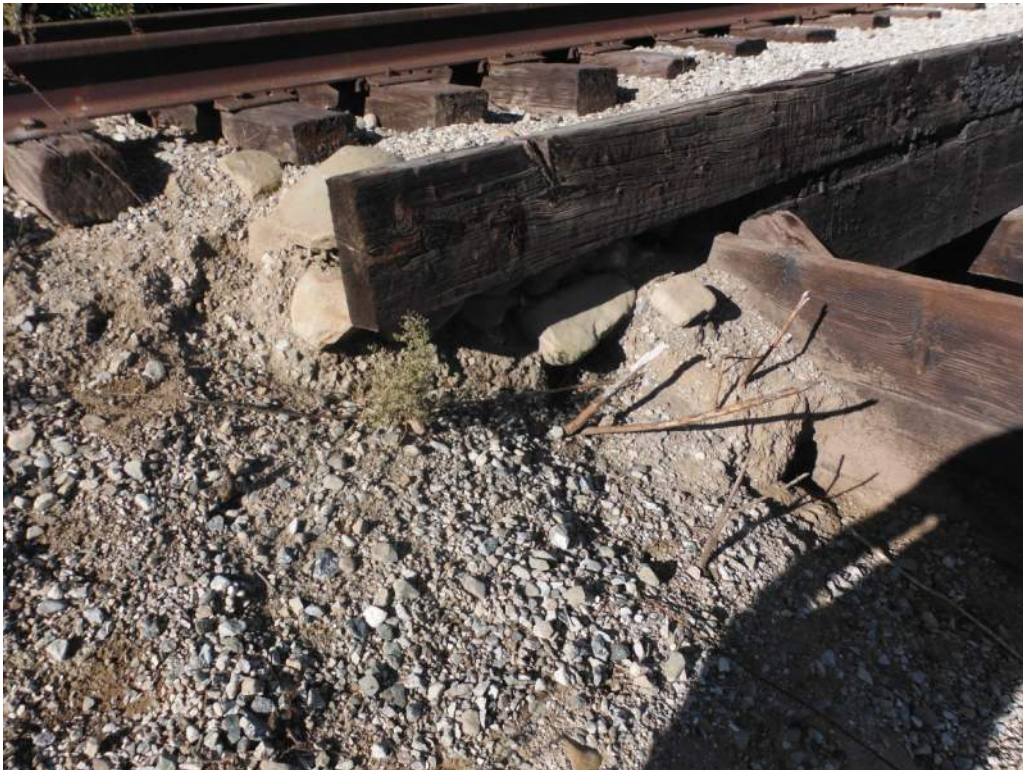
420.20 Undermining ballast retainer – north and south sides
