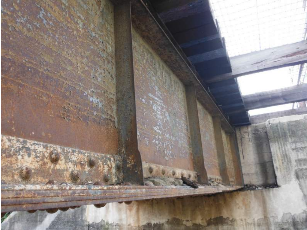
410.40 Deck girder is in fair condition with paint failure and surface rust
