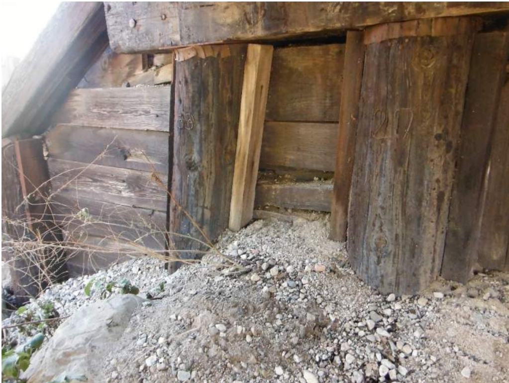
420.46 Abutment 1 backwall failed plank's supplement failed
