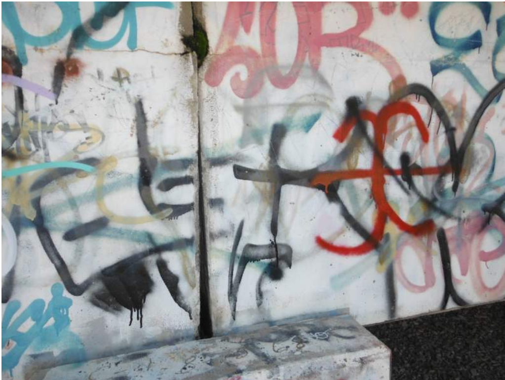
425.15 No gap between girders - Pier 2
