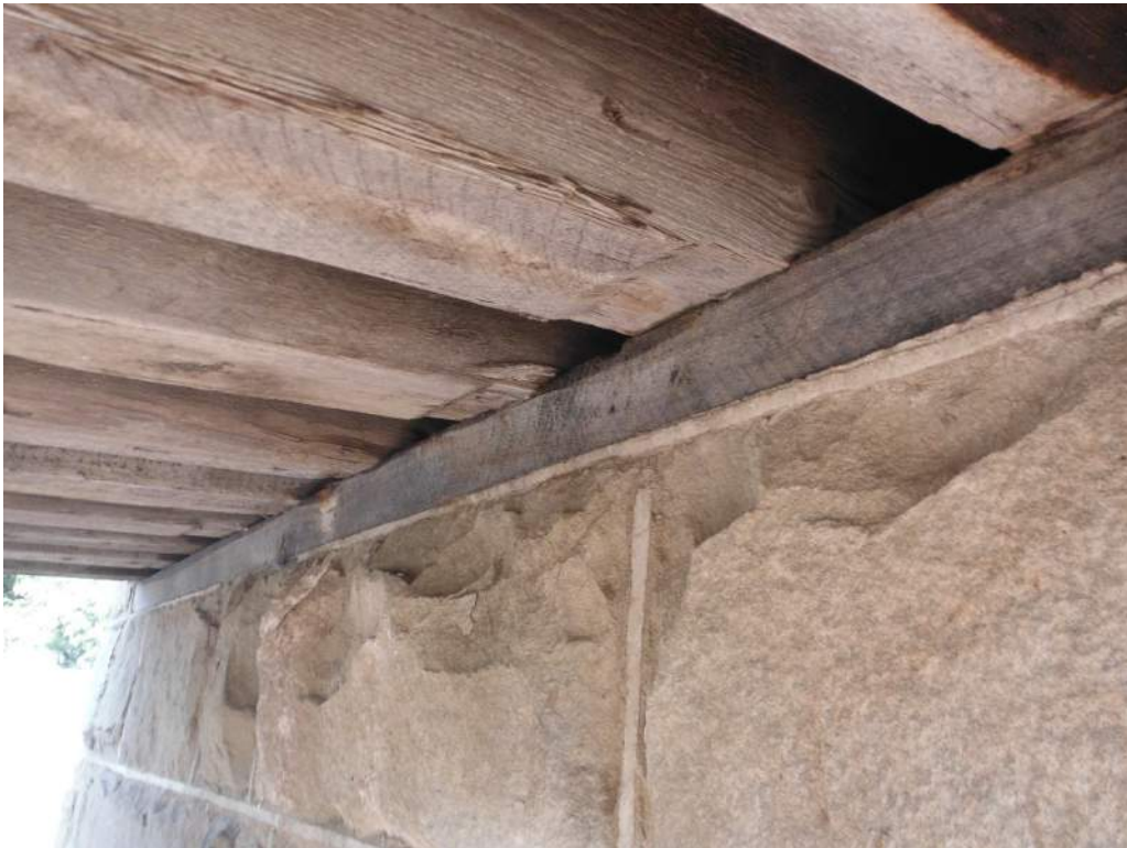
418.02 Stringers #5, 6, 7 crushing at Abutment 2
