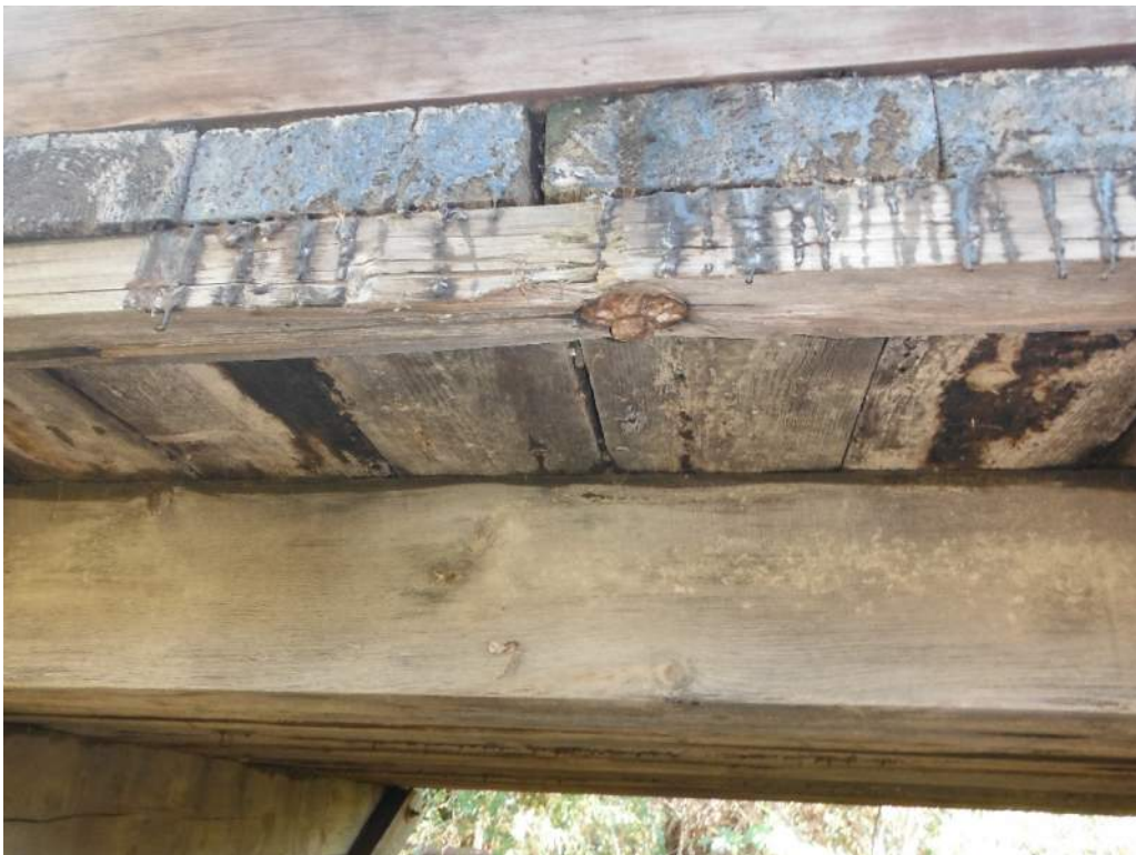
421.05 Deck sill splitting – Span 1
