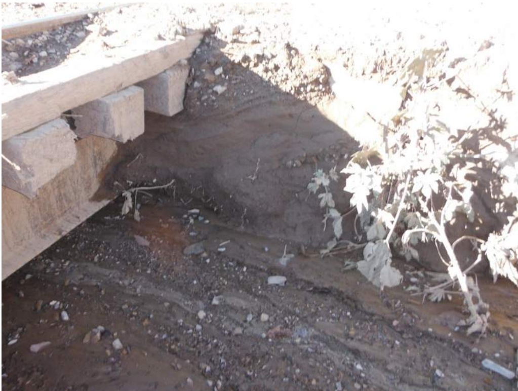
427.64 Backwall rotting – top timber of backwall failing, Abutment 1
