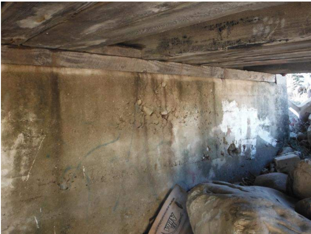
415.69 Abutment 1 Spall
