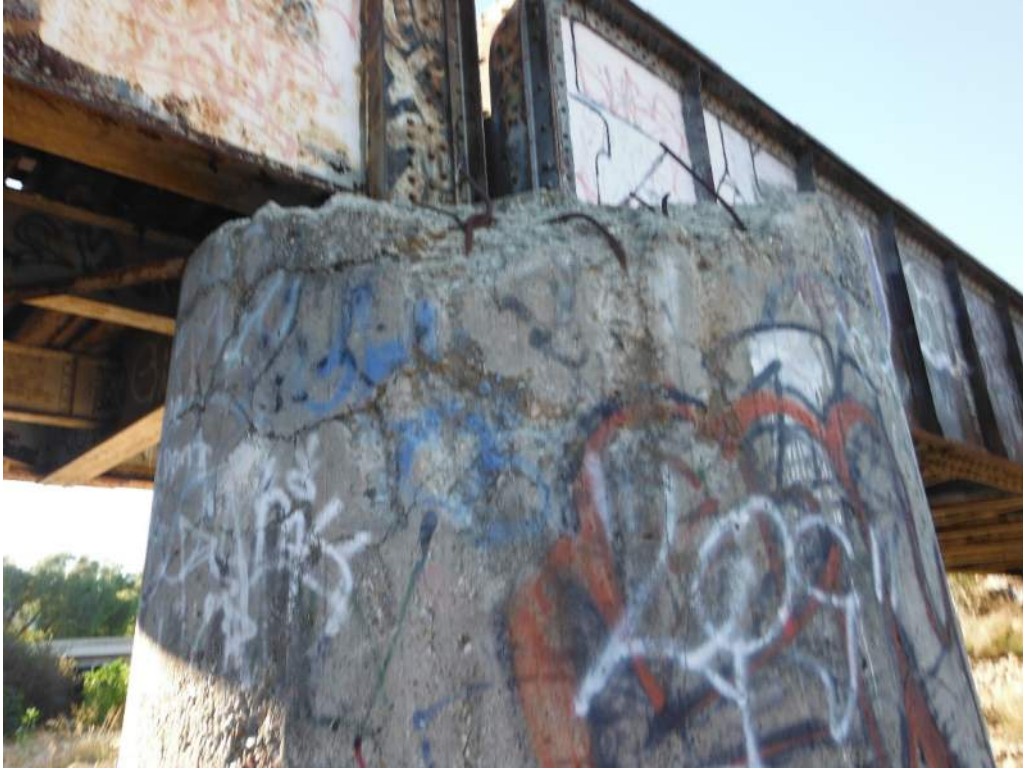
429.79 Exposed rebar - Pier 2 north side
