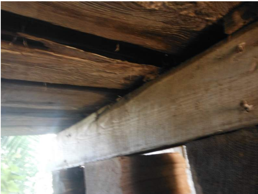
415.92 Stringer 5 rotten, Stringer 2 & 4 failed, Span 2
