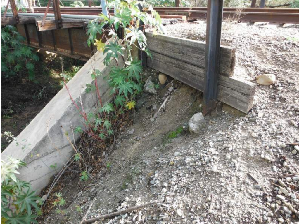
410.40 NW ballast retainer undermining
