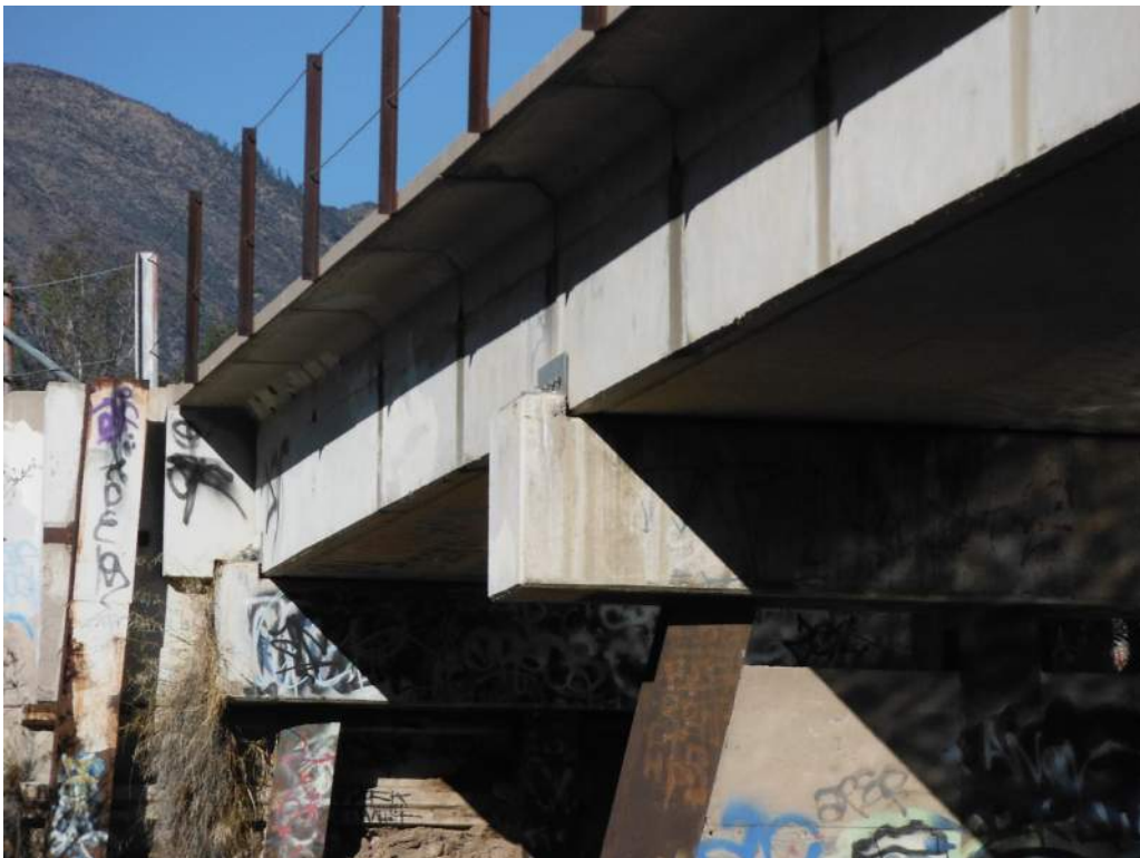
423.44 Keeper spall on Pier 2
