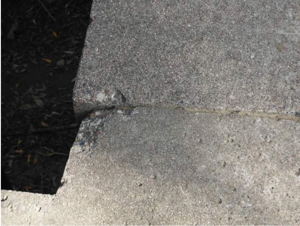
411.97 Spall on NW Corner of Walkway
