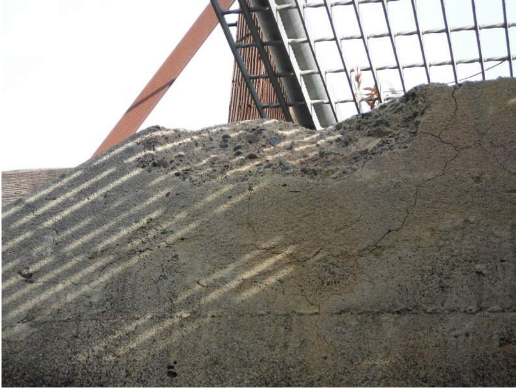
410.40 NE Wingwall spall – Abutment 2
