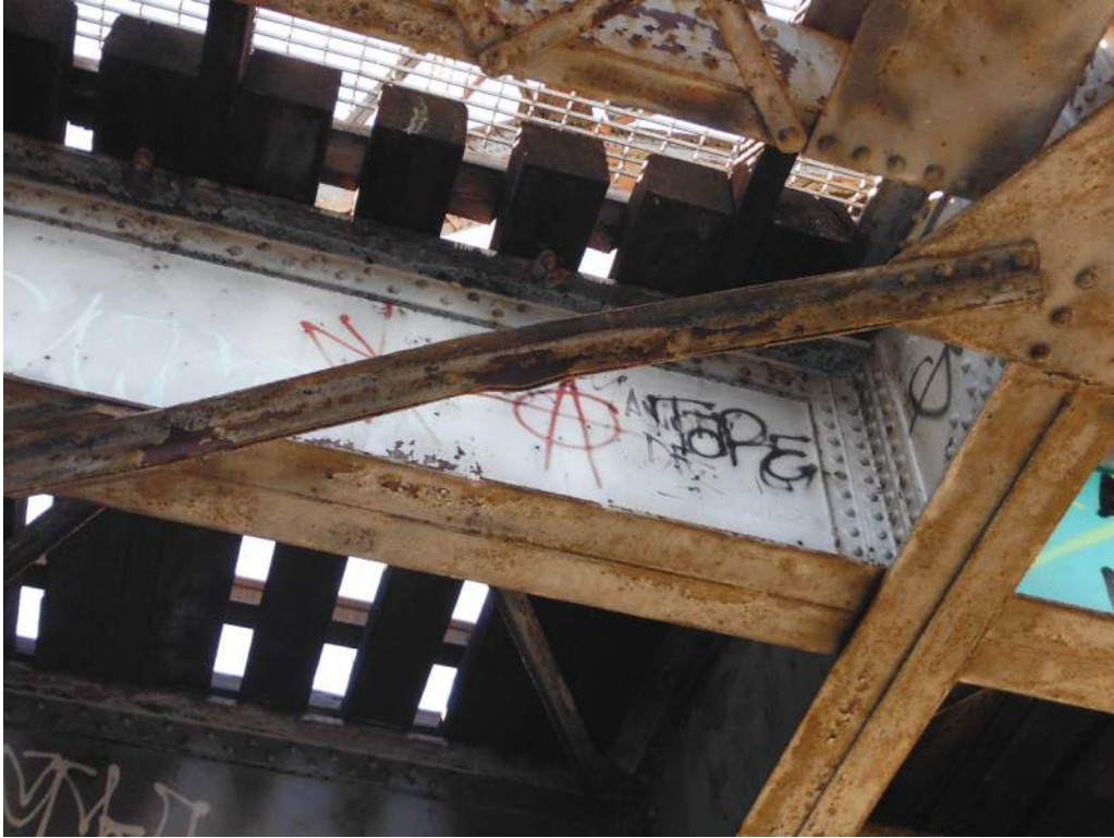
423.28 Minor impact damage to cross bracing near Abutment 2
