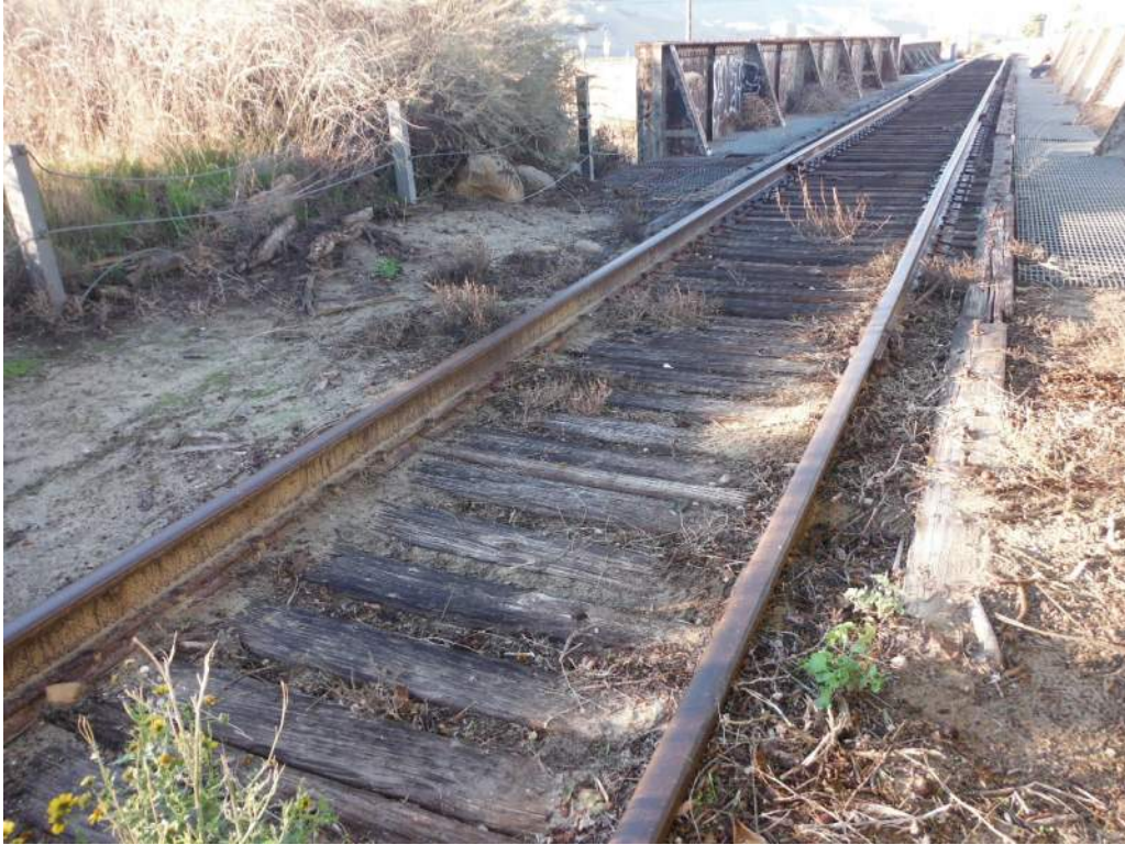
429.79 Timber approach spans fully silted in
