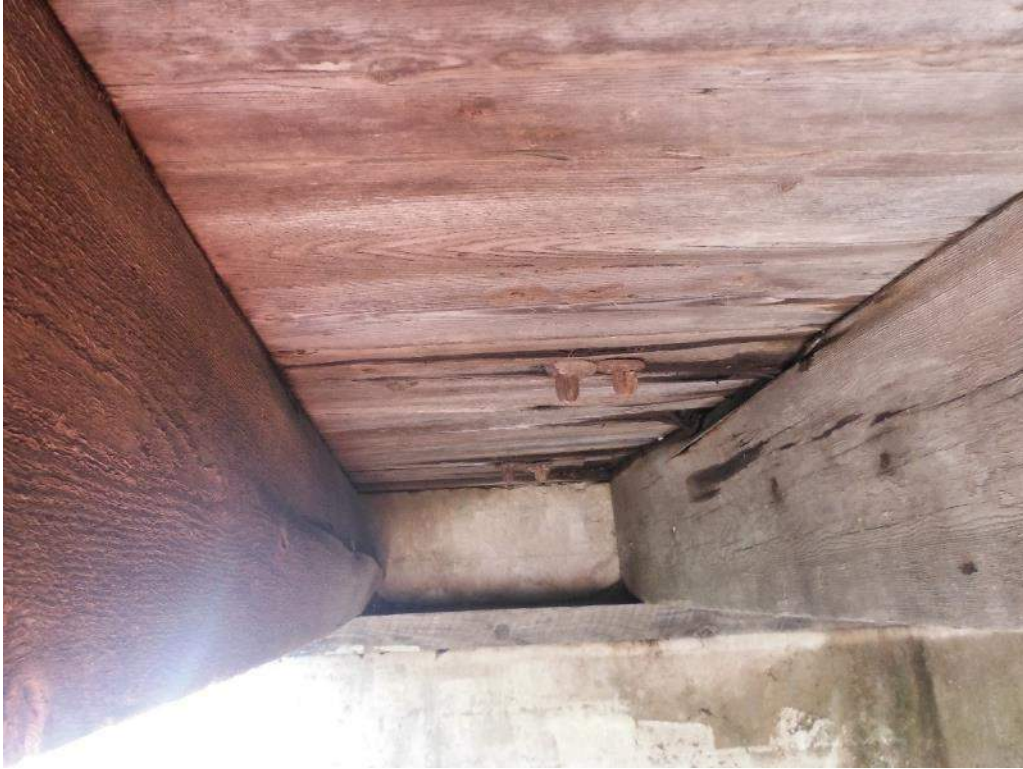
415.69 Rotten deck plank at Abutment 1
