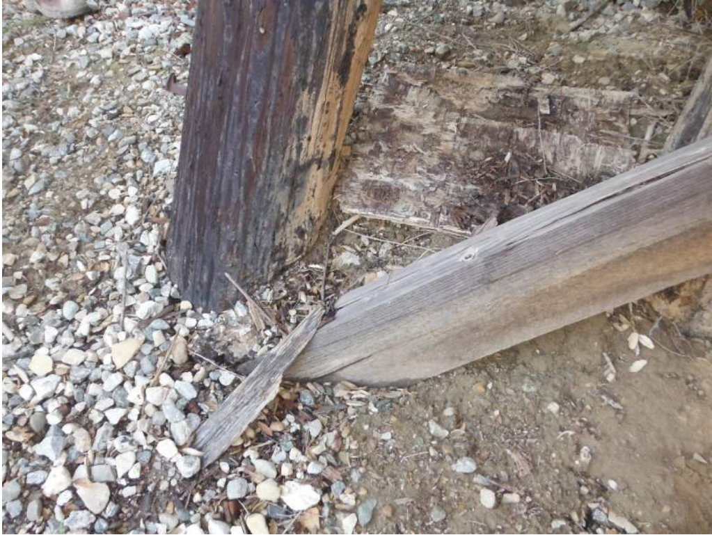
420.46 Cross bracing rotten, Bent 6
