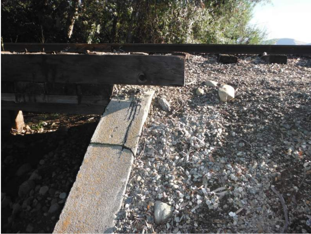
421.05 Ballast Curb Undermined all 4 Corners
