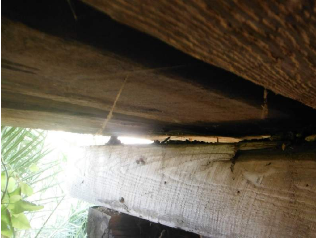
415.92 Helper bents not shimmed to stringers – both spans
