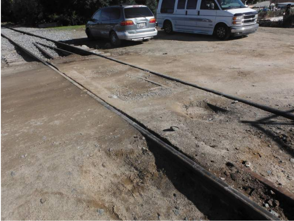
415.59 Material between inside guardrail and running rail, typ both sides
