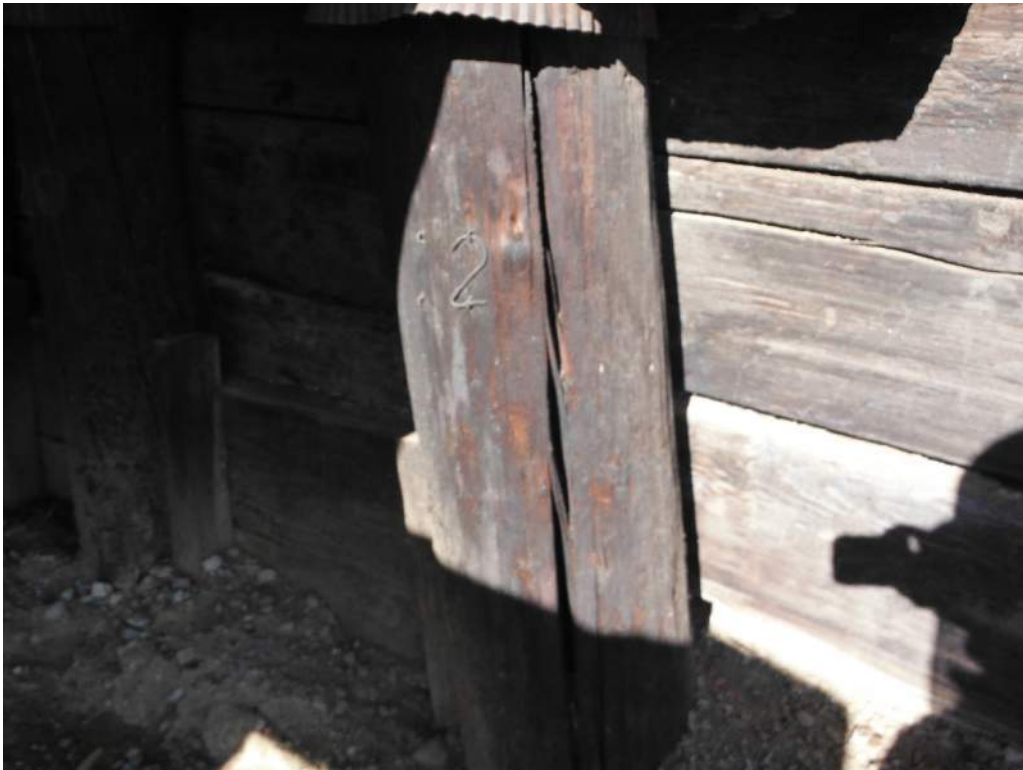
420.20 Abutment 5 Pile 5 split
