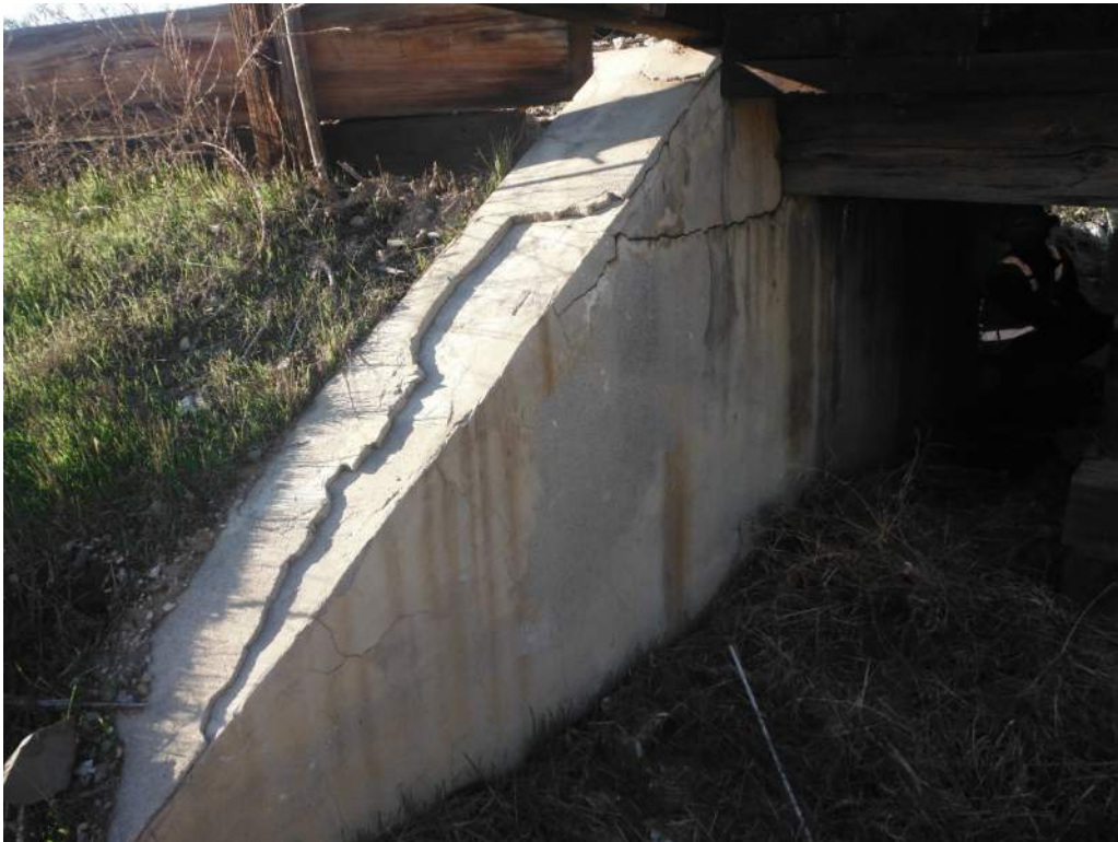
415.92 Abutment stringer retainer cracked- typical NW, SW, SE
