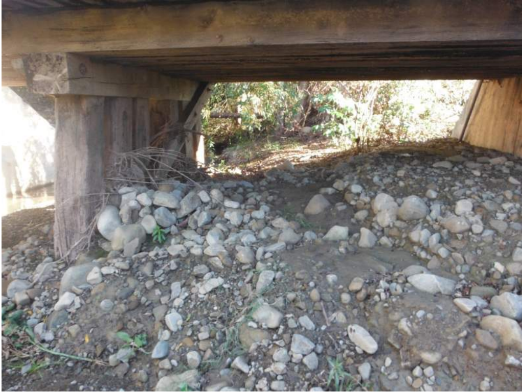
421.05 Span 1 silting in
