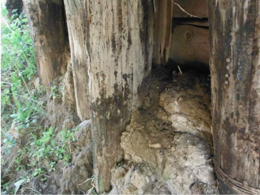
419.92 Abutment 1 back wall scour
