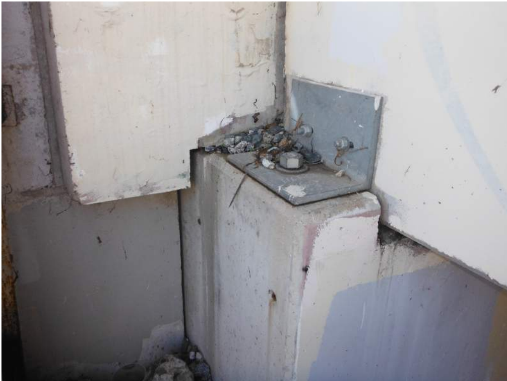
423.44 Ballast leaking on bearing seats, near Abutment 16
