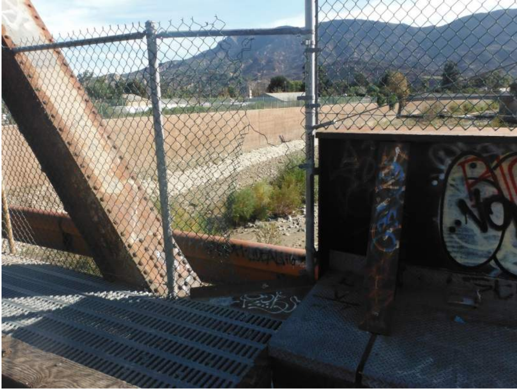
415.59 Fence breach over Pier 2, south side
