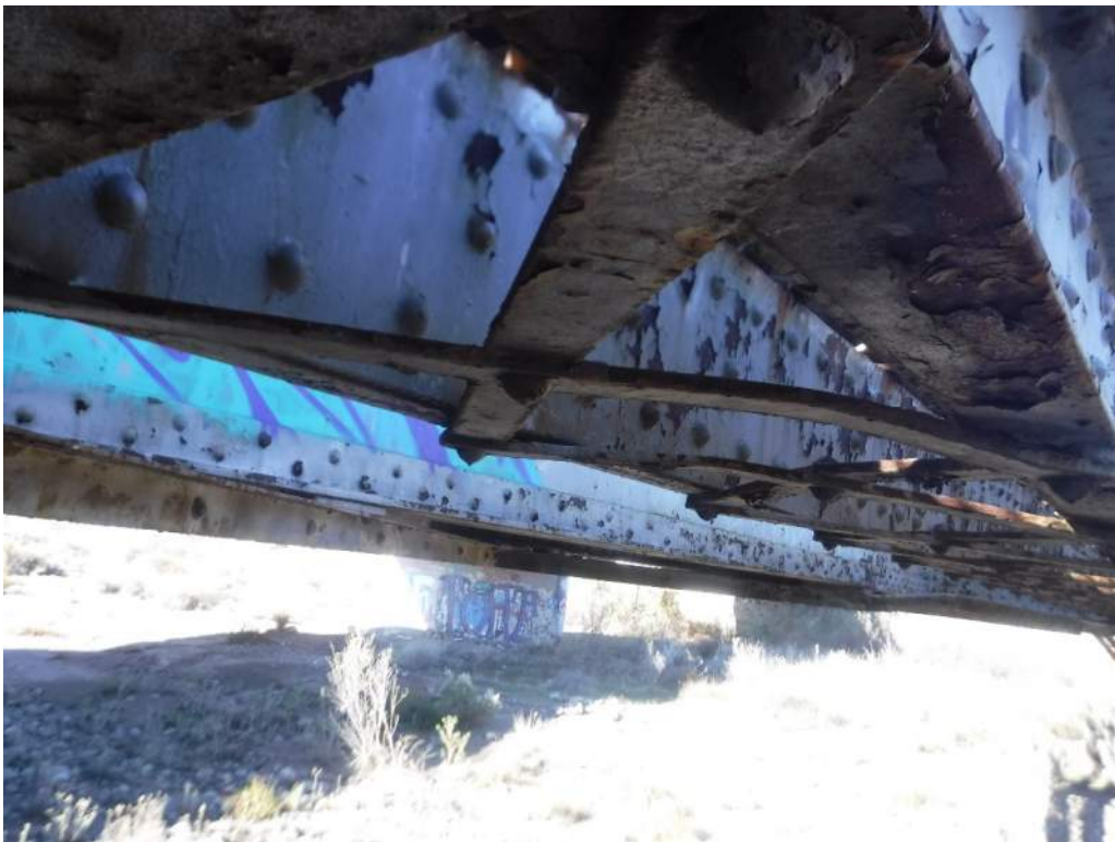
423.28 Impact damage to bottom chord lattice bracing at bay 7
