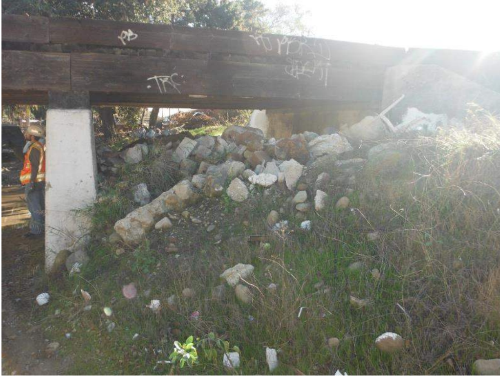
415.69 Debris under Span 1
