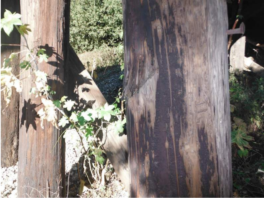
420.46 Impact damage pile 5, Bent 5
