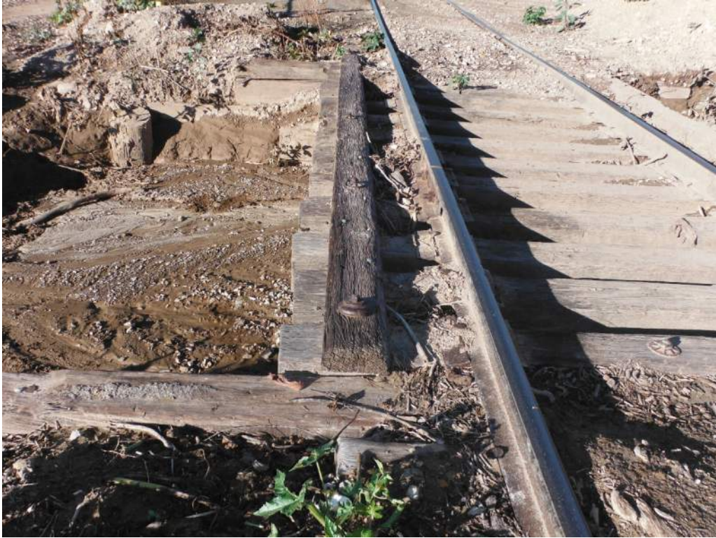
427.64 Hole in ballast behind Abutment 2
