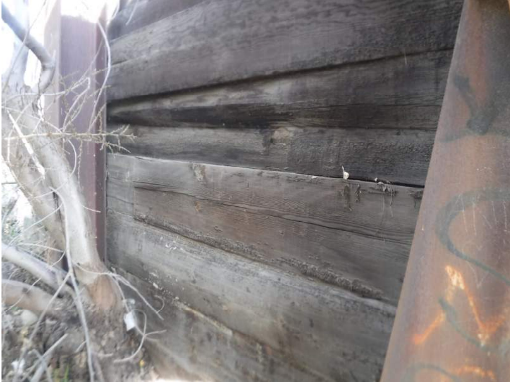
408.84 Abutment 6 backwall rotten
