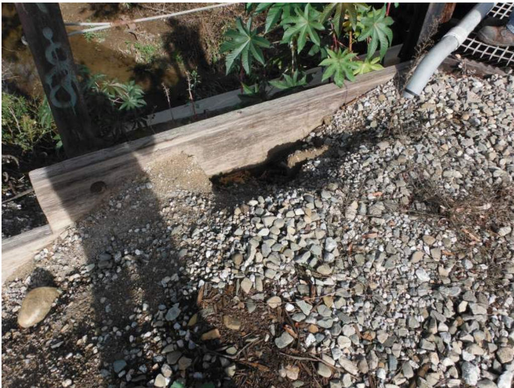
410.40 NW Hole in Ballast due to Undermining
