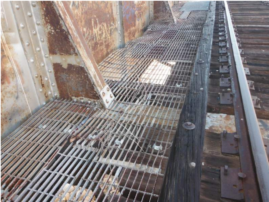
429.79 South walkway damaged near Pier 2
