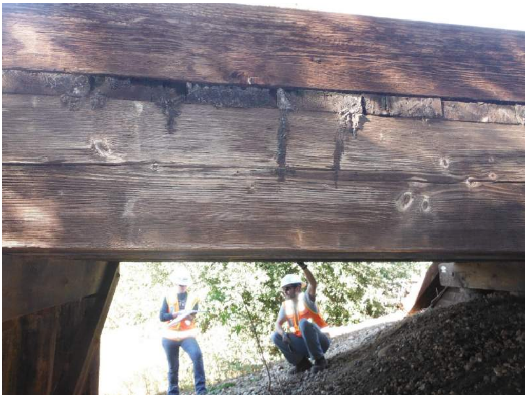
420.46 Spans 5 and 6, south exterior stringer has deep checking
