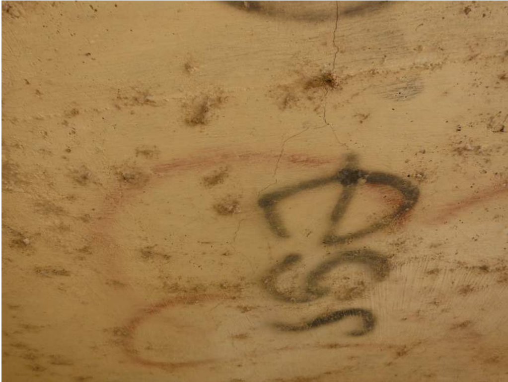
408.02 Hairline cracking underside of top slab, south side
