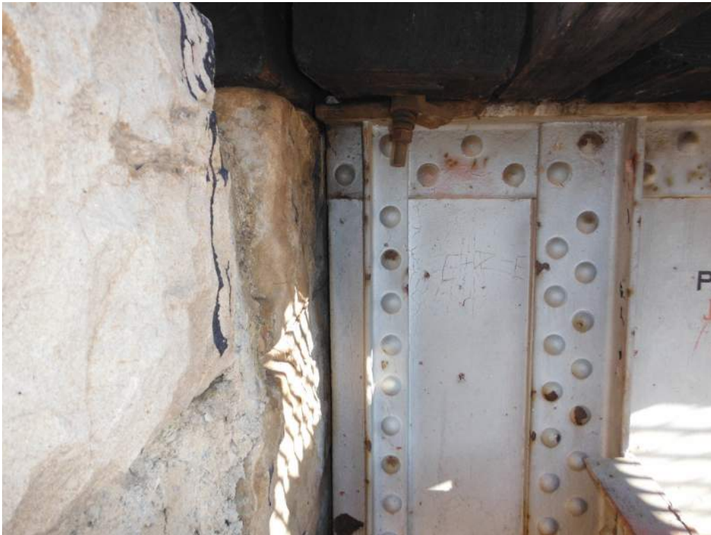
423.28 No gap between end of stringer and backwall – Abutment 1
