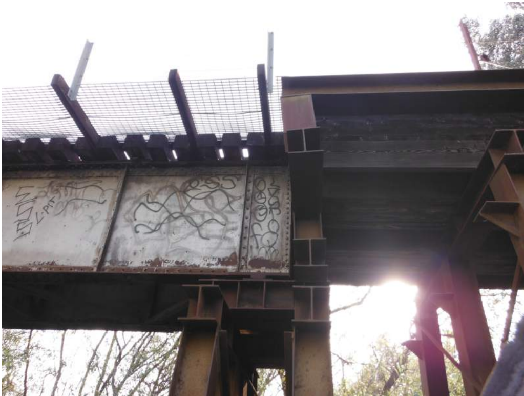
408.84 Pier 2 & 4 built up section rotated
