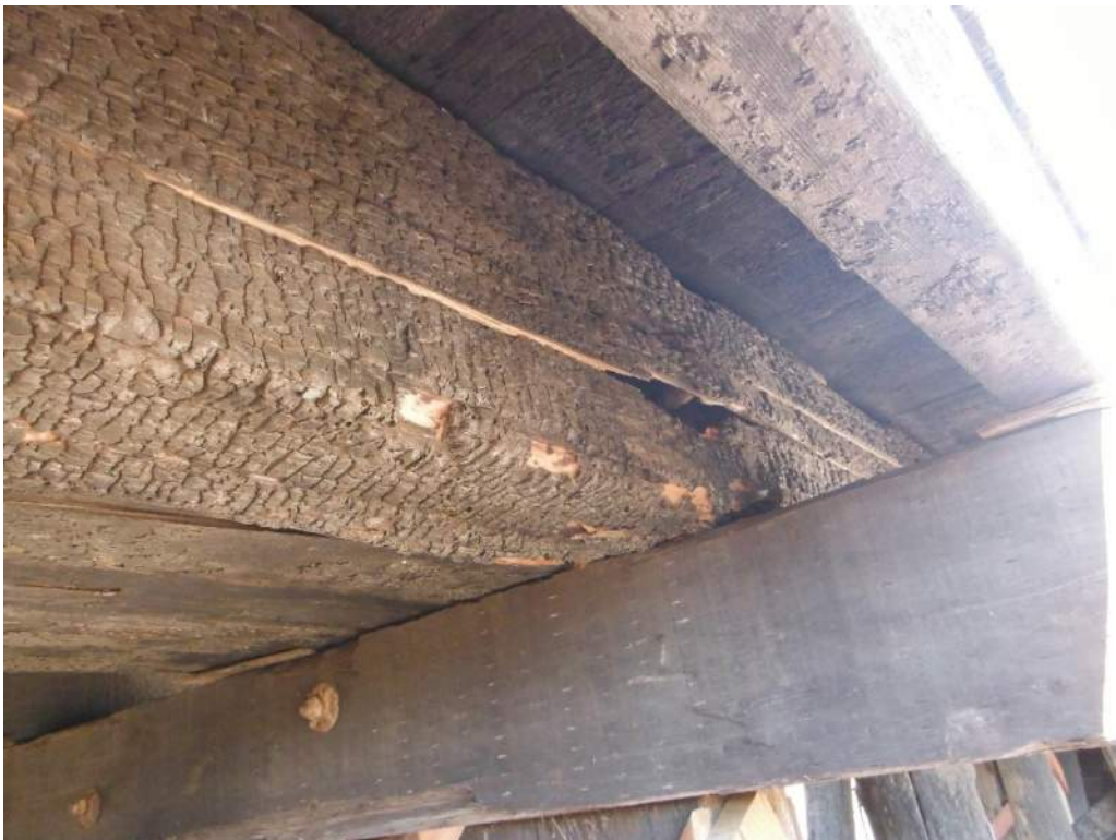
420.20 Span 2, Stringer 9 failed at helper bent
