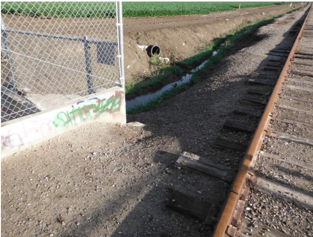
408.02 Erosion at Northeast embankment
