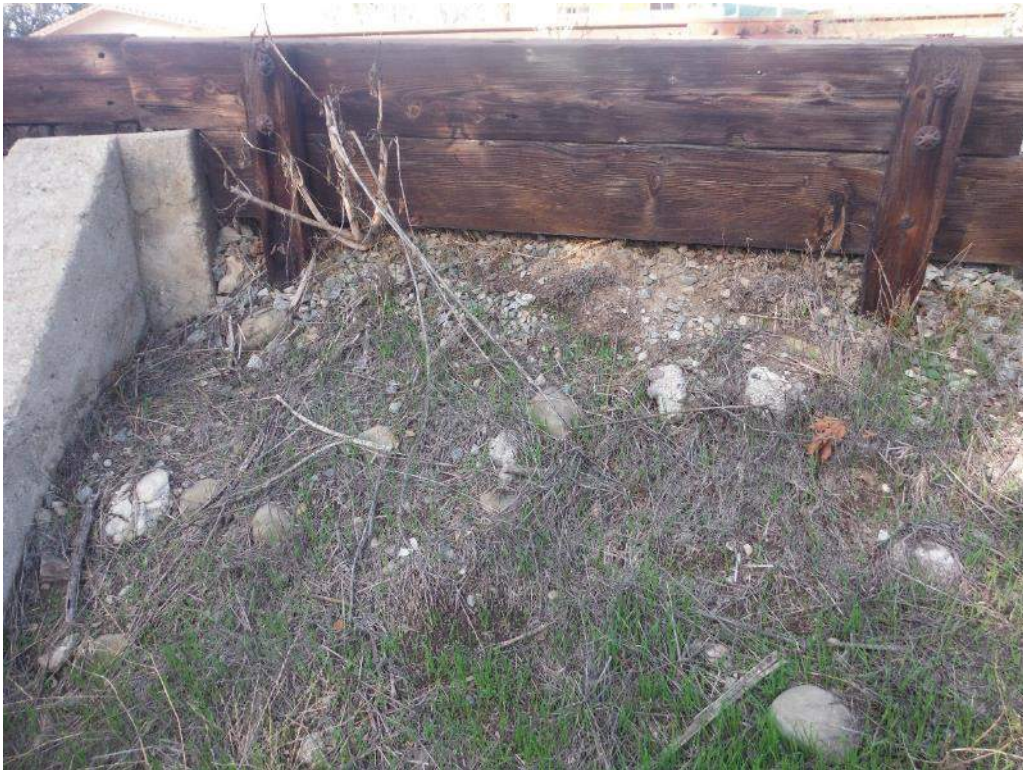
415.69 Undermining SE ballast retainer
