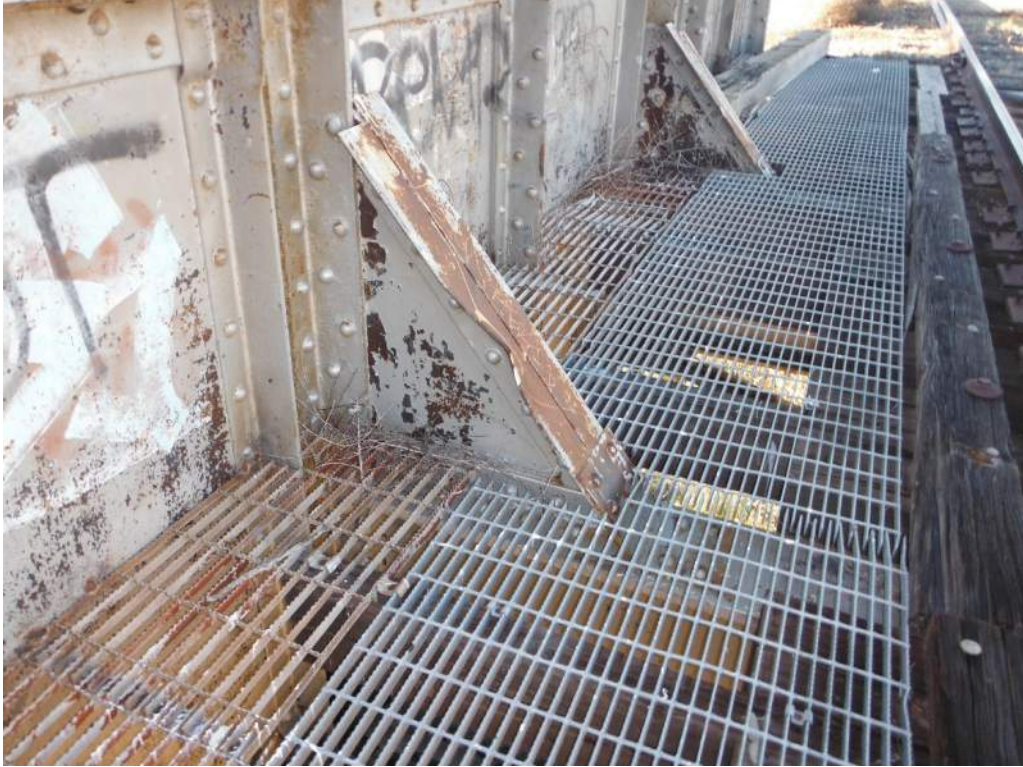
429.79 Minor impact damage on knee braces
