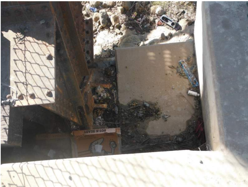
415.59 Debris at NE Bearing
