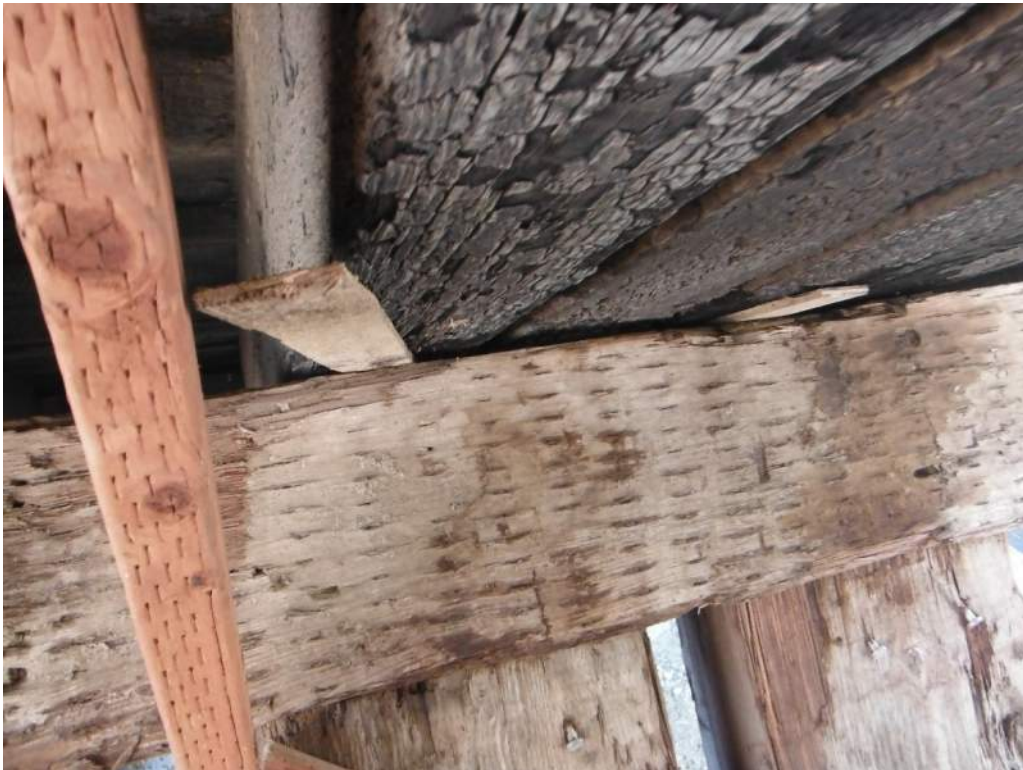
420.20 Gap between stringer and helper bent, typ.
