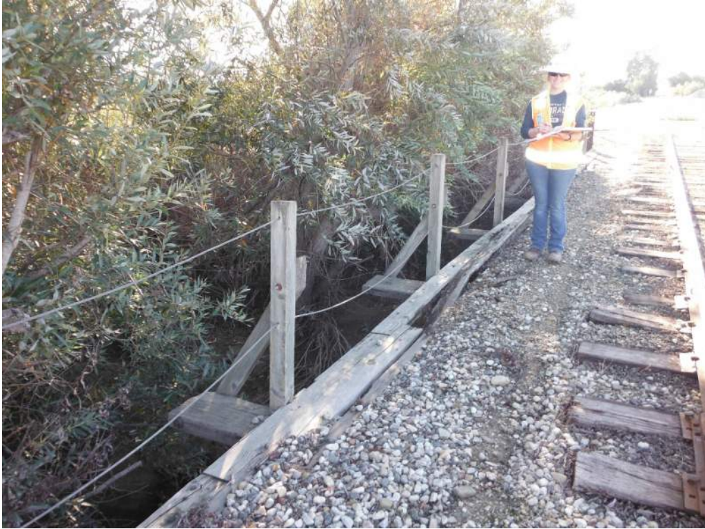
421.23 Loose Handrail Cable Both Sides
