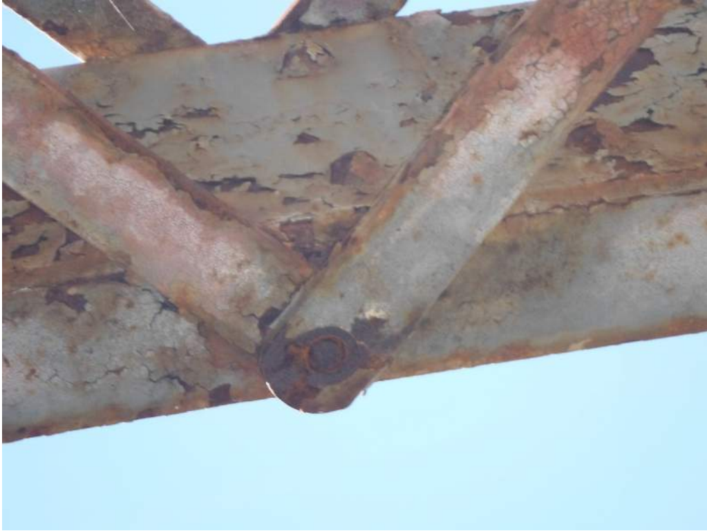
423.28 Missing rivet near Bay 2 bottom chord
