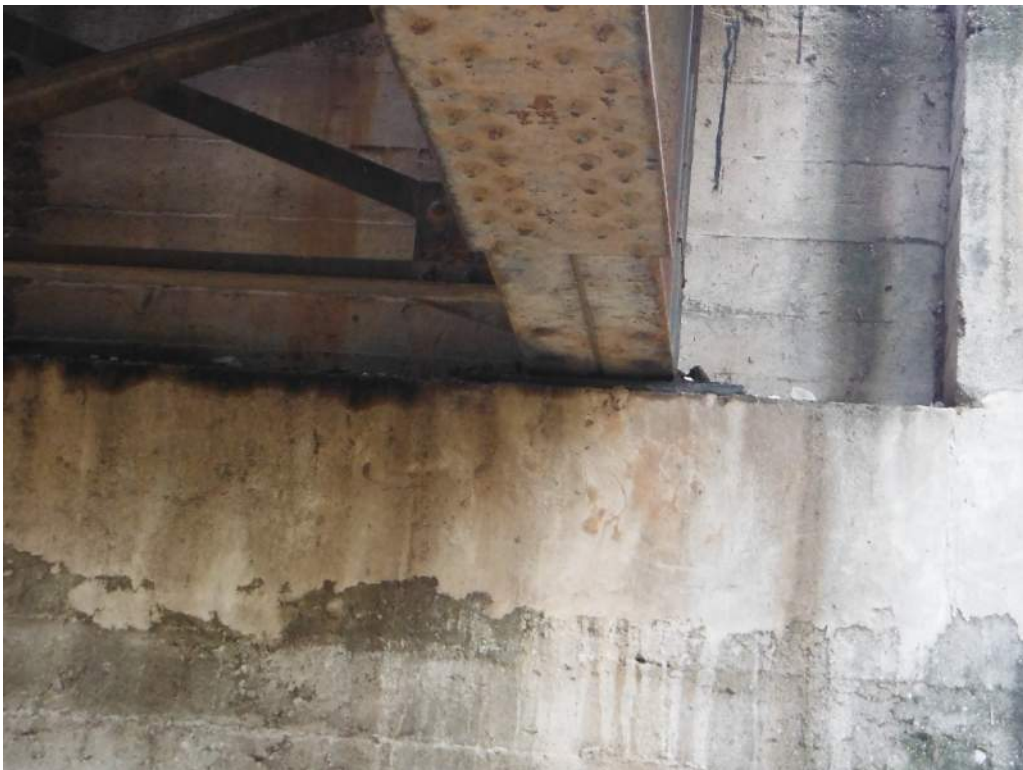
410.40 Open Flange Holes near Bearing, Abutment 1
