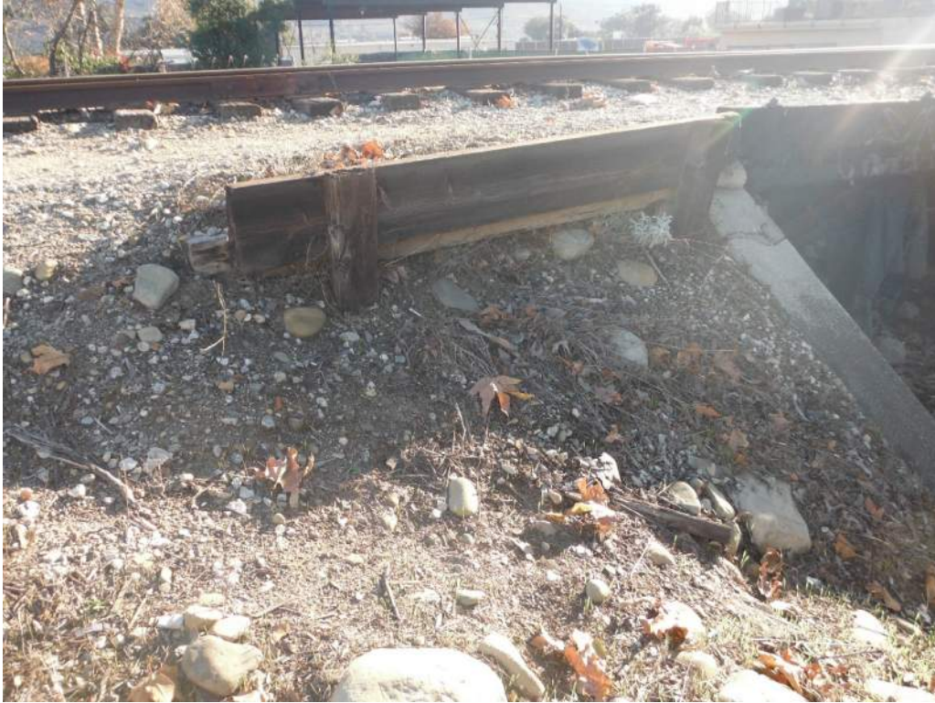
415.82 Wingwalls undermined – typical all 4 corners
