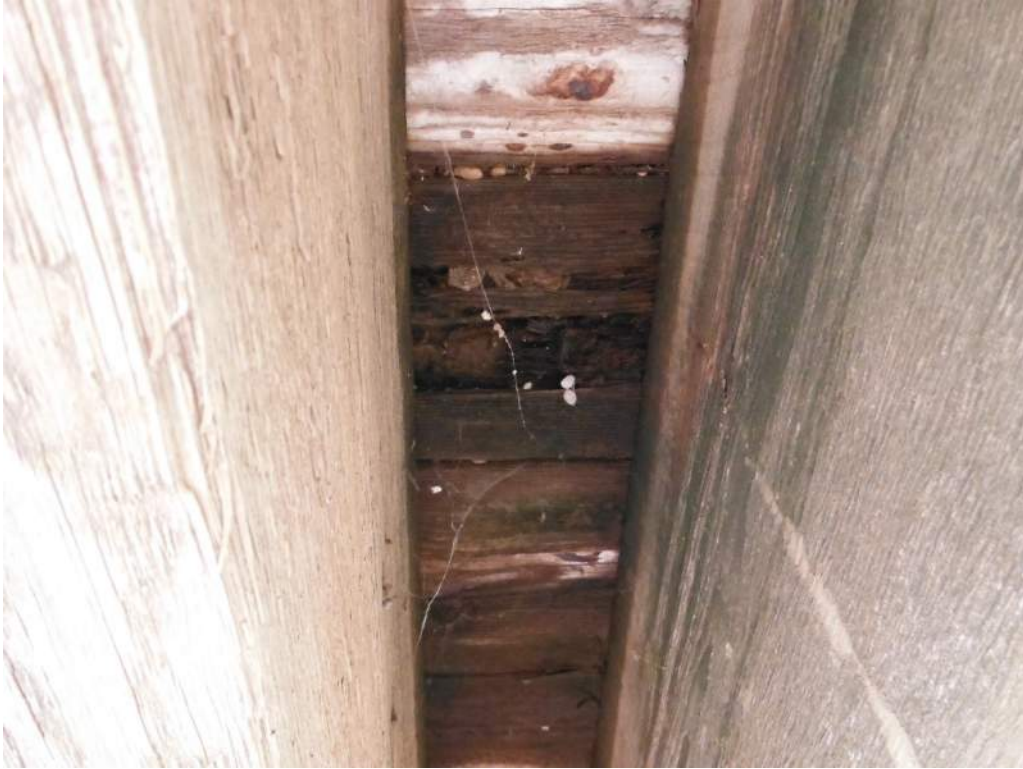
418.02 Deck planks showing signs of rot and multiple holes
