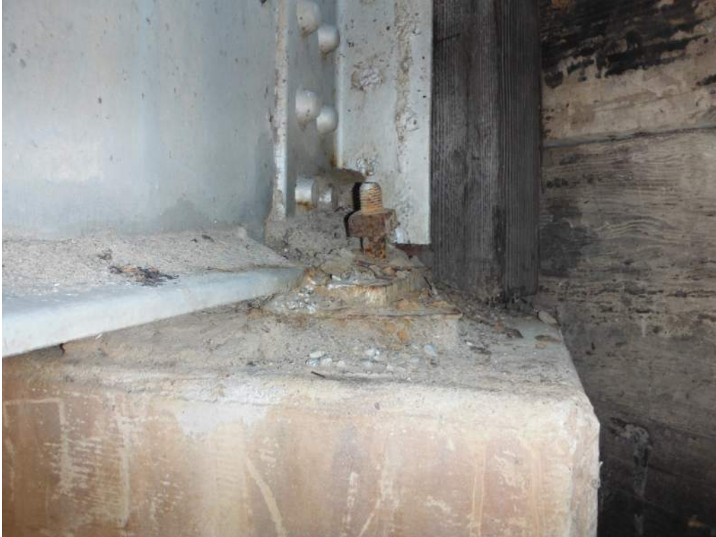
429.79 Loose anchor bolt – Stringer 1 & 2, Abutment 1
