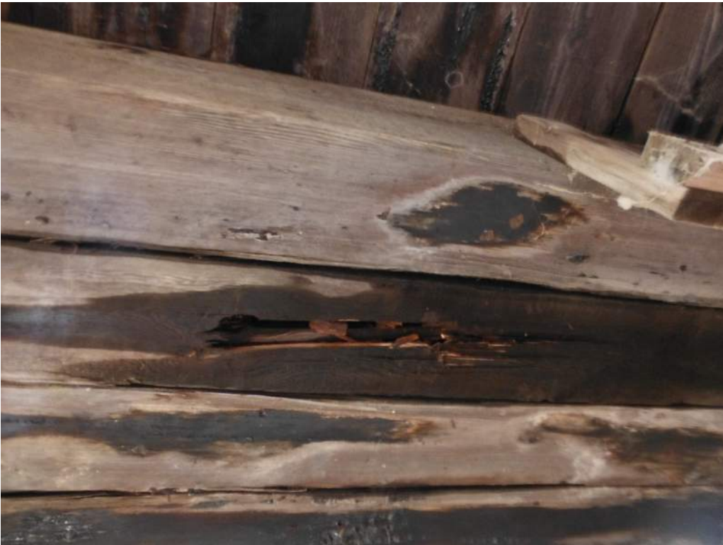
417.24 Stringer 3 failed, Span 1
