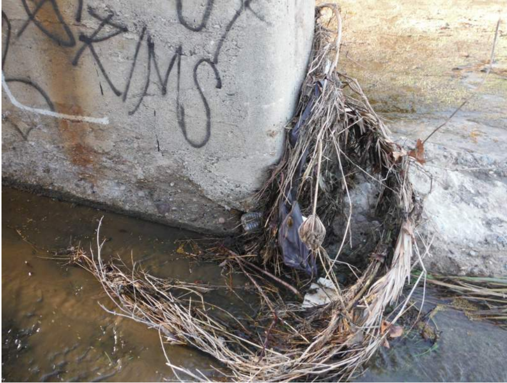
407.48 Spall and debris on upstream side of Pier
