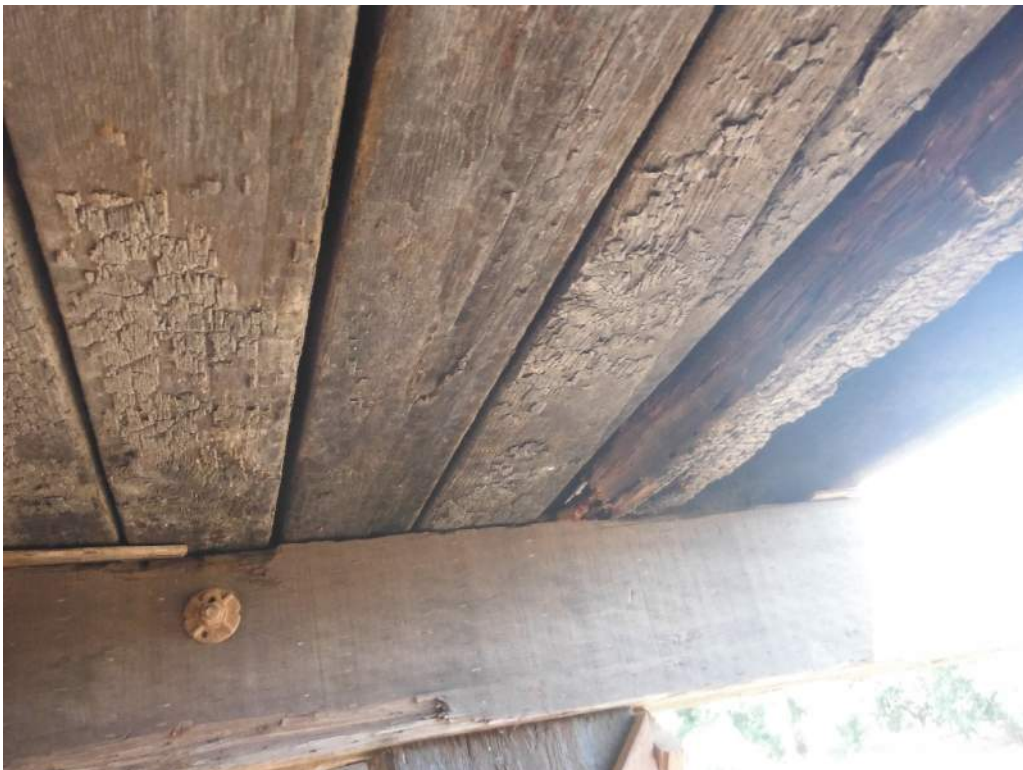
420.20 Stringer 8 shear split and Stringer 9 failed Span 2
