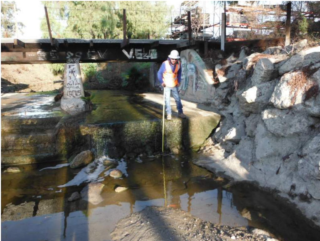
407.48 Scour at Downstream End of Channel Paving – approximately 3'
