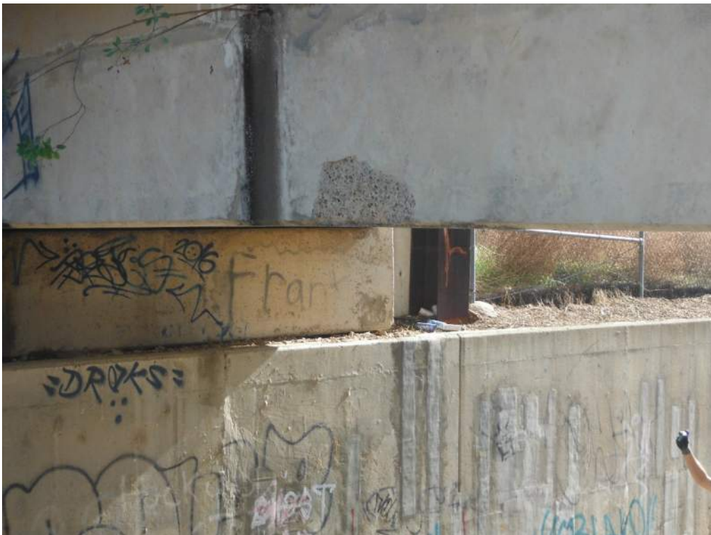
425.15 Spall at midspan - Span 2 north side
