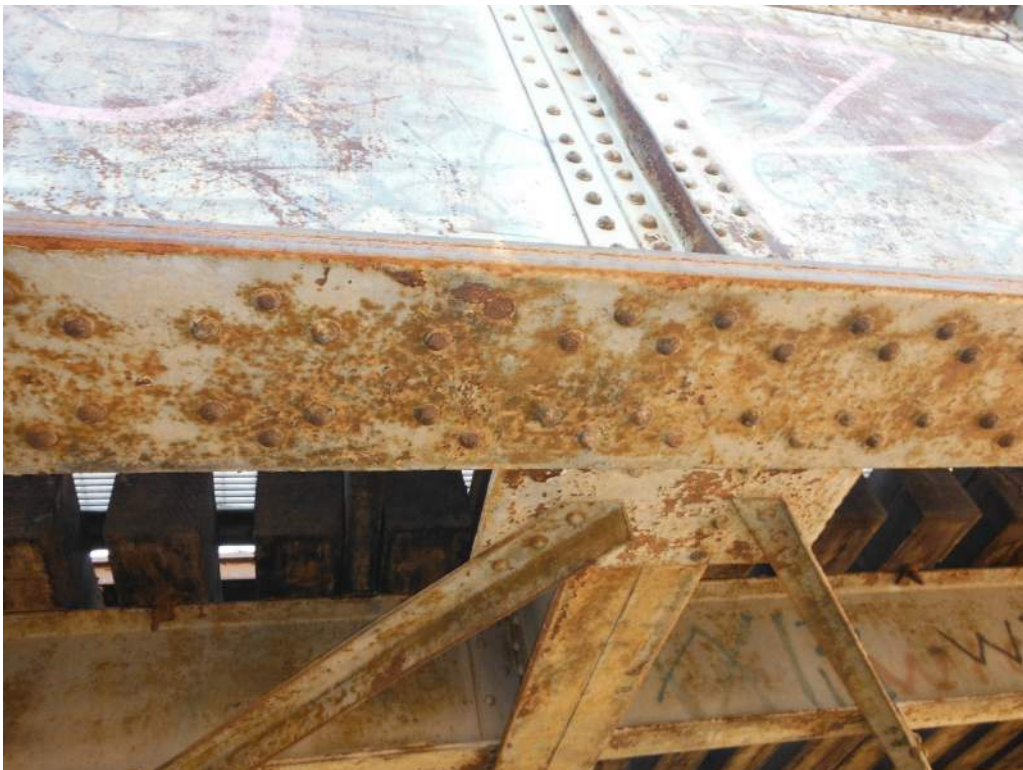
429.79 Sheared rivet GI mid span, Span 2 at floor beam 3
