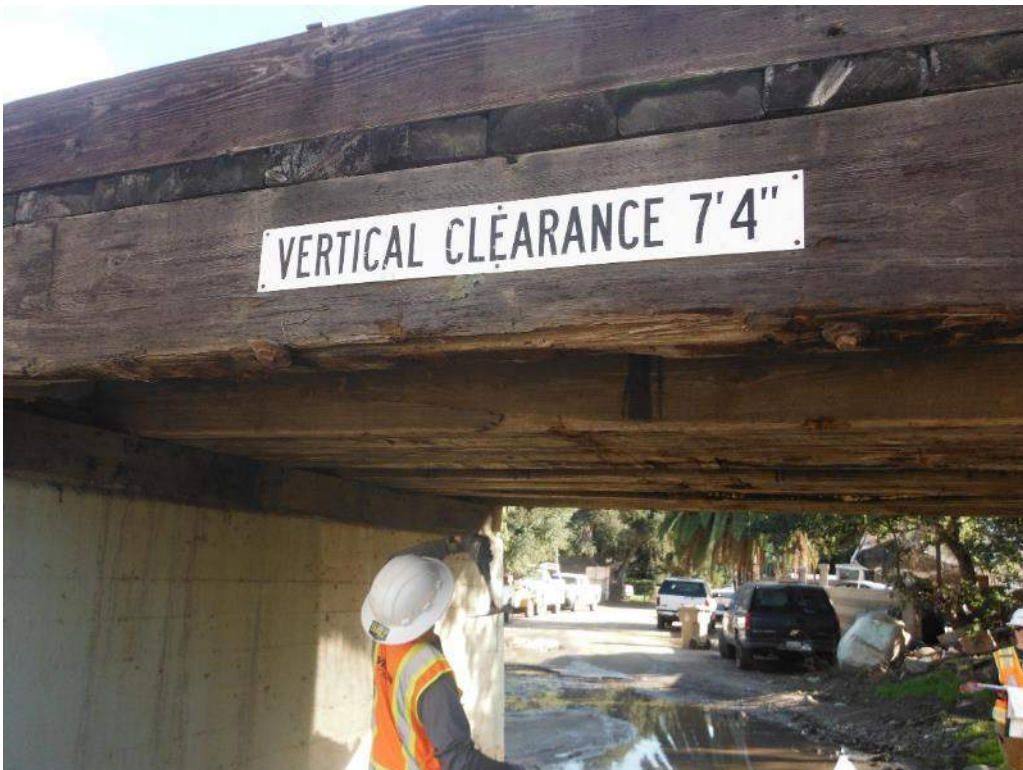
415.69 Major impact damage to Stringer 1, typ Span 2 and 3
