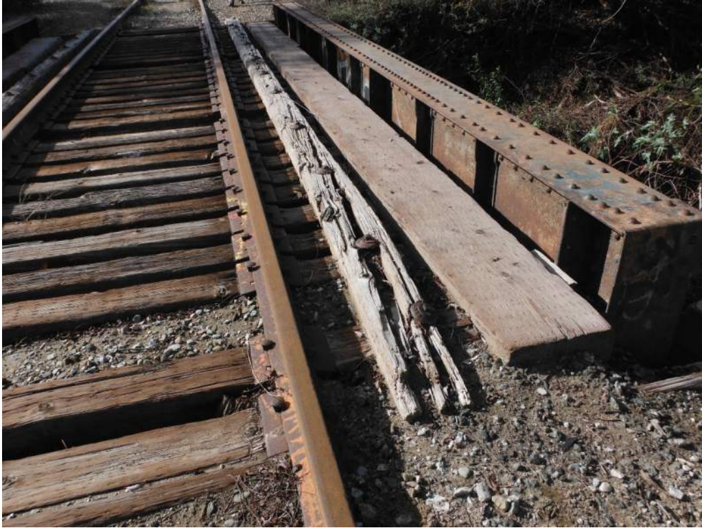
412.25 Damaged curbs at east end
