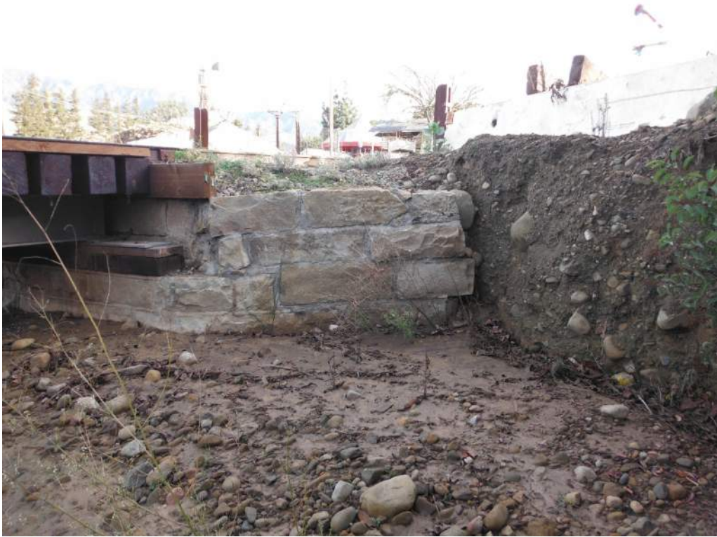
416.32 Erosion around wingwalls (typ.)
