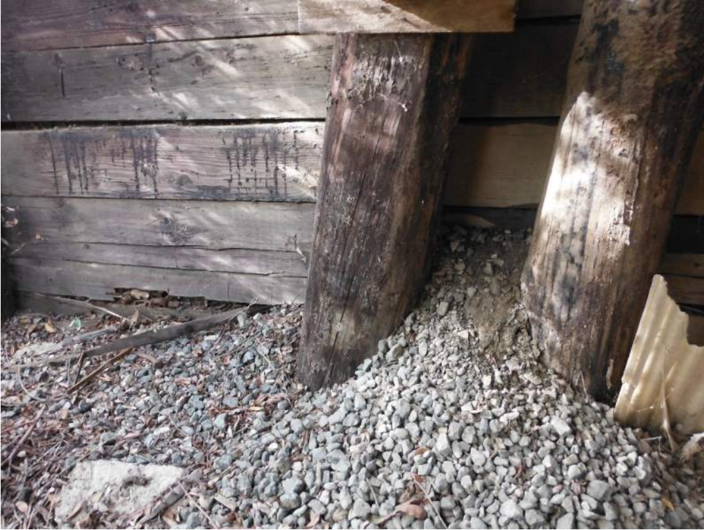
417.24 Abutment 1 bulging and rotten bottom beam with ballast leaking
