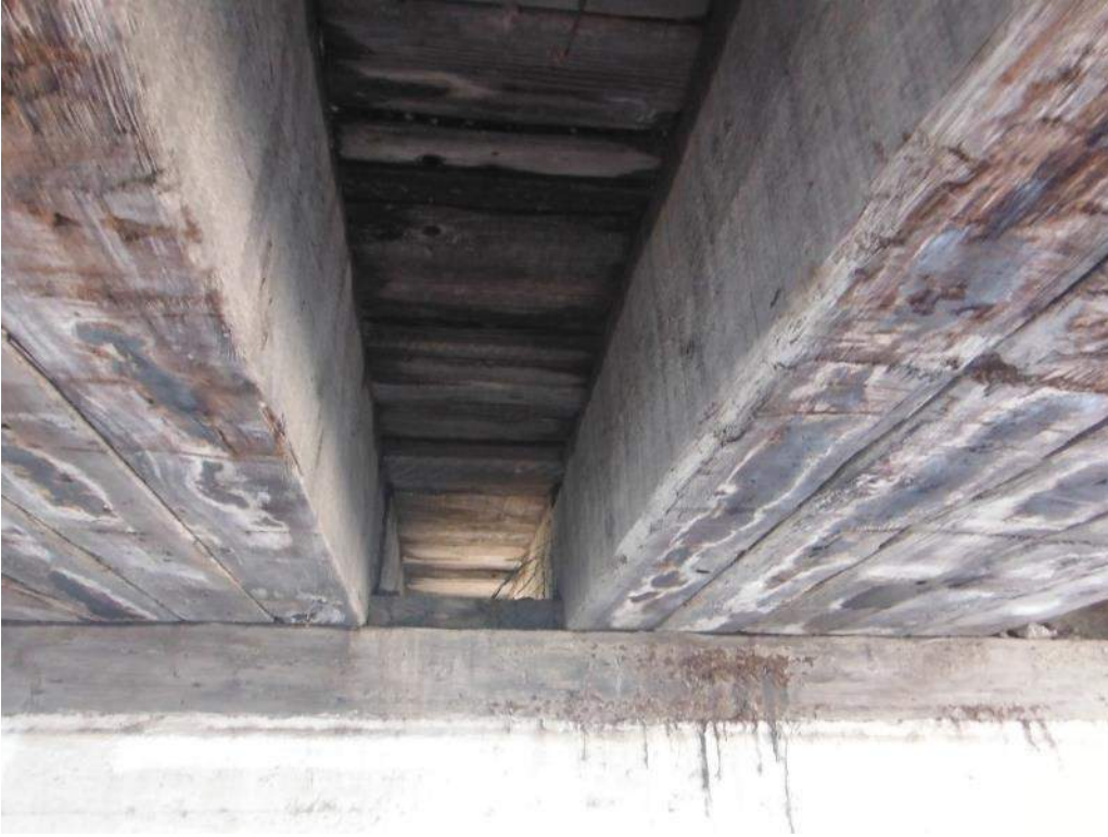
415.69 Stringer 6 rotated 1" at Pier 3 & Abutment 4
