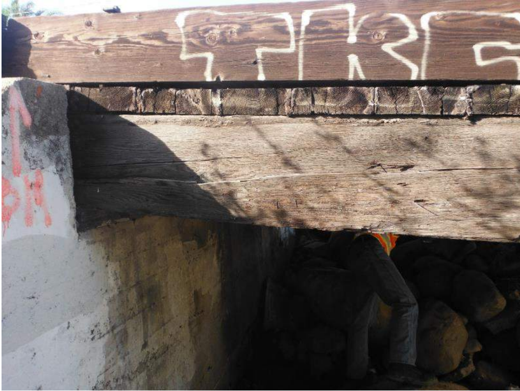
415.69 Stringer 12 crushing – Abutment 1
