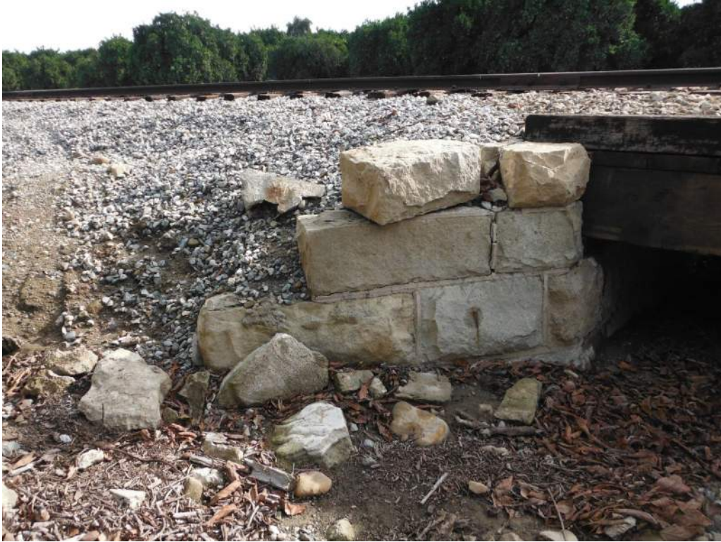
417.96 Loose block in wingwall – Abutment 2
