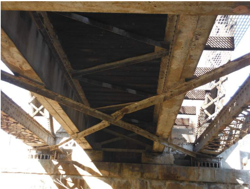
423.28 Minor impact damage to cross bracing near Abutment 1
