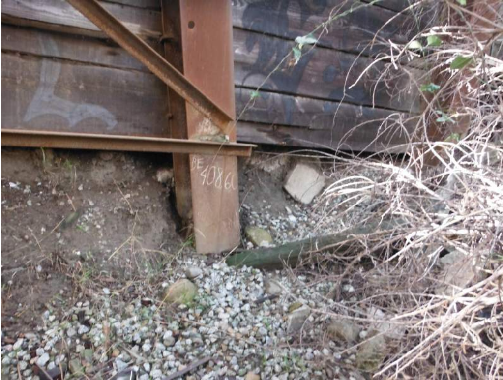
408.84 Scour at the base on Abutment 1
