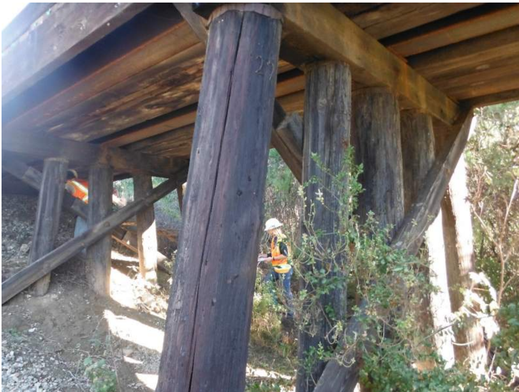
420.46 Pile 1 vertical split, Bent 5
