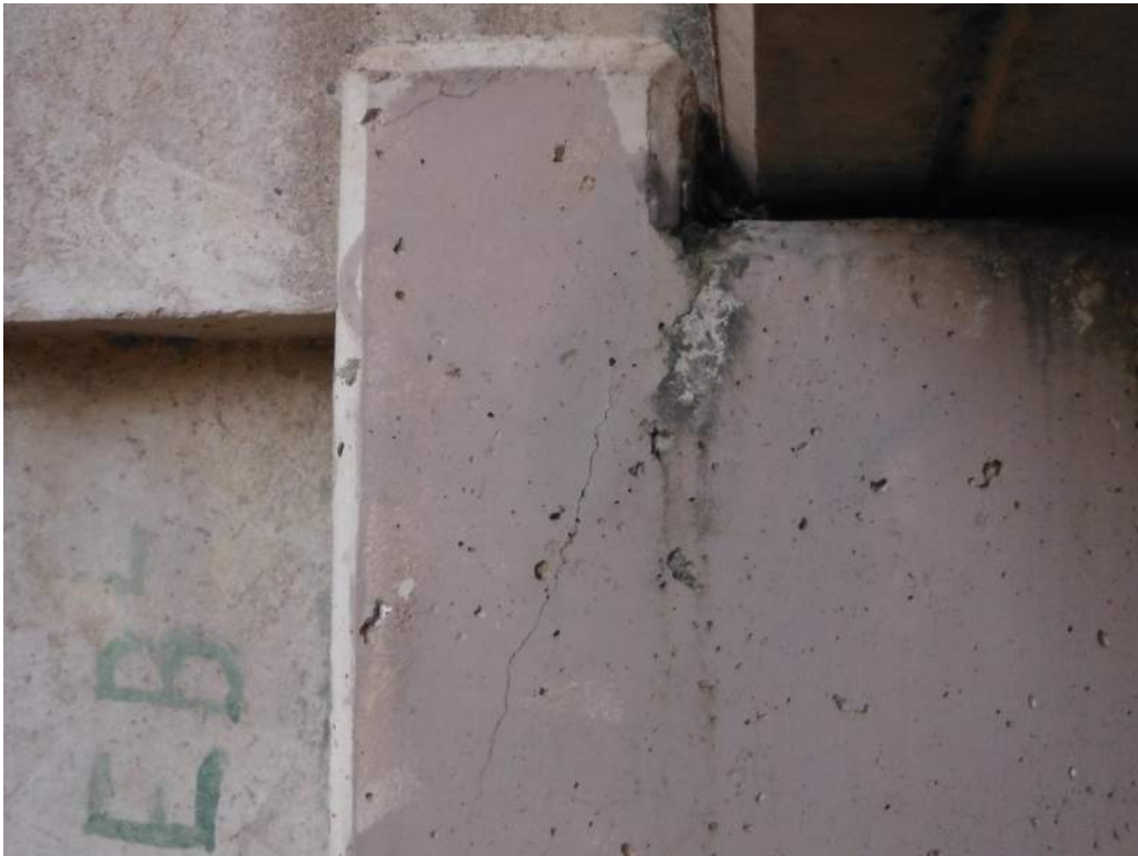
411.97 Abutment 1 South keeper cracking
