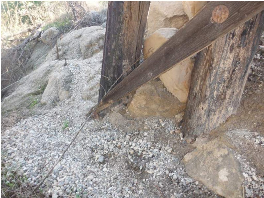
420.46 Span 2, Bent 2 sway brace is broken on right side at pile 5
