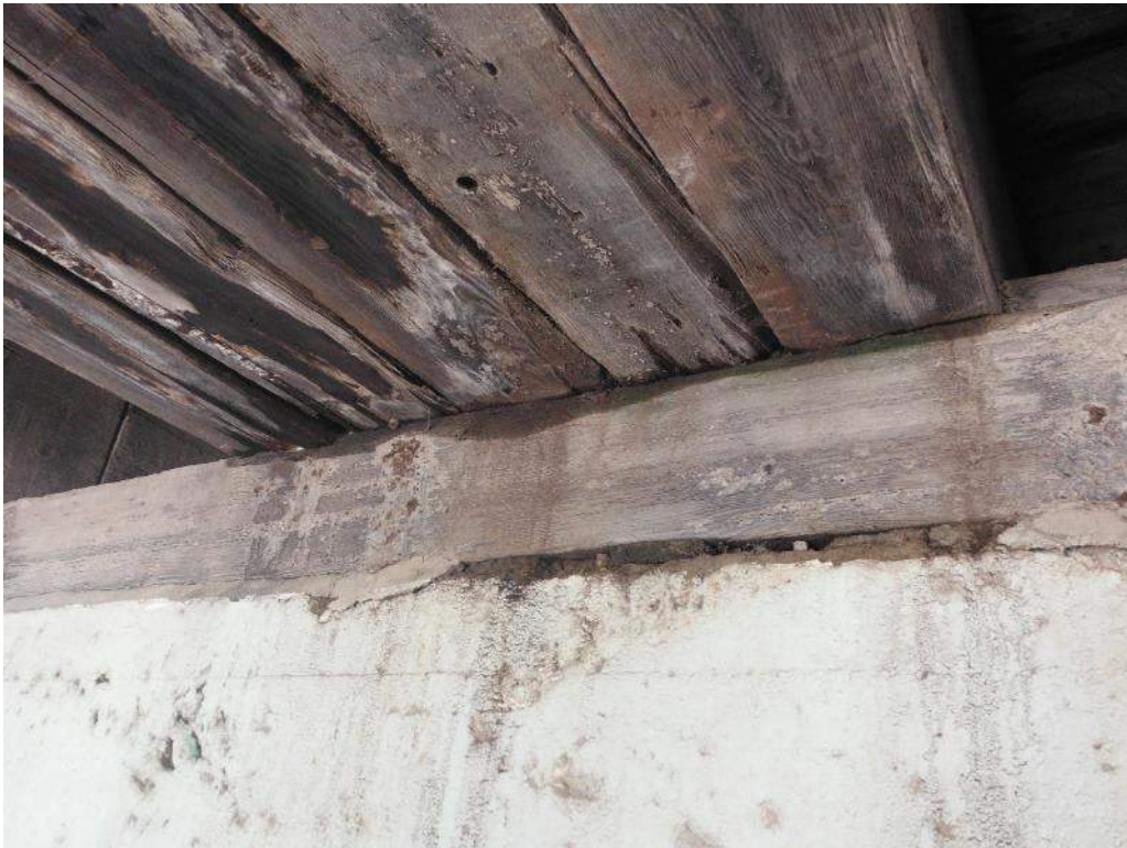
415.69 Stringer 11 crushing - Pier 2
