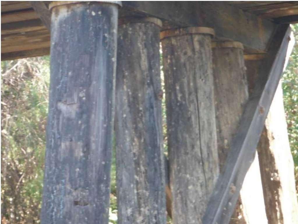
420.46 Pile 1 minor impact, Bent 6
