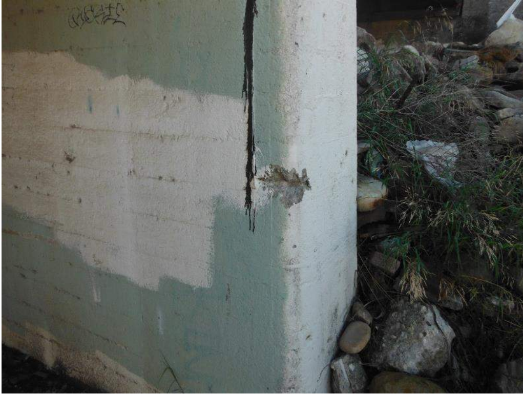
415.69 Spall North Side of Pier 2
