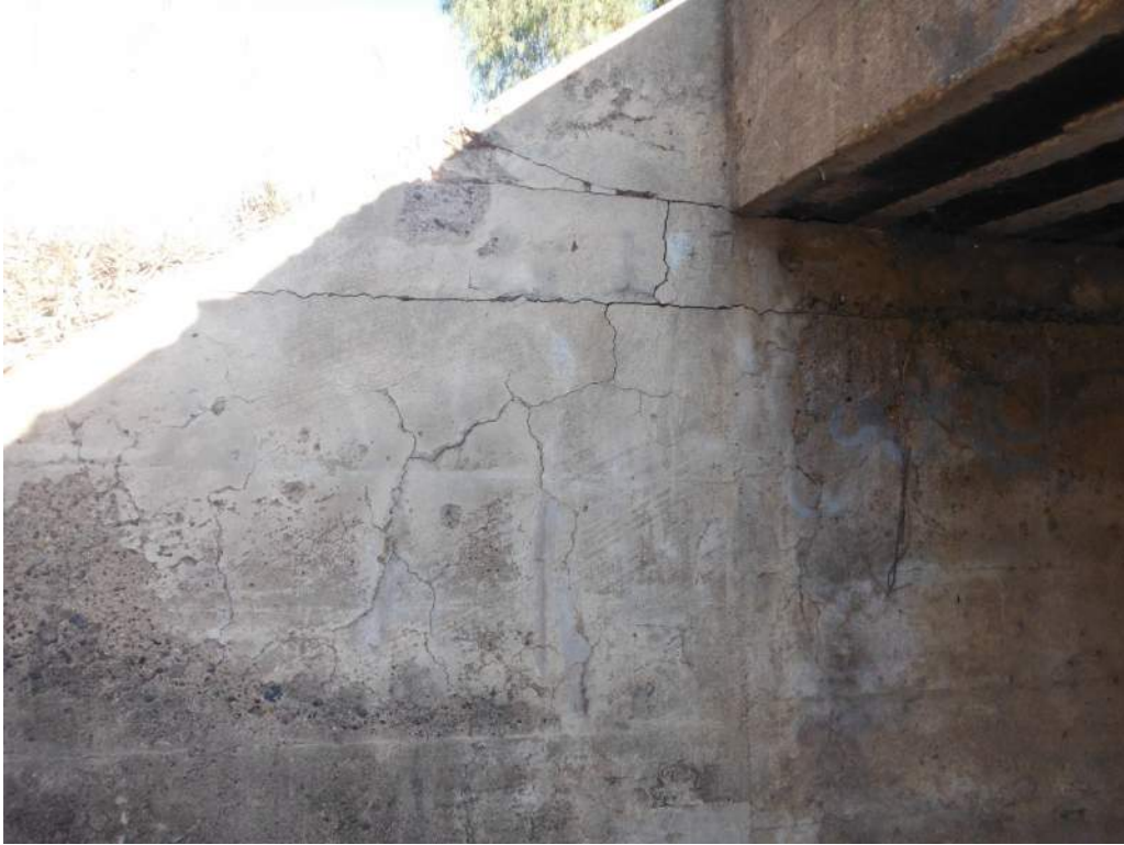
422.89 Abutment 2 cracking – cracking typical both sides each Abutment
