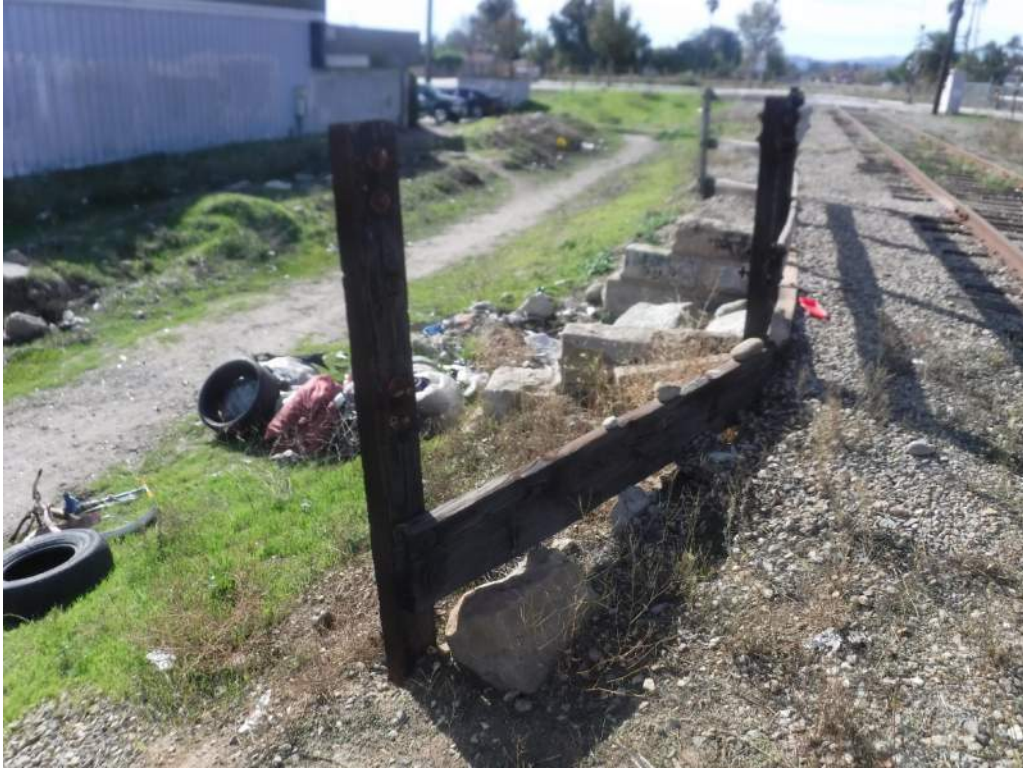
415.20 Southeast wingwall undermining
