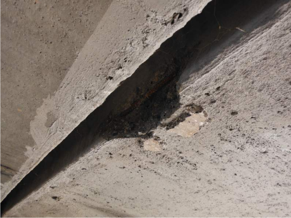
416.21 Cell 3 concrete spall on underside of top slab. Rebar exposed
