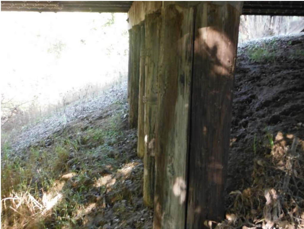
419.92 Pile #5 is Split, Bent 6
