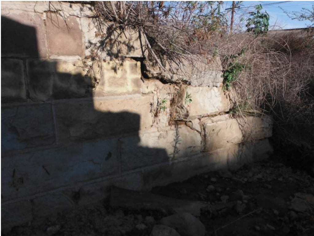
422.53 Southeast Wingwall Blocks Loose
