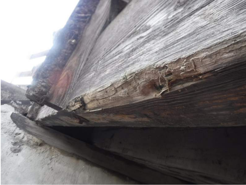
409.74 Stringer 1 impact damage
