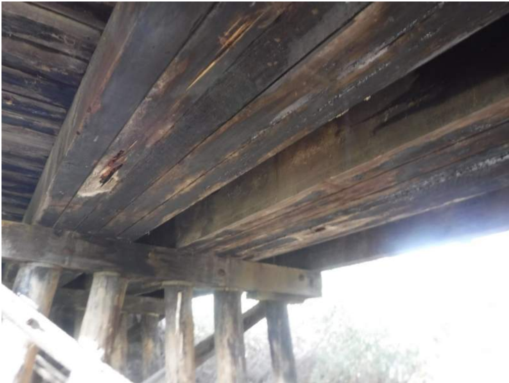
417.24 Stringer 10 failed, Span 3
