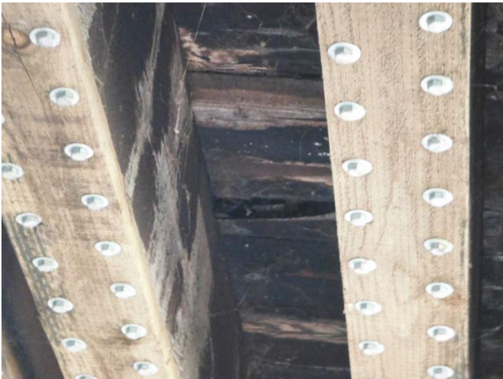
419.92 Hole beginning in deck between stringer 6 and 7 - Span 4
