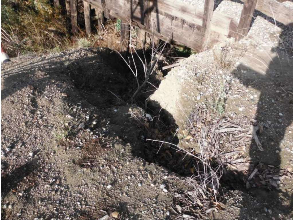
417.24 SE wingwall erosion
