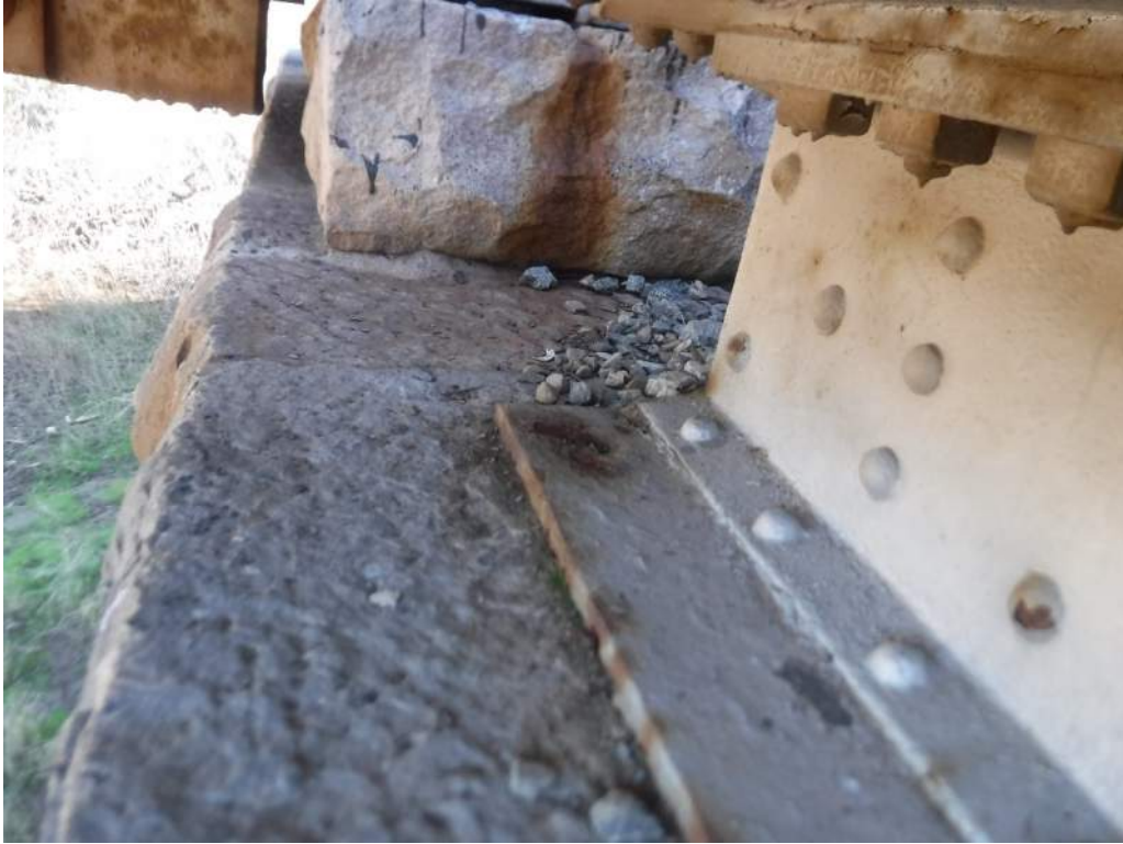
423.28 South bearing, Abutment 2 – Missing NW anchor
