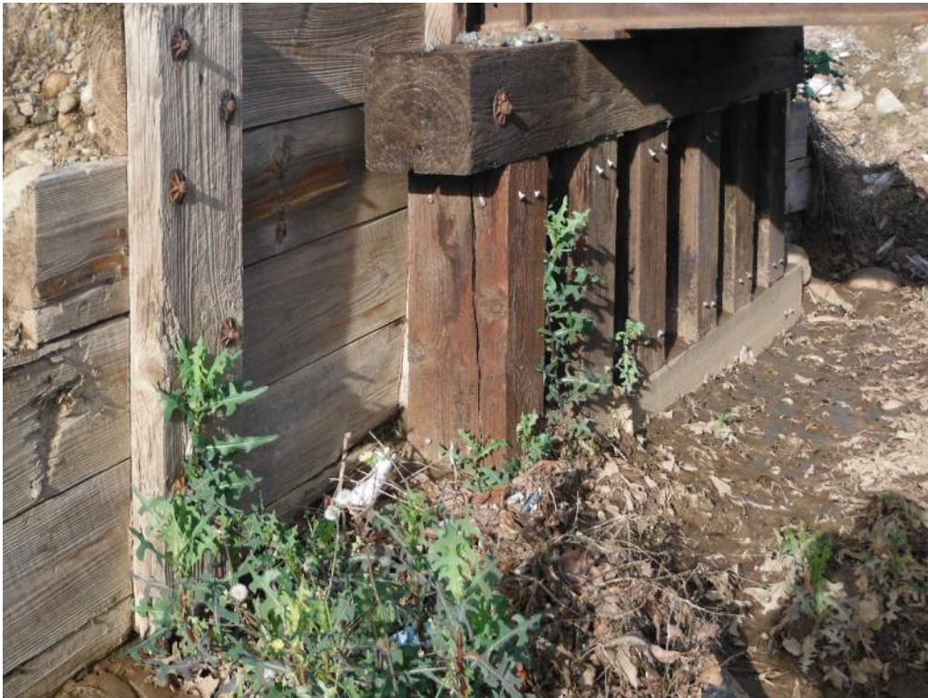
416.63 Split pile 6 at Abutment 1, typ multiple locations
