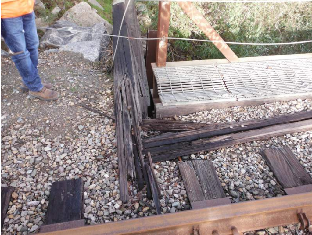
408.84 Rotten/failing backwall at Abutment 1
