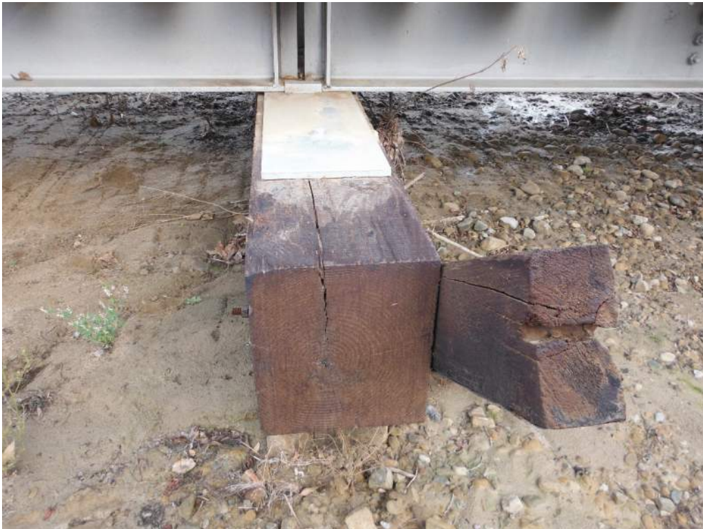
416.32 Vertical split in cap – Pier 2
