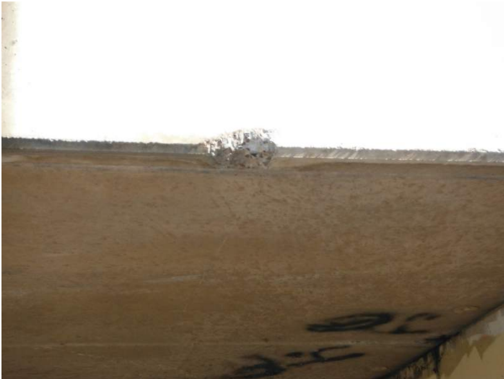
423.44 Minor spall - south side Span 13
