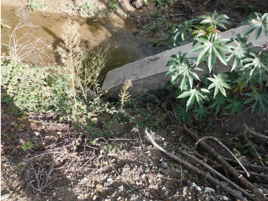
410.40 Undermining and Scour behind NW Wingwall Upstream
