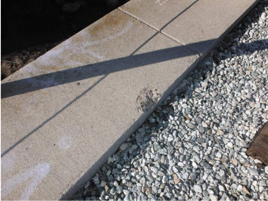
423.44 Walkway Spall on Span 2 and multiple locations
