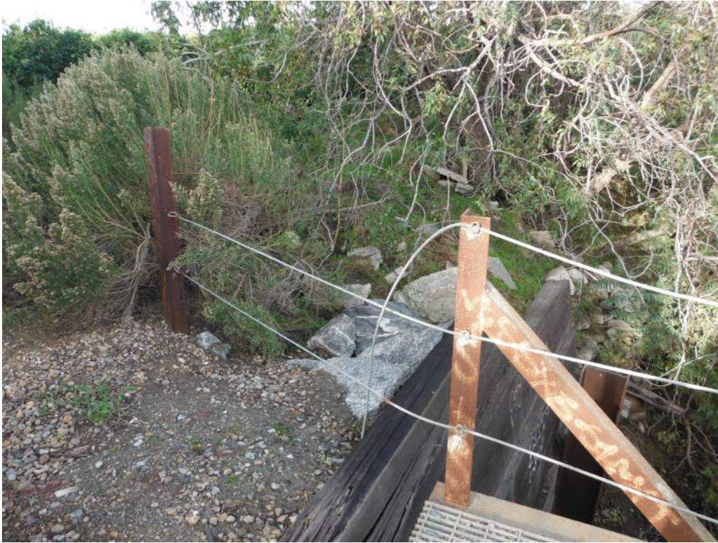
408.84 Loose/broken handrail cable – Span 1 north side
