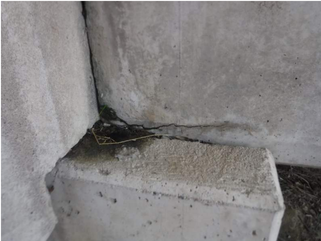
411.97 Girder 1 cracking at Abutment 1
