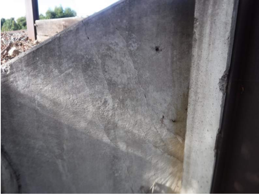
411.97 Southwest wingwall cracking
