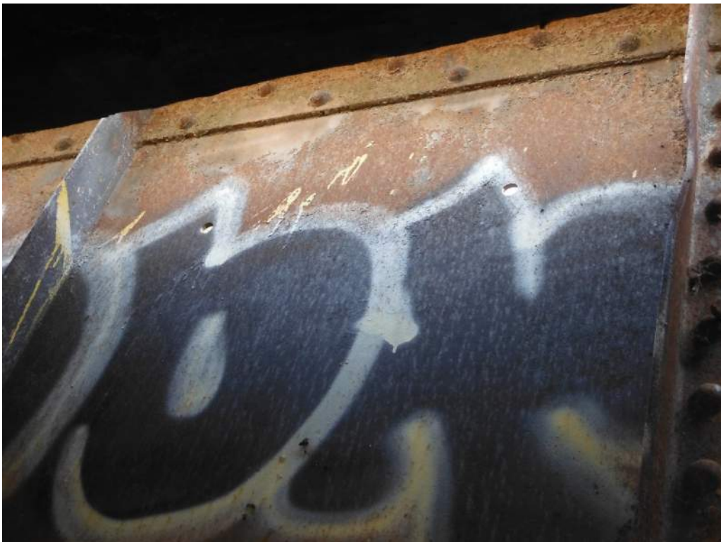
412.25 Hole in web and stiffener damage at midspan G2
