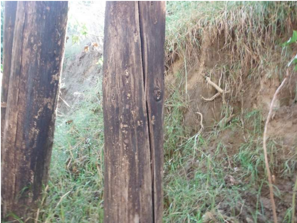
419.92 Piles #2, #3, and #4 are split 1" - Bent 2
