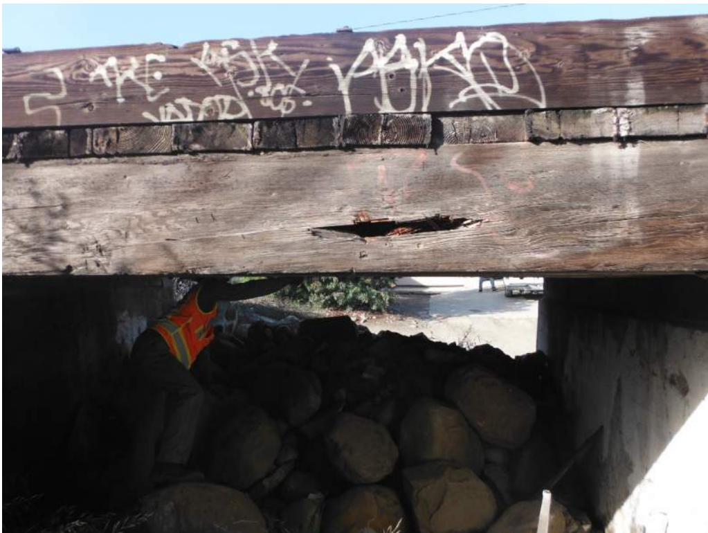
415.69 Stringer 12 is rotten/failed – Span 1
