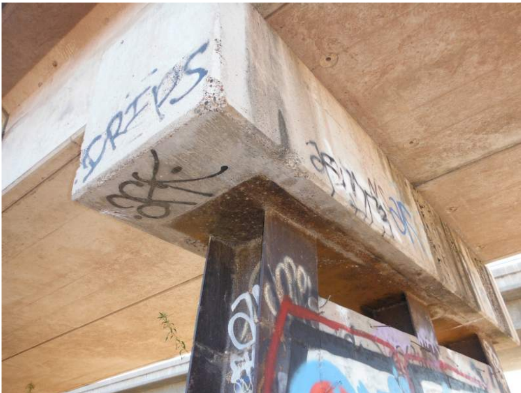
423.44 Minor spall on bottom corner of pier cap, Pier 5
