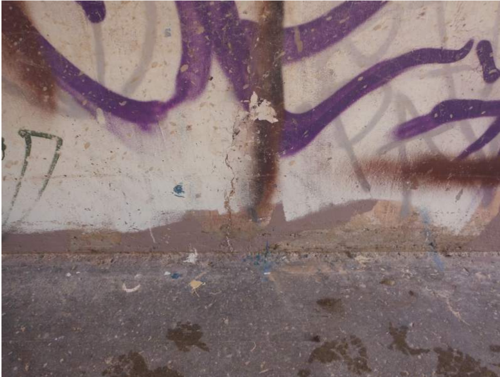
408.02 Vertical crack center of Abutment (typ.)
