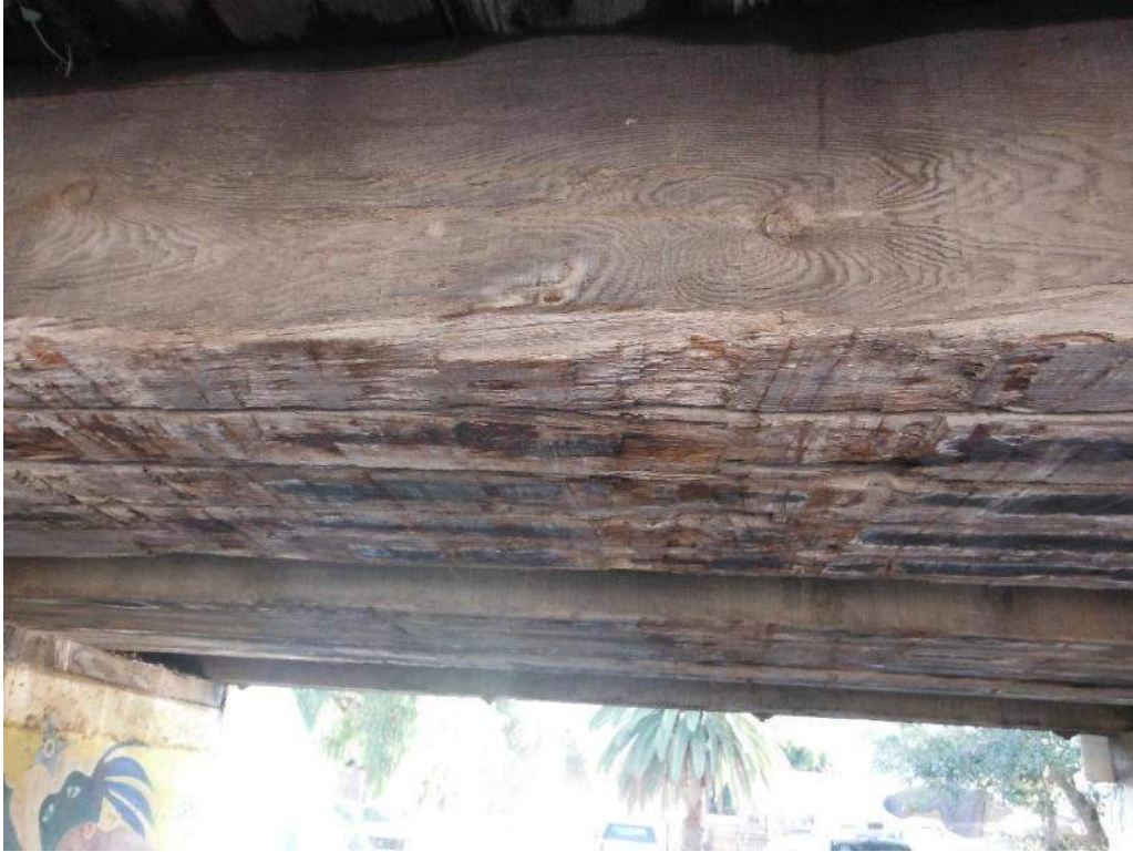
415.69 Impact damage on stringers (typ.)
