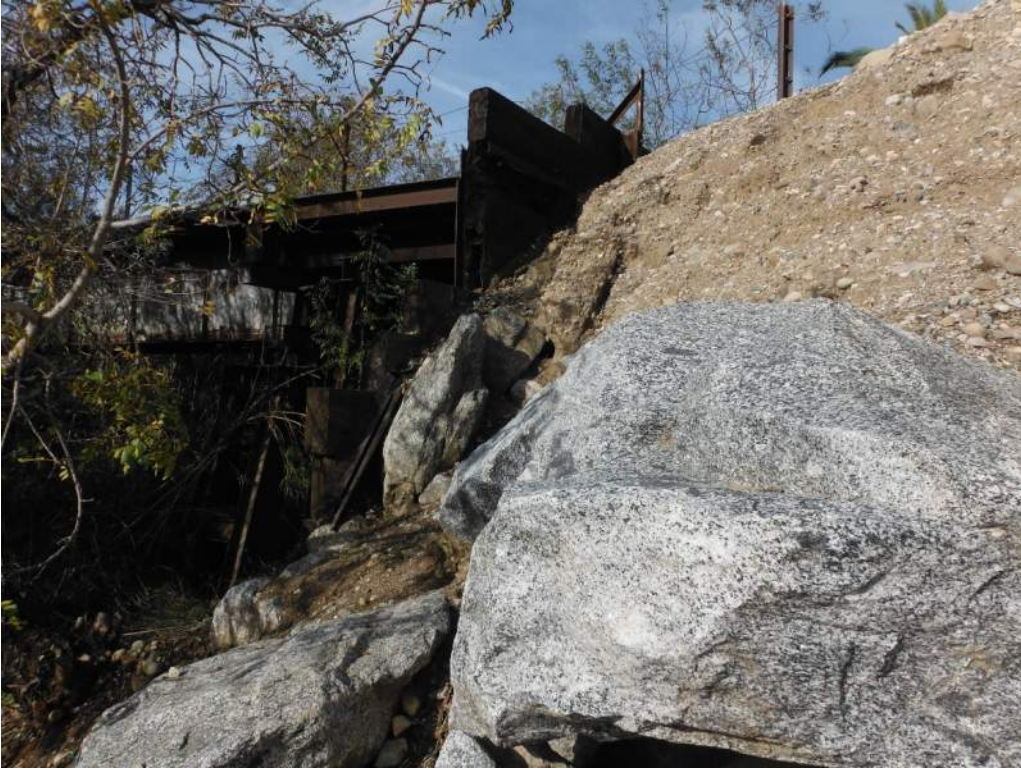
408.84 Erosion at Southeast slope behind wingwall
