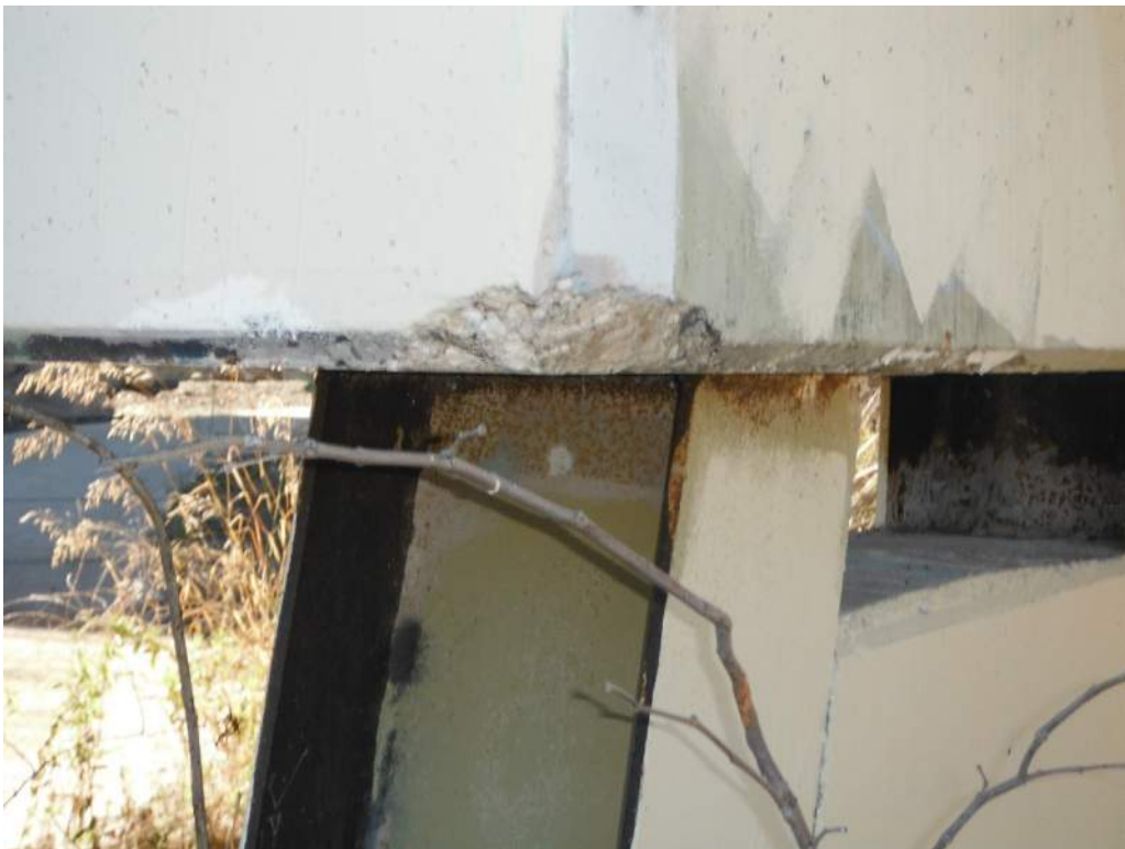
423.44 Spall NE bottom corner of cap, Pier 14
