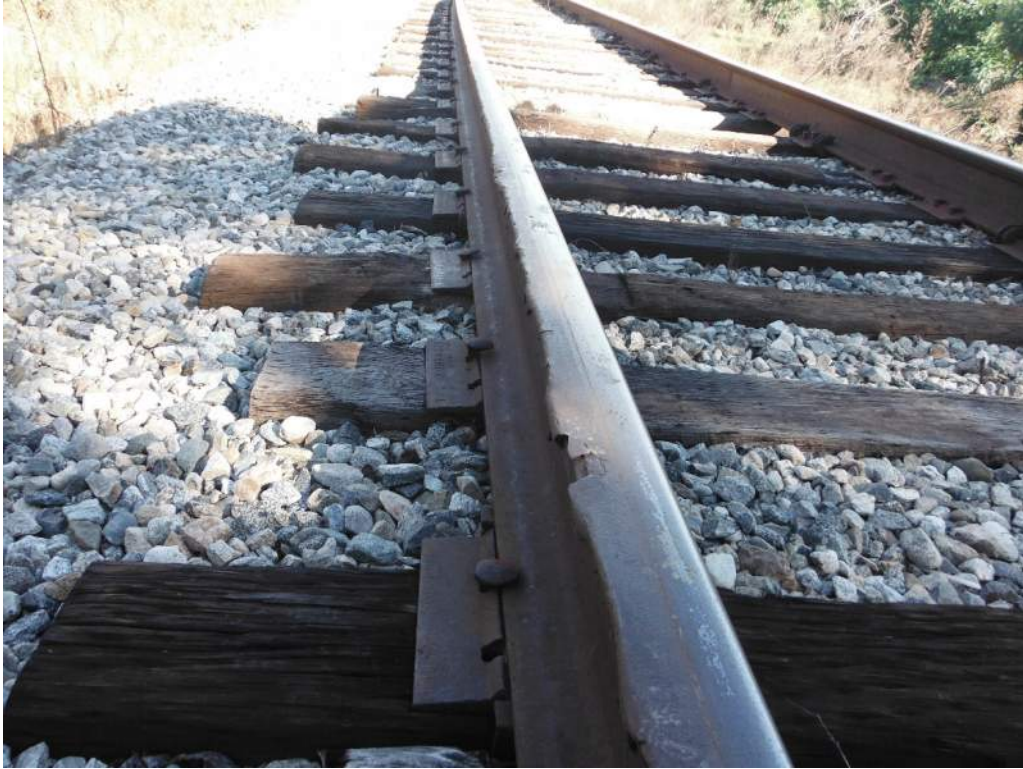
419.92 Rail section loss – east and west sides and along length of bridge
