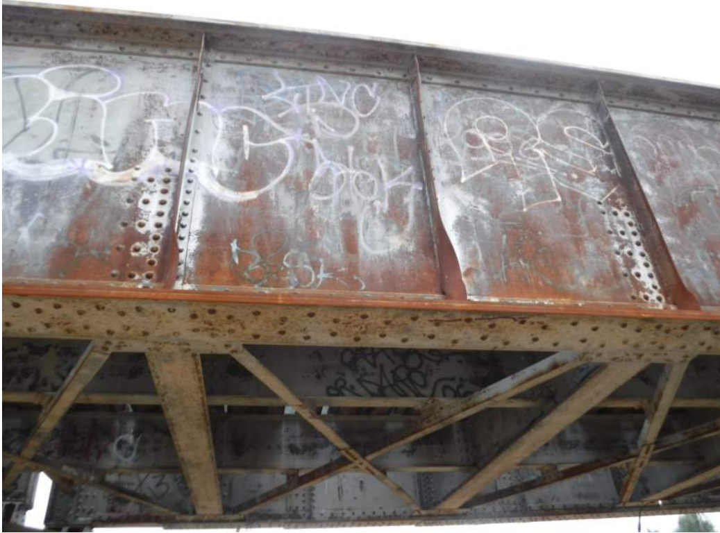
429.79 Multiple stiffeners Impact damage - Span 1 north side
