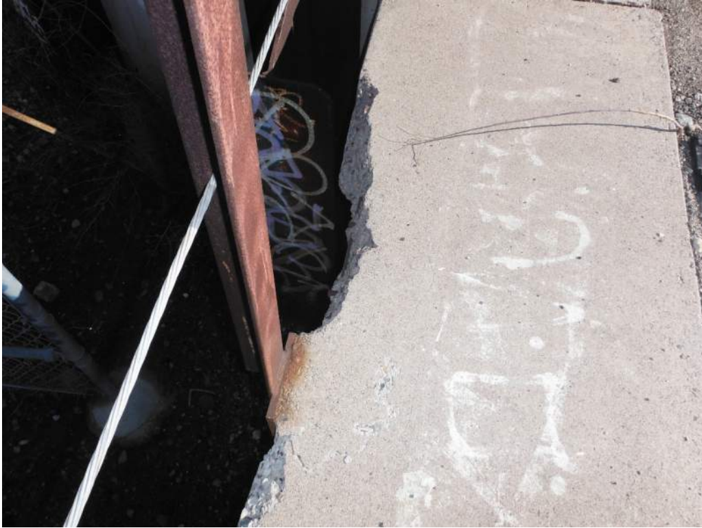
425.15 Spall with exposed rebar - Span 2 north side
