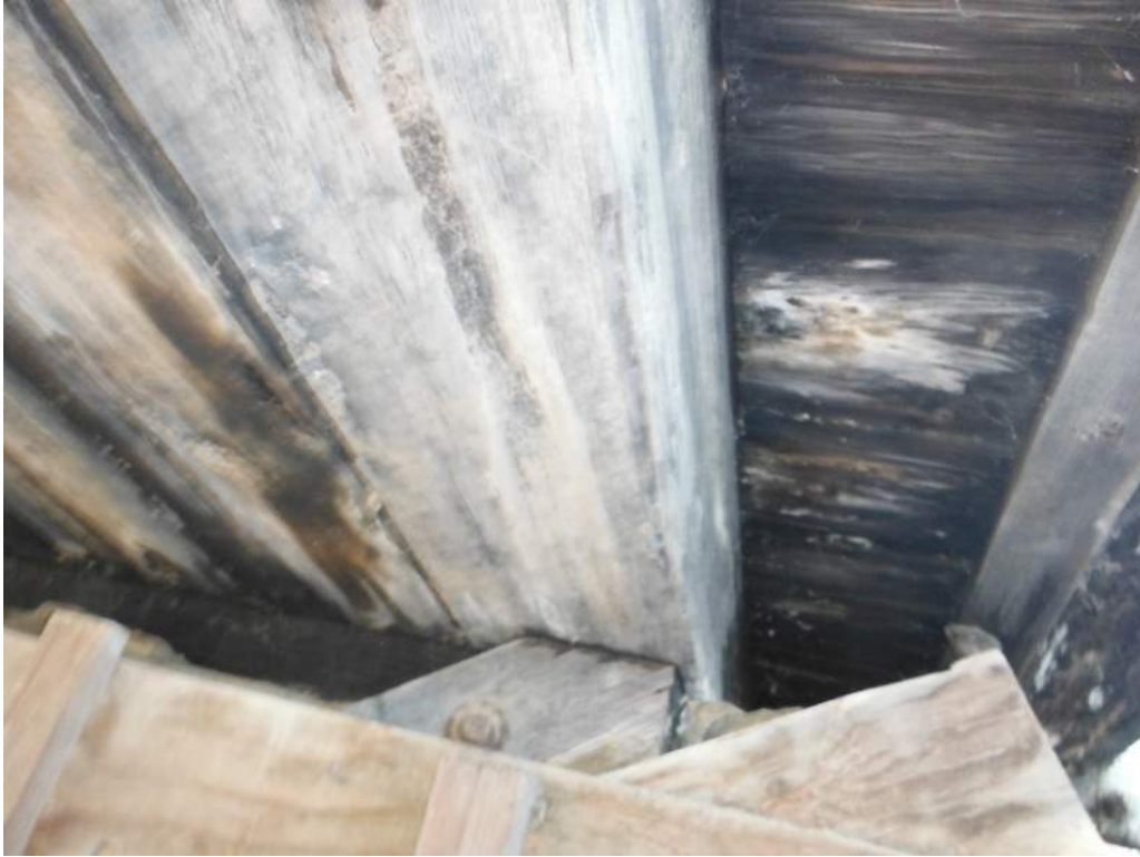
421.23 Stringer 12 Splitting, Span 2
