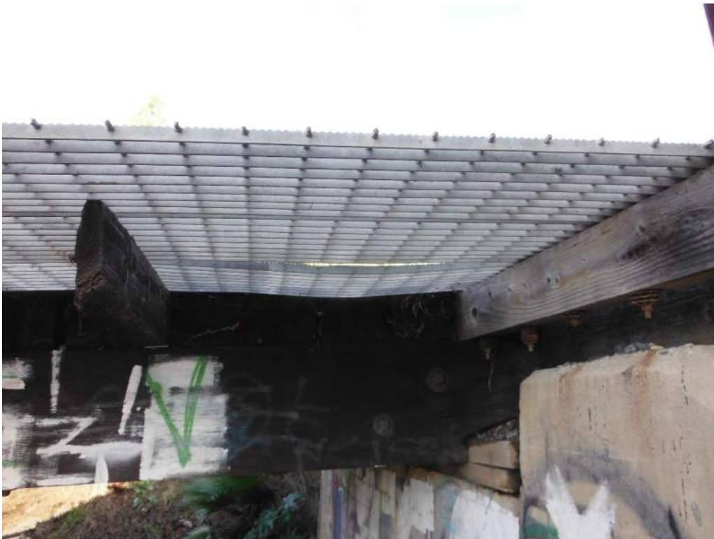
407.48 SE Walkway Panel Deflection Damage
