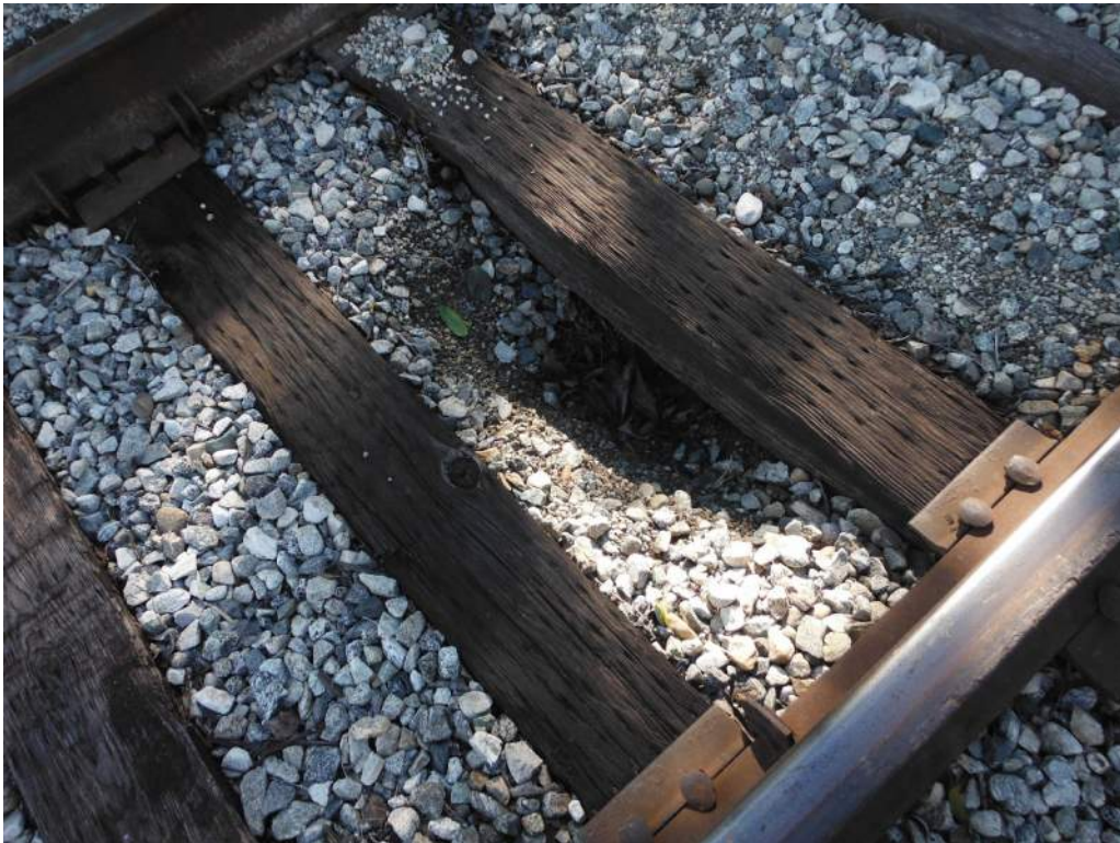
419.92 Holes in ballast near abutment 1 & 7
