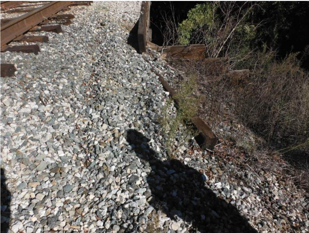
419.92 Ballast overtopping SW ballast retainer
