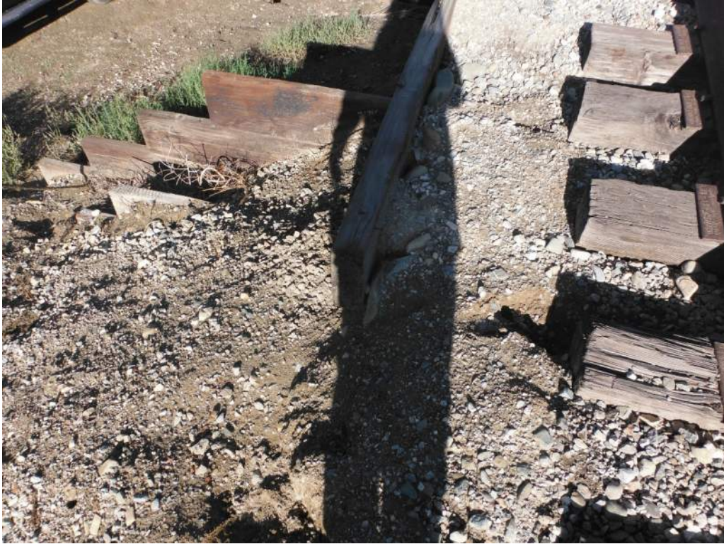
420.20 Typical holes in ballast – east and west ends
