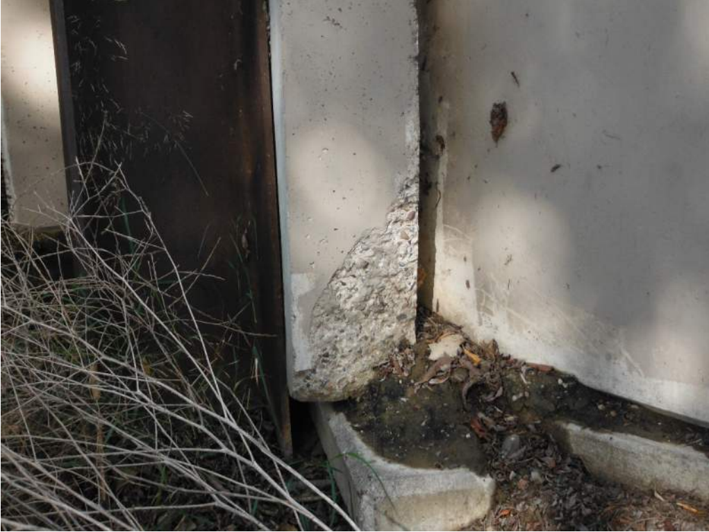
411.97 Southeast Backwall Spall
