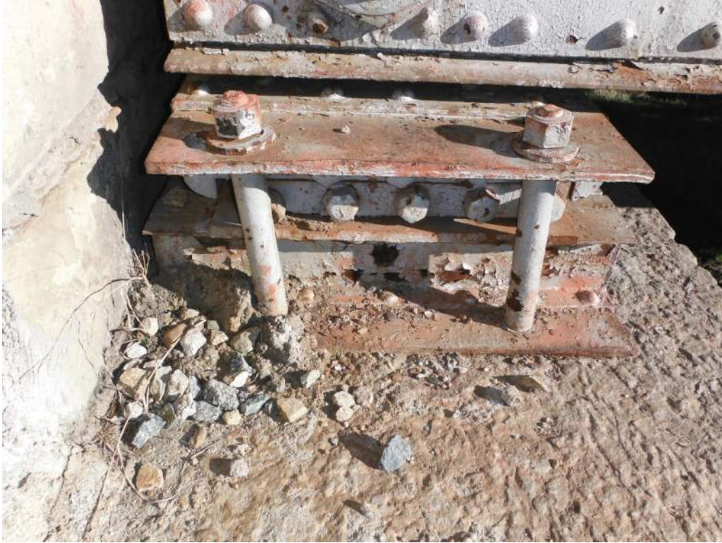
423.28 Abutment 1 bearings rocked
