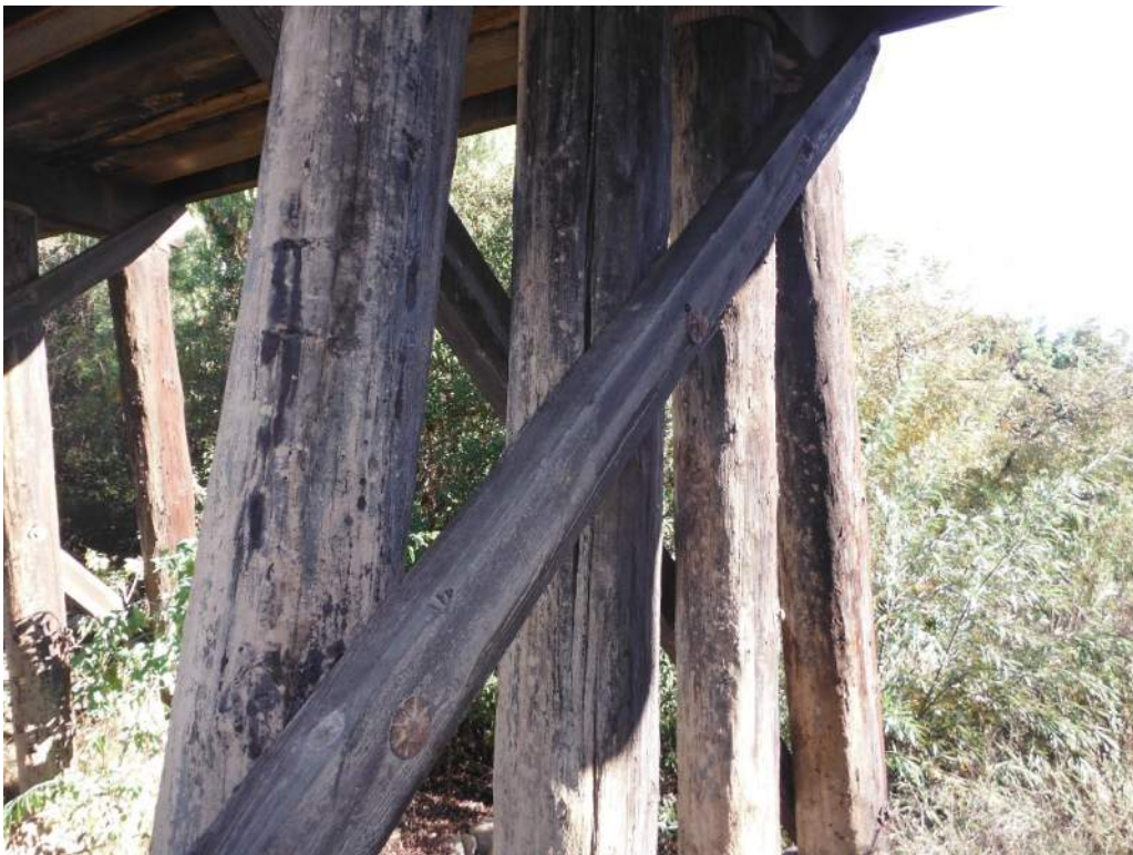
420.46 Pile 3 vertical split, Bent 3
