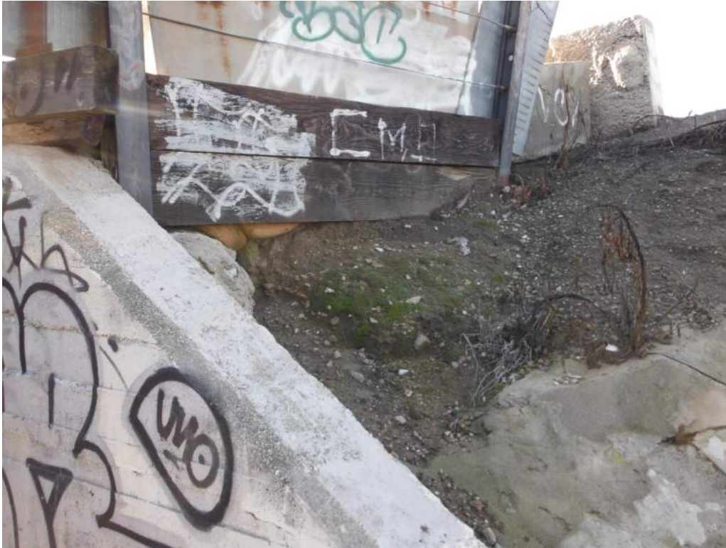
407.48 Northwest Wingwall Undermining
