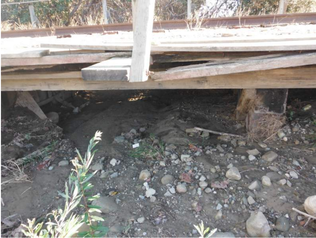
421.23 Walkway Timbers Broken on North Side Span 2
