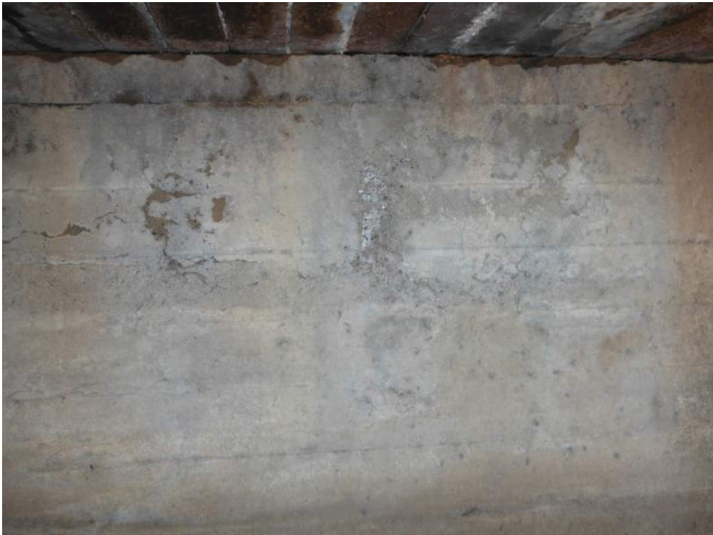
422.89 Abutment scaling – typical each Abutment
