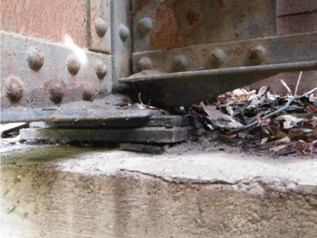
410.40 Broken grout under bearing plates, Abutment 2
