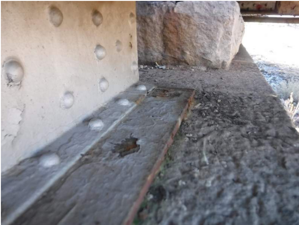
423.28 North bearing, Abutment 2 – Missing SW anchor
