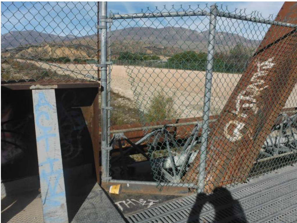
415.59 Fence breach over Pier 2, north side
