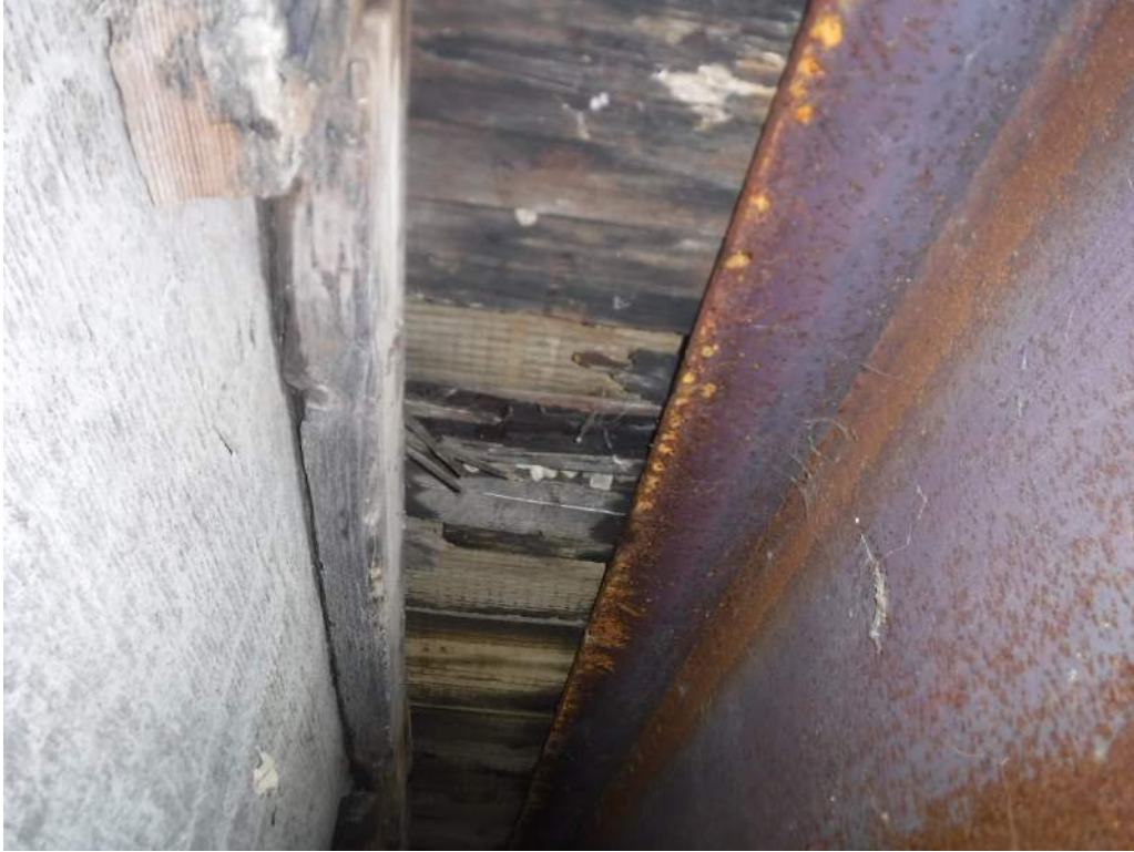
420.46 Holes in deck planks, Bent 6
