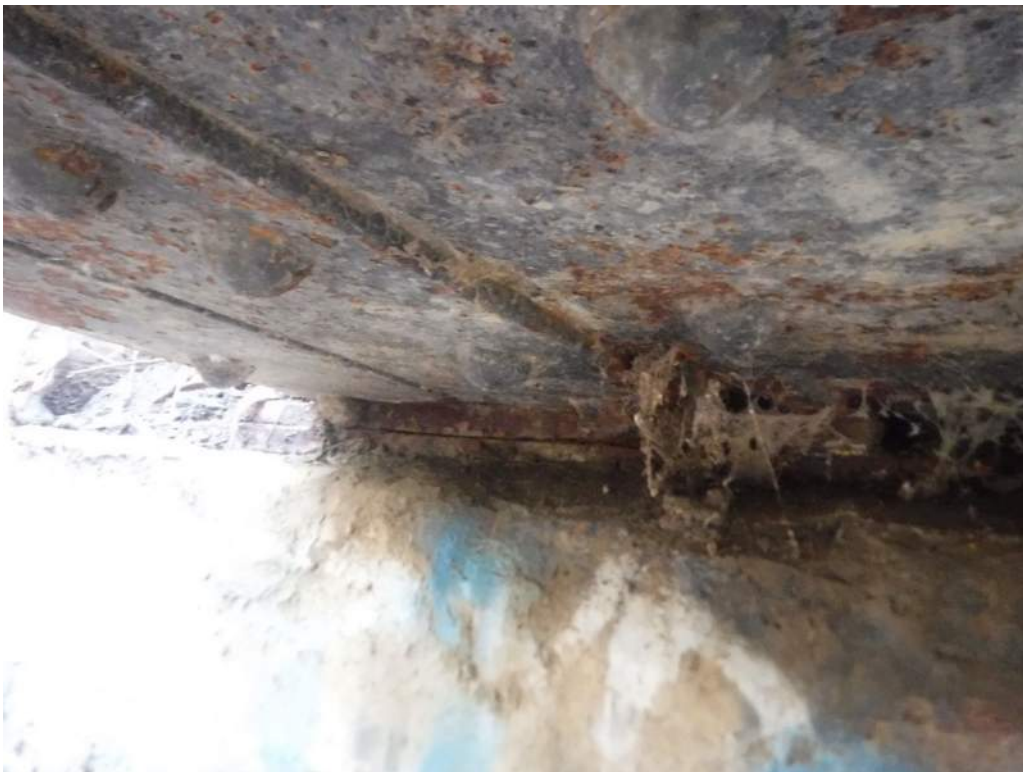
412.25 Minor section loss/pack rust at bearings (typ.)
