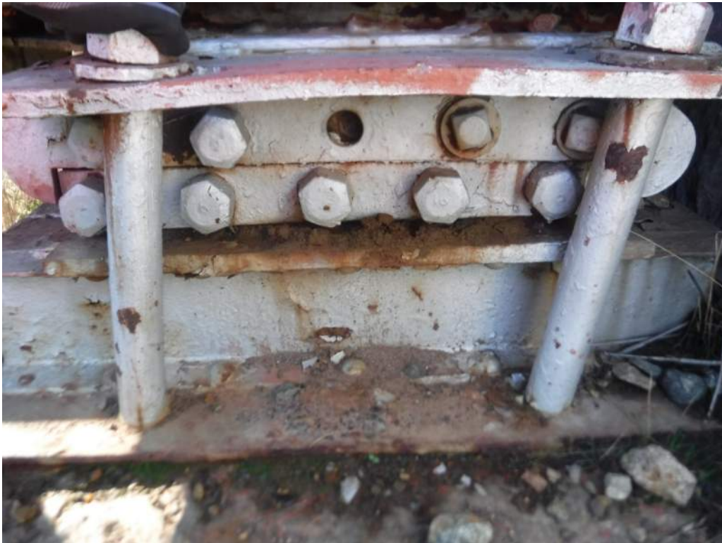
423.28 Bolt missing at Northwest bearing bridge rollers
