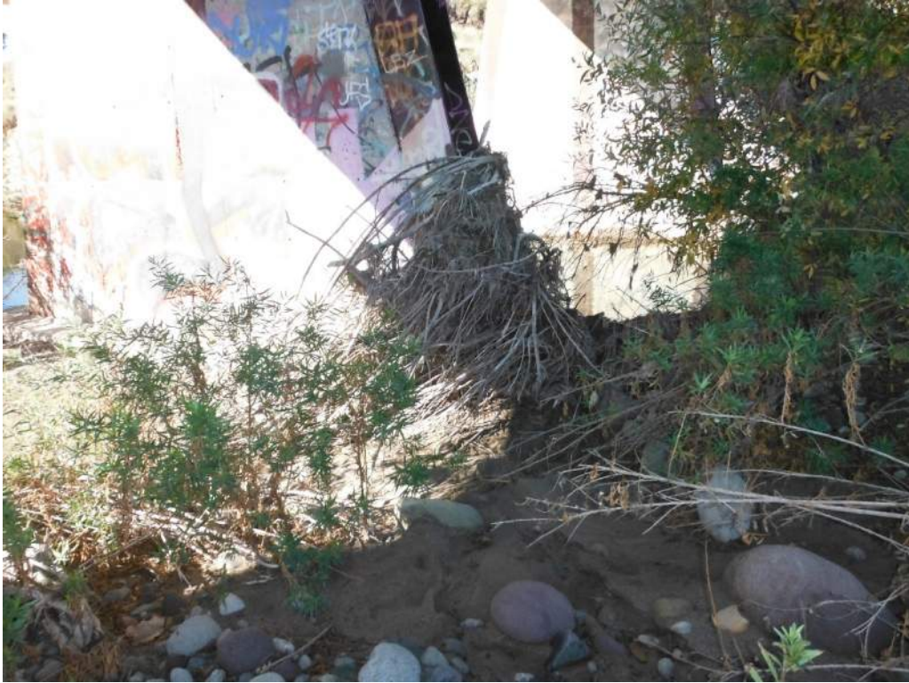
423.44 Debris Upstream on Pier 4
