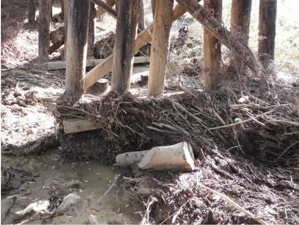
417.24 Span 3 sash brace covered in dirt and debris at bent 3
