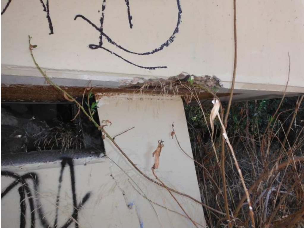
423.44 Spall with Exposed Rebar – Pier 15 west side
