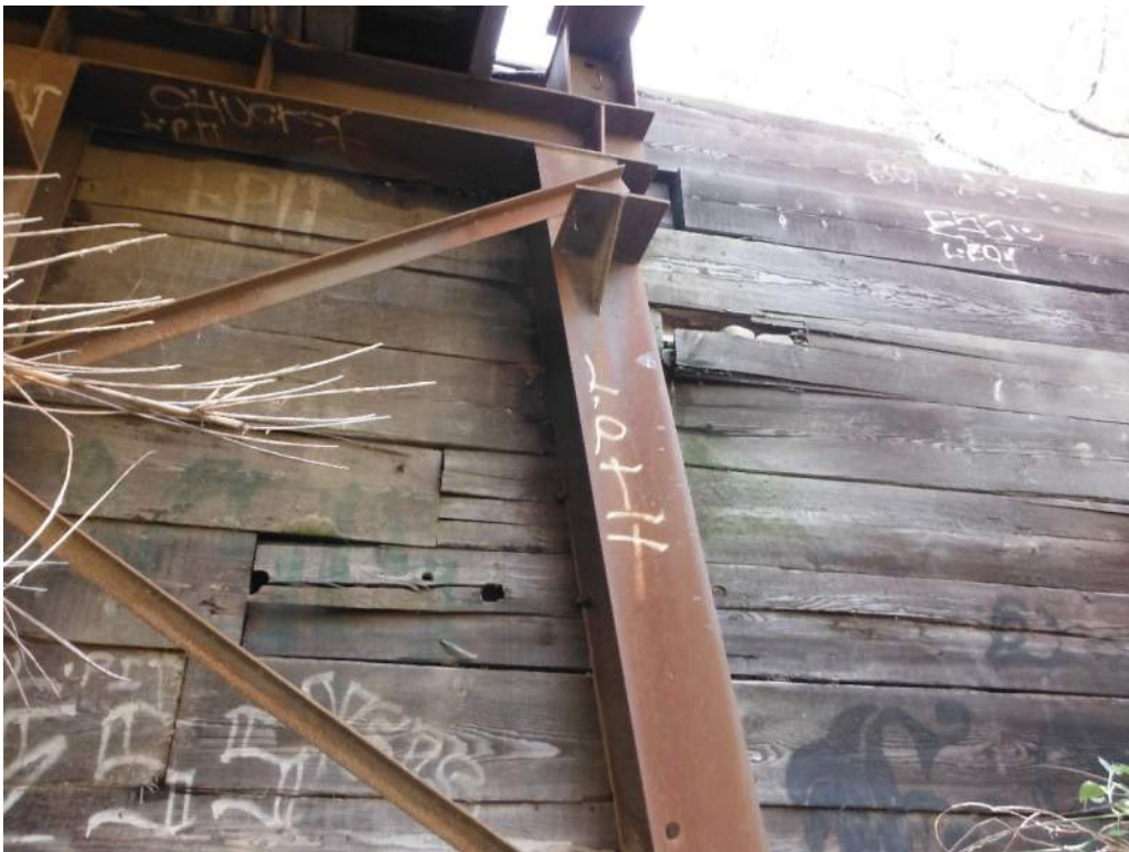
408.84 Abutment 1 Backwall rotten
