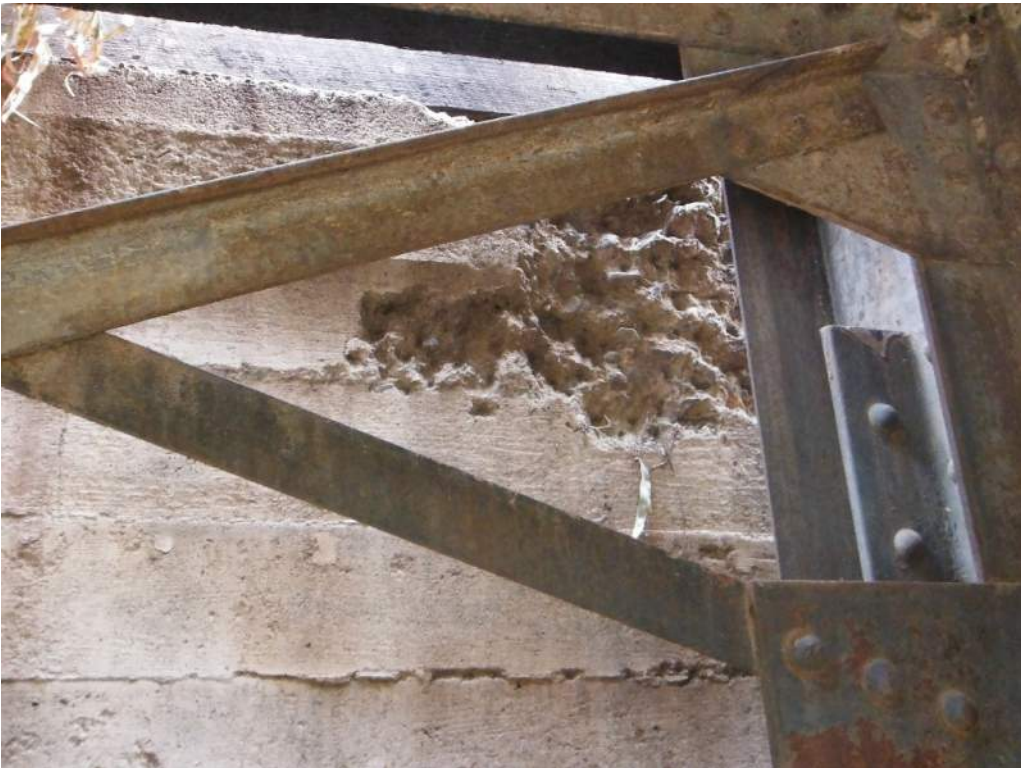
410.40 Backwall spall – Abutment 2
