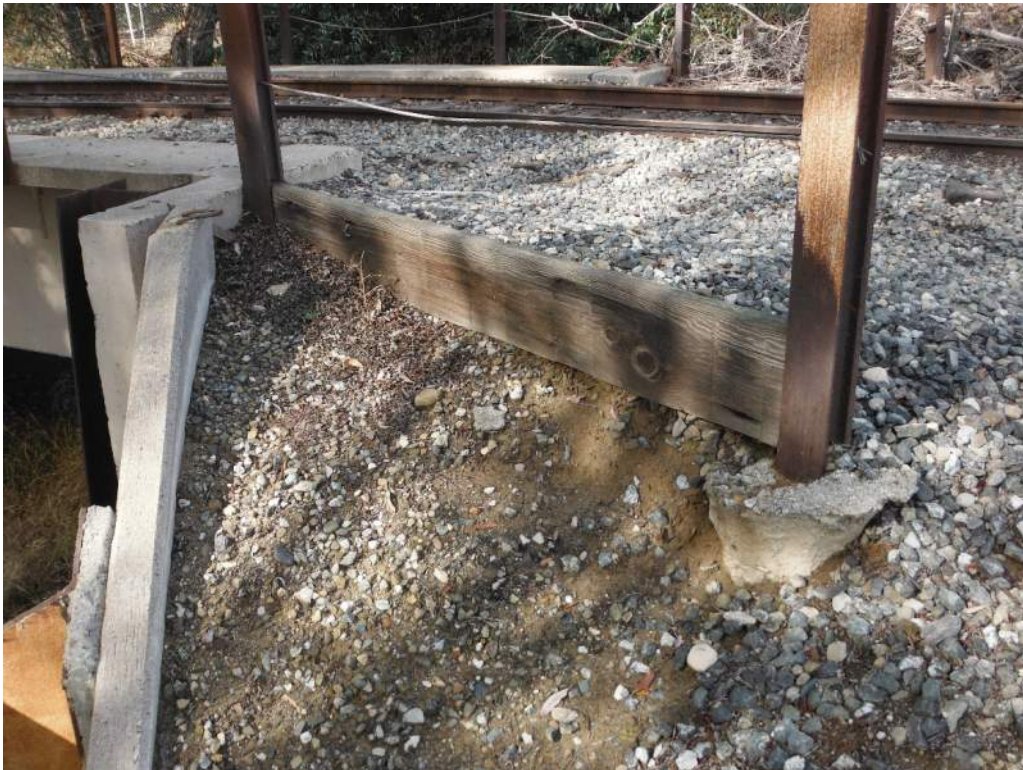
411.97 Abutment 2 undermining SE Ballast retainer
