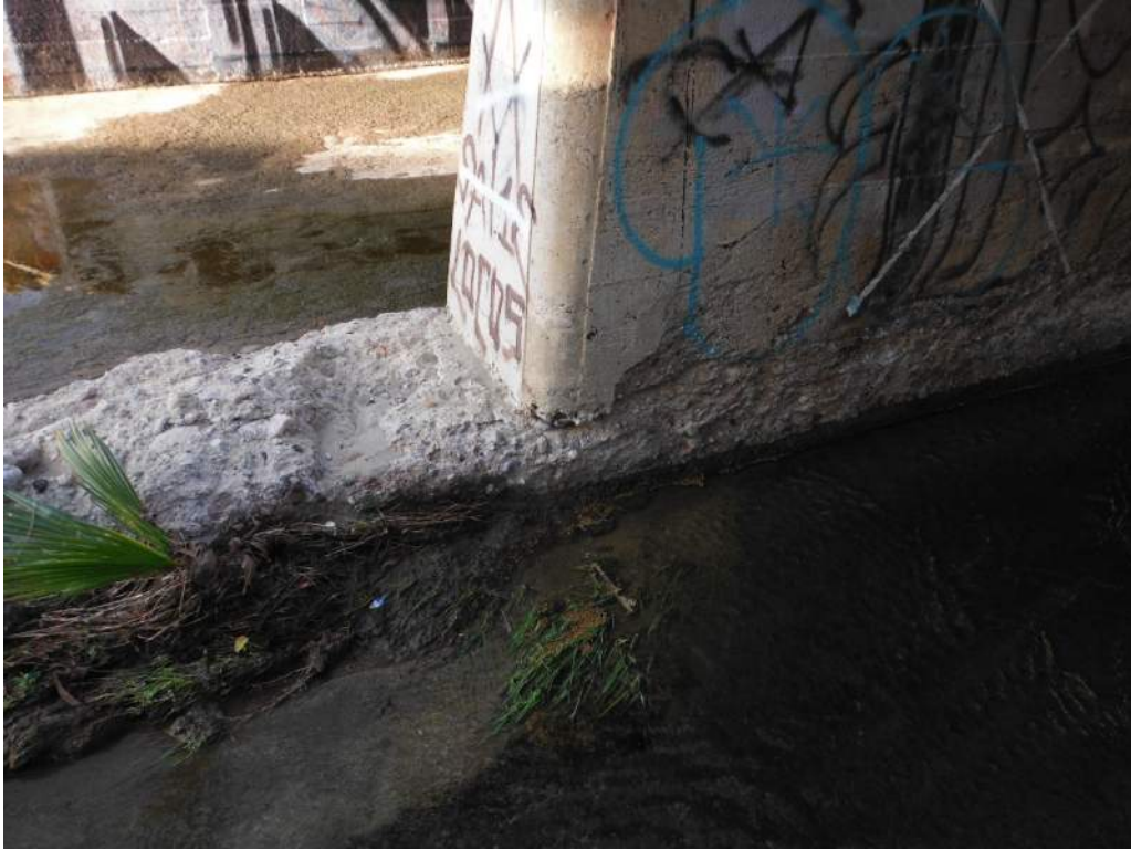
407.48 Scaling at Base at Abutment 3
