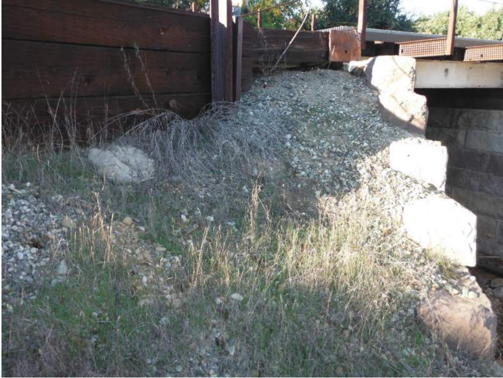
422.53 Southwest ballast curb undermined
