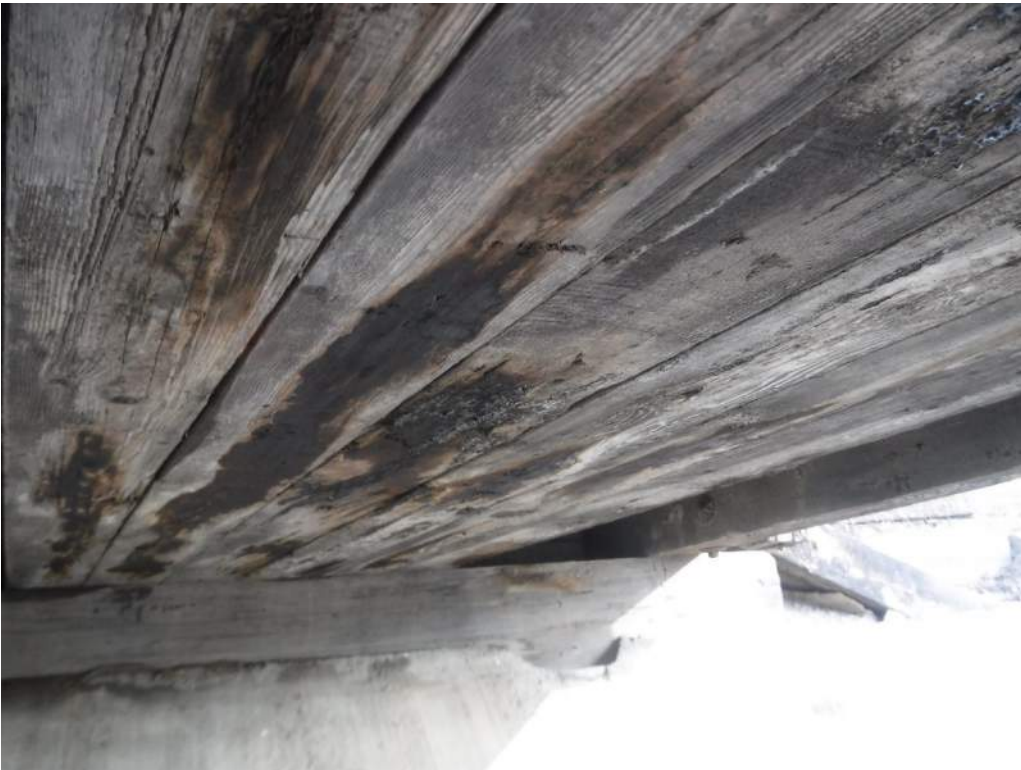
409.74 Stringer 8 impact damage
