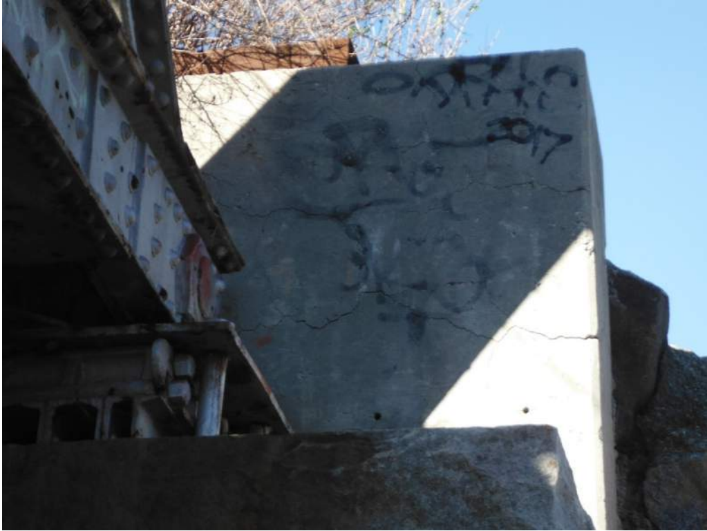
423.28 Map cracking Northside of backwall - Abutment 1
