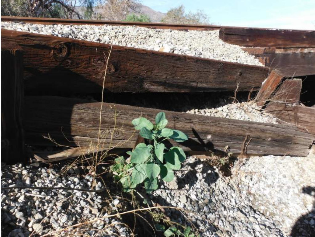
420.46 Southwest wing failing
