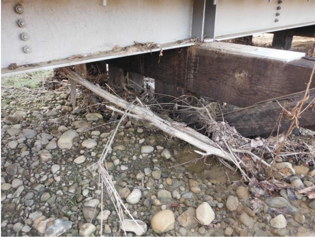
416.32 Debris on piles – Pier 2
