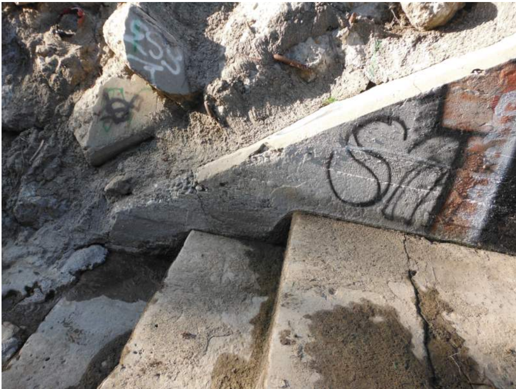
407.48 Southwest Wingwall Crack
