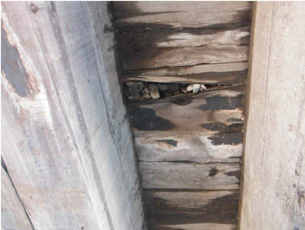
415.69 Poor ballast planks (typ.)
