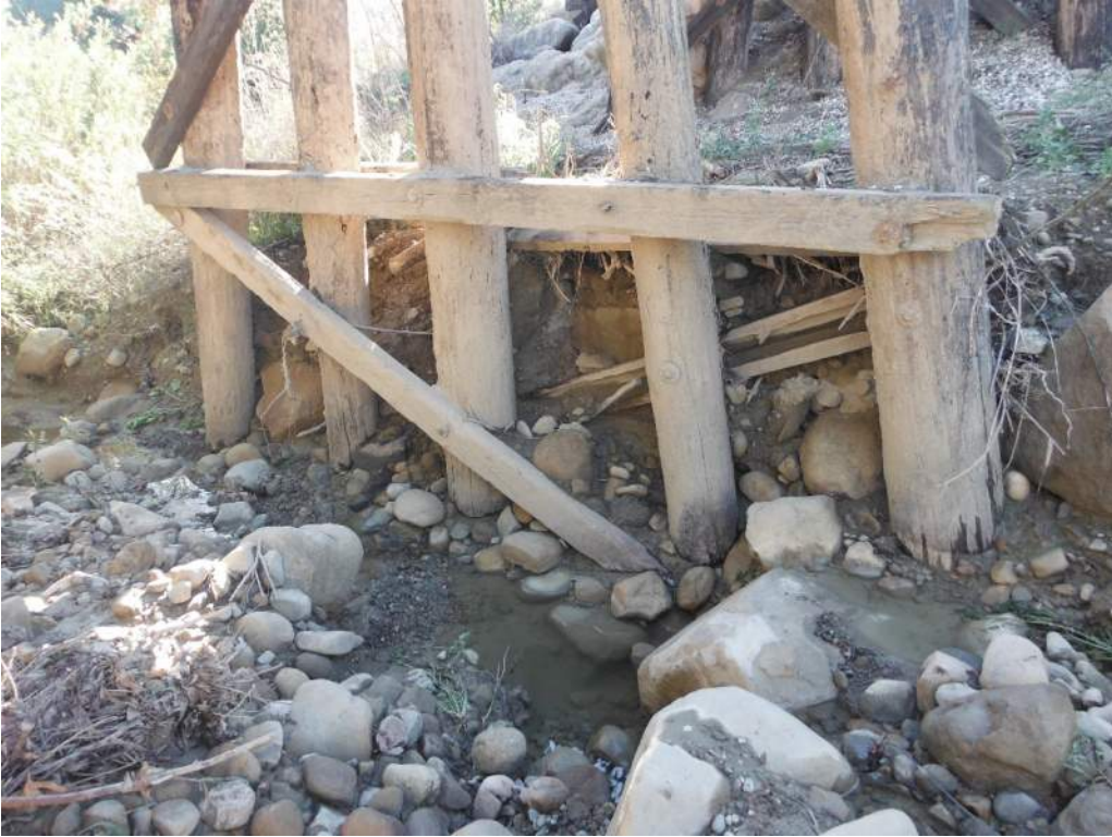
420.46 Scour between Bent 3 and 4
