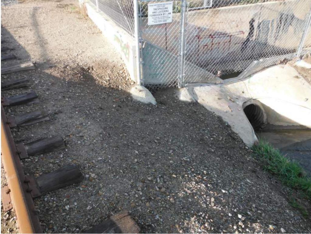
408.02 Fouled Ballast across Culvert
