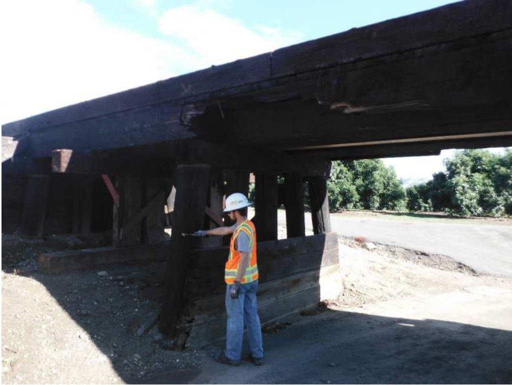
420.20 Exterior stringer failed due to impact - Span 3 typ
