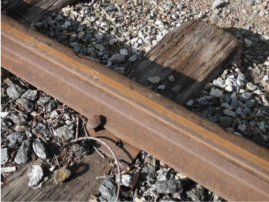
411.97 NW rail section loss
