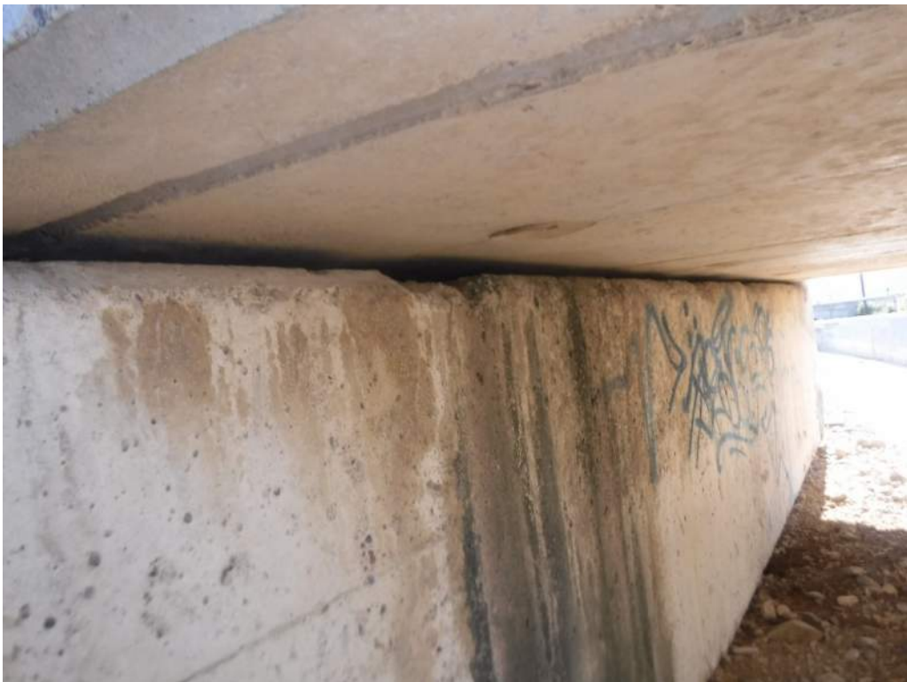
425.15 Abutment 3 Cap Spall
