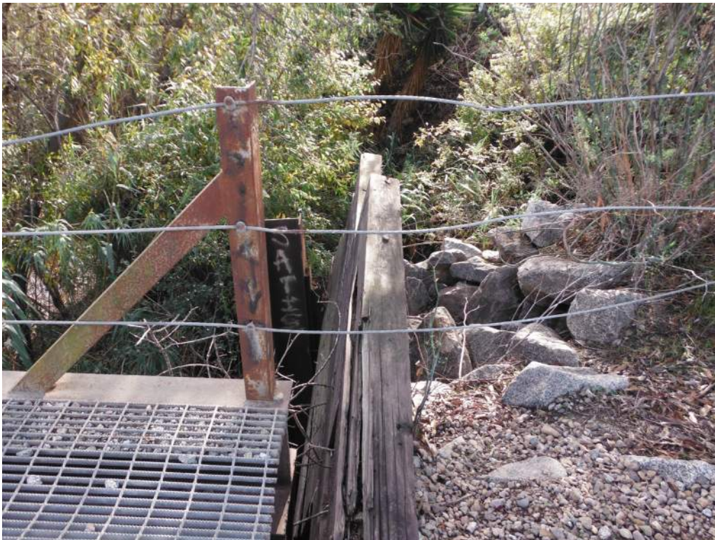
408.84 Abutment 1 backwall leaning
