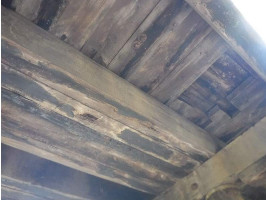
417.24 Stringer 2 failed, Stringer 3 rotten with 3" hole depth, Span 3
