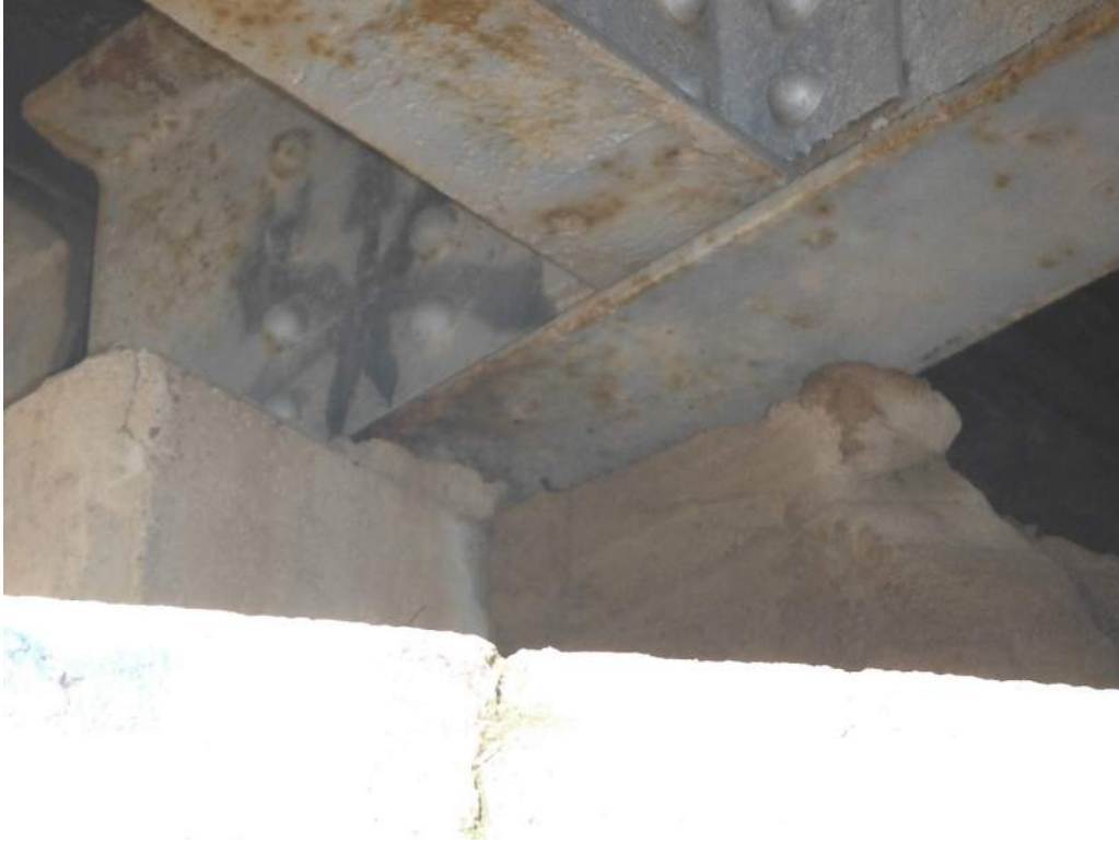
429.79 Miss punched holes in flanges. Multiple members, Span 2
