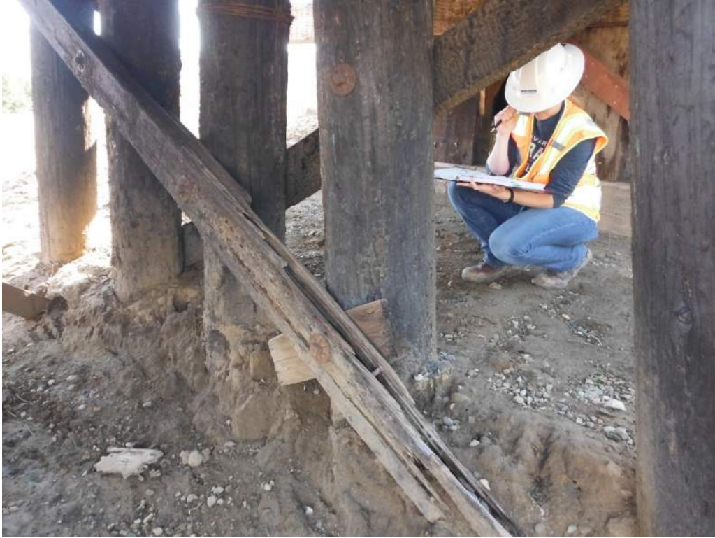
420.20 Span 2 sway brace rotten
