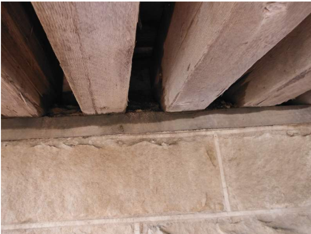
418.02 Debris and moisture on sill plate
