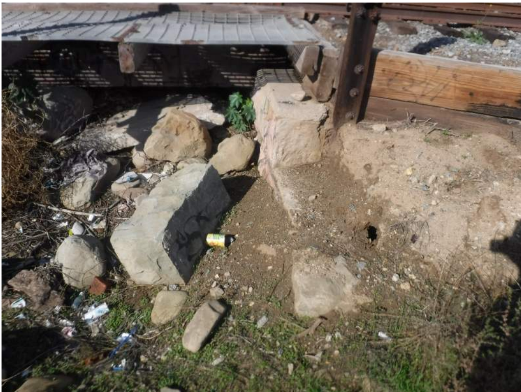
415.32 SE abutment stone block dislodged
