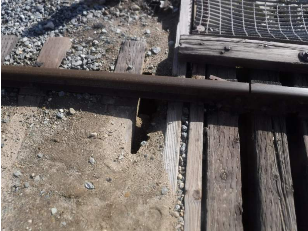
415.32 Hole in soil behind Abutment 2
