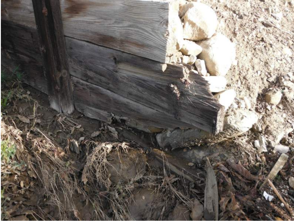
416.63 Backwall rotting/leaking material at bottom (Typ.)
