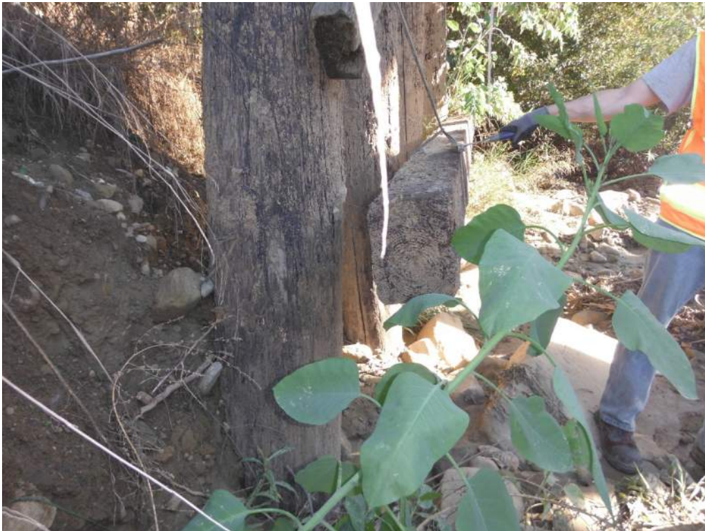
420.46 Diagonal sash bracing is not attached, Bent 4
