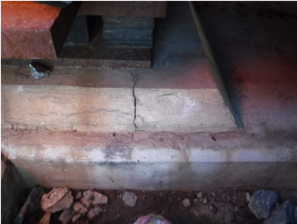
415.59 Grout pad cracked under bearing, Pier 2
