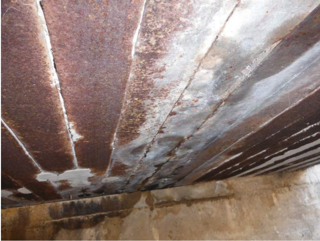
422.89 Efflorescence on rail top superstructure
