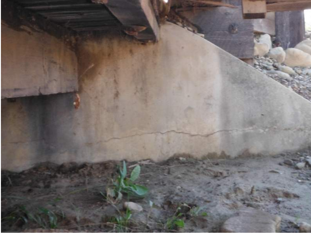
421.23 Horizontal Crack in North Side Abutment 1
