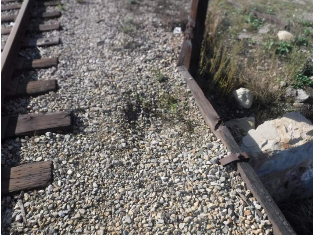
415.20 Holes in ballast on west side
