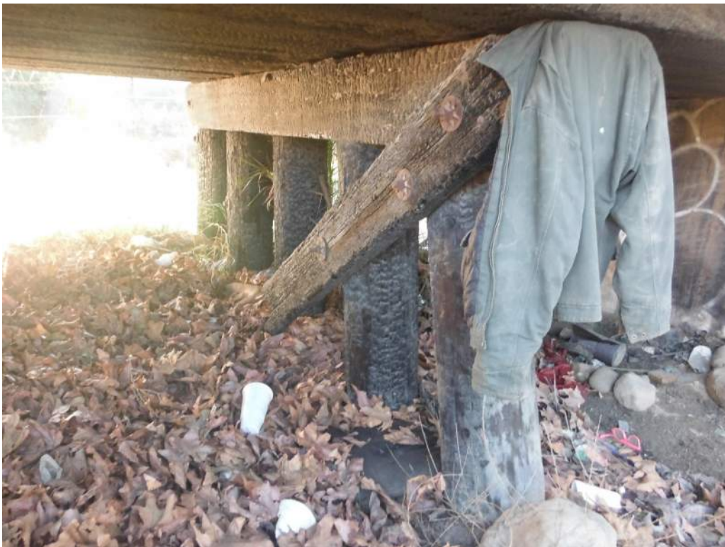
415.82 Failed sway brace – pier 2
