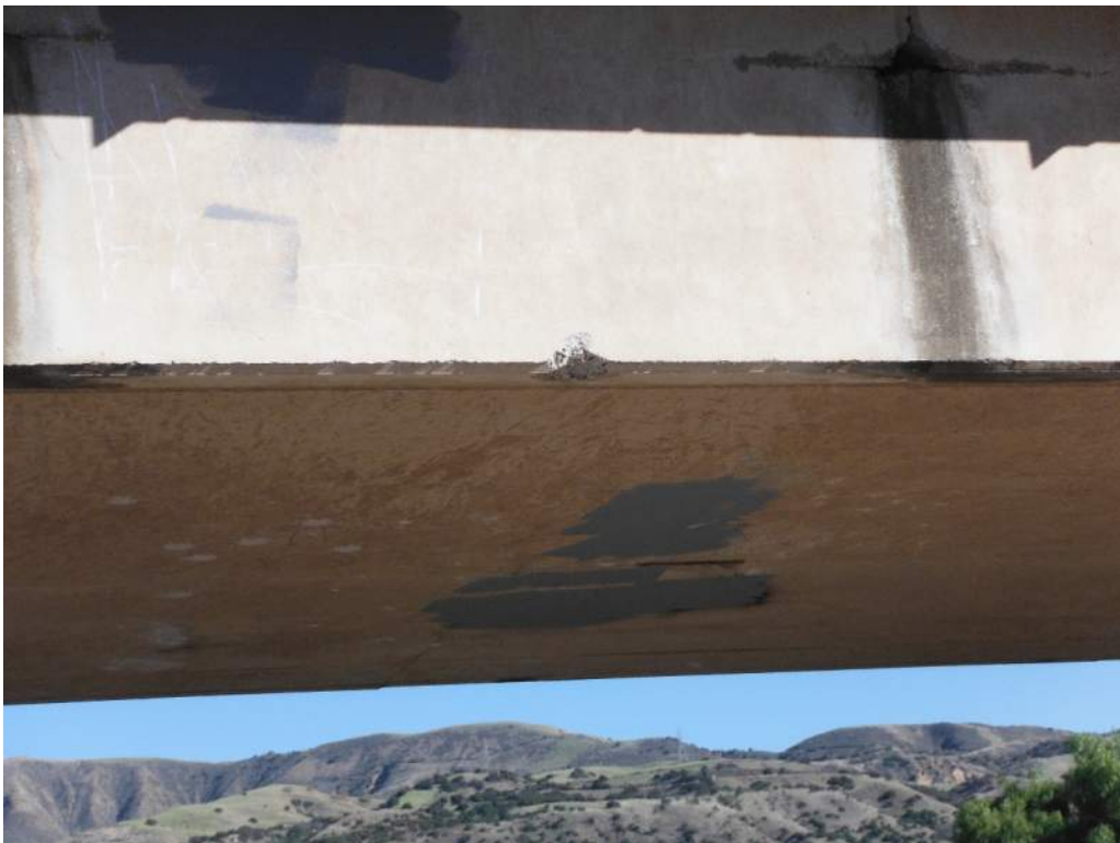
423.44 Minor spall midspan, Span 11
