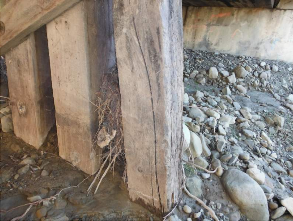
421.05 Vertical split in Pile 1 – Bent 2
