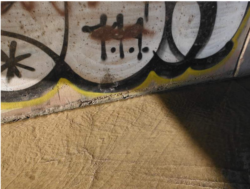
408.02 Scaling at base of Abutment #1
