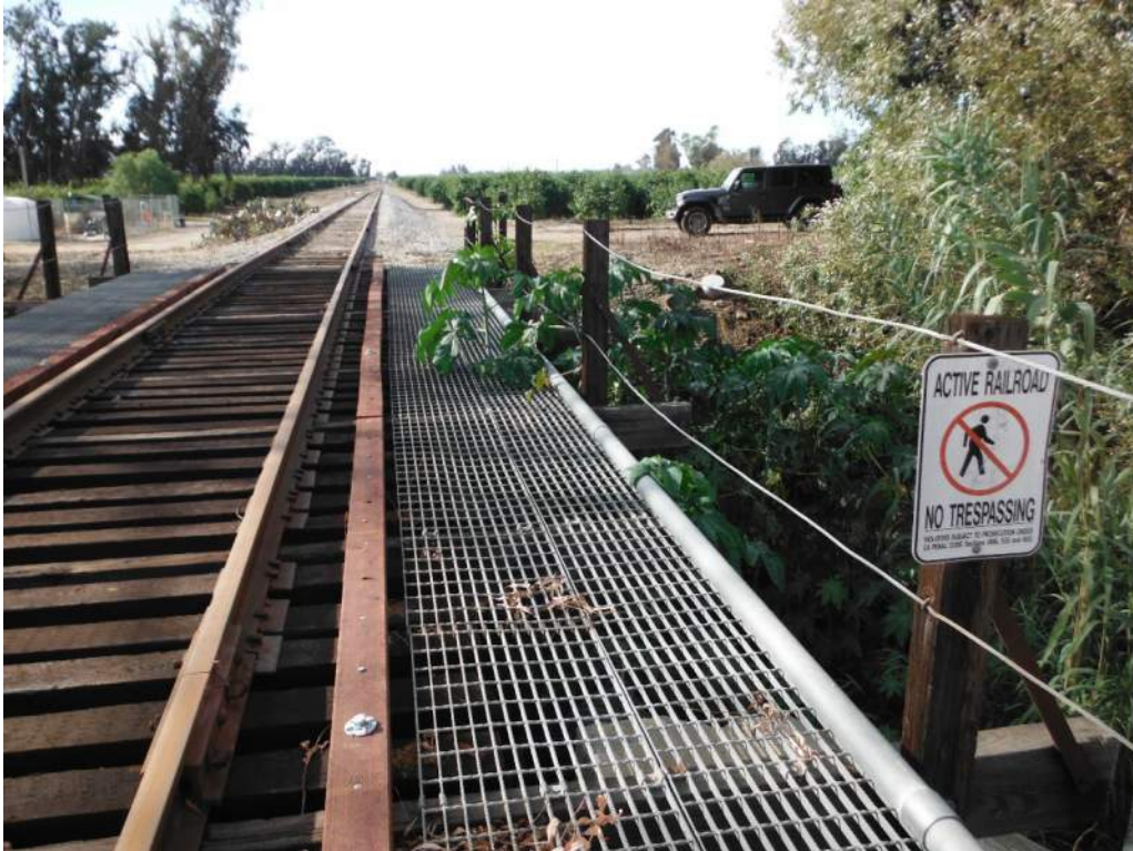
410.40 Loose handrail cables (Typ.)
