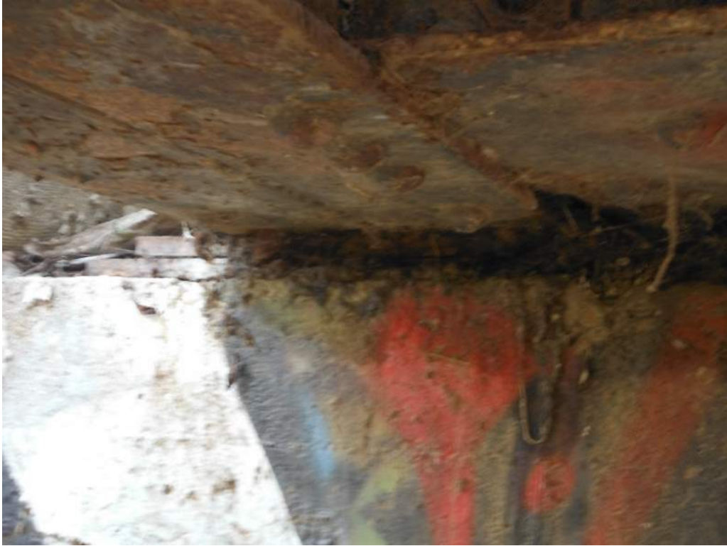
412.25 Pack rust at bearing plates (typ.)
