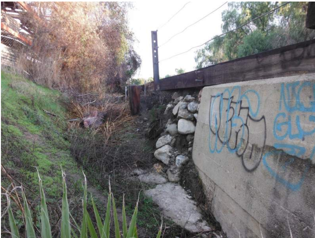
407.48 NE Wingwall Erosion
