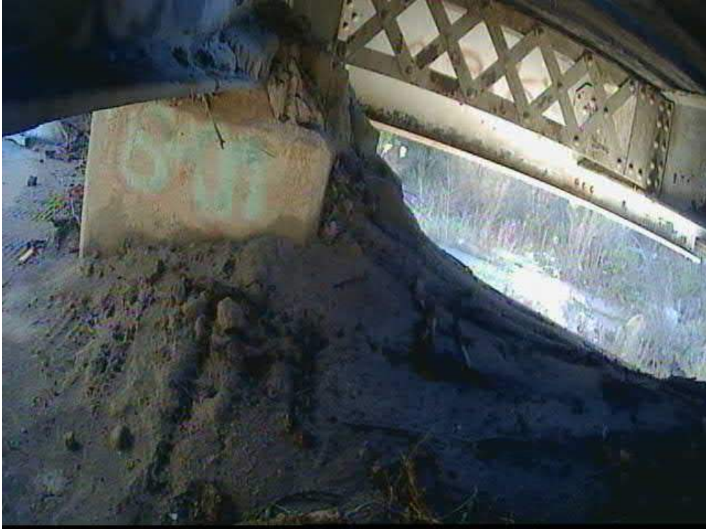
429.79 Seats are covered with silt, Pier 2 Bearing
