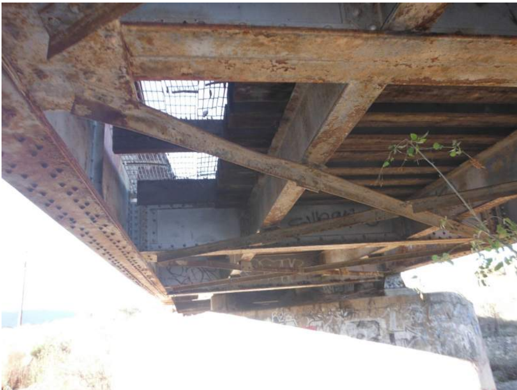
429.79 Lower cross bracing has minor impact throughout
