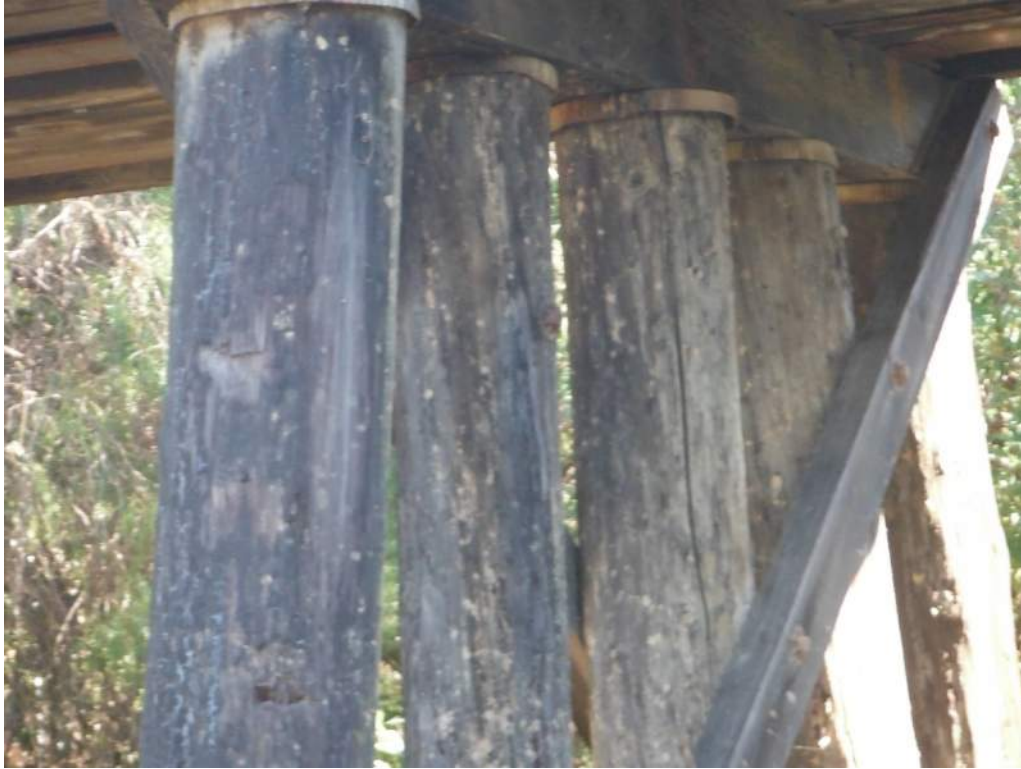
420.46 Pile 3 is punky and has a vertical split, Bent 4
