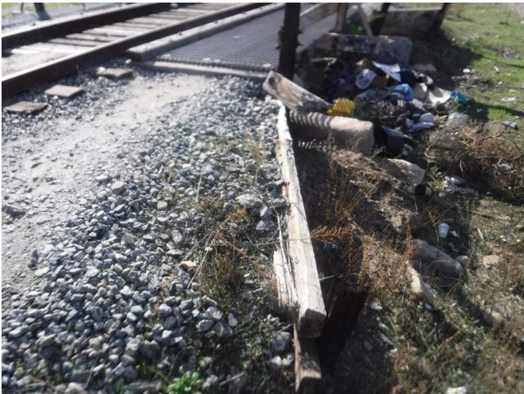
415.32 Wingwall failing, typ all corners
