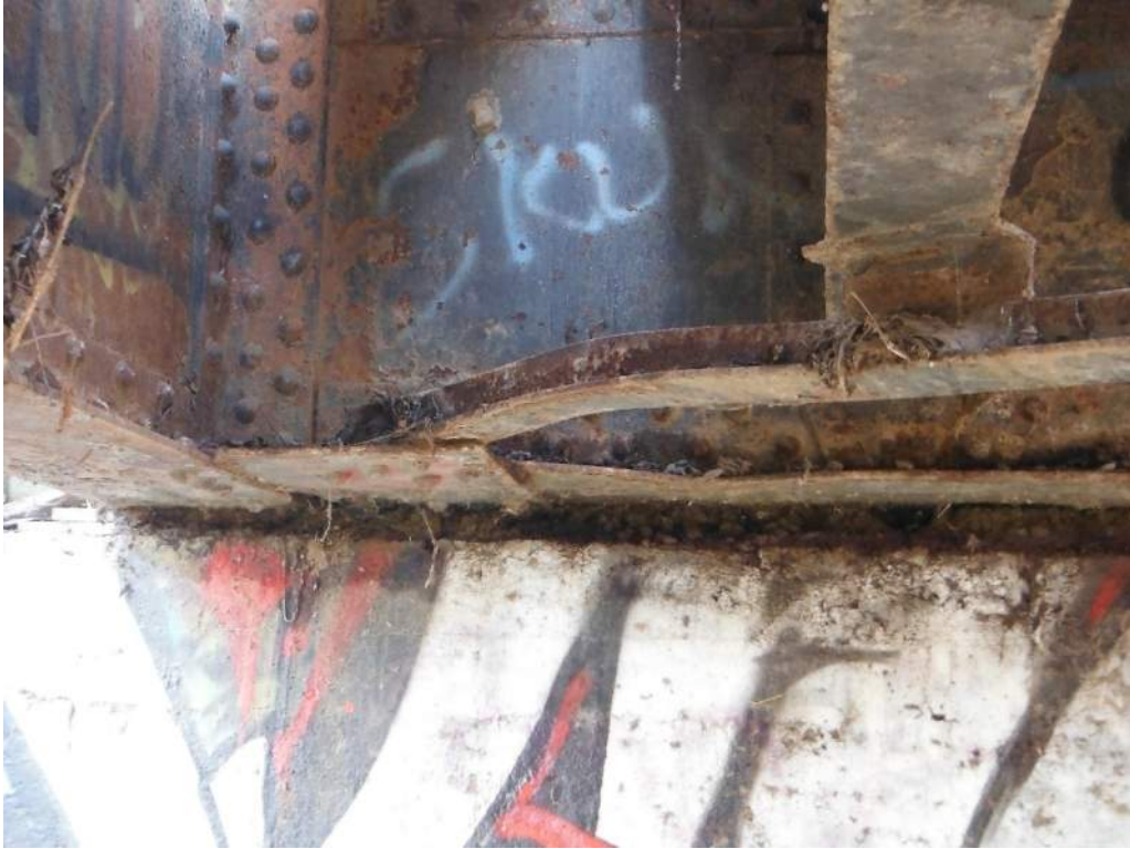
412.25 Minor impact damage near Abutment 1
