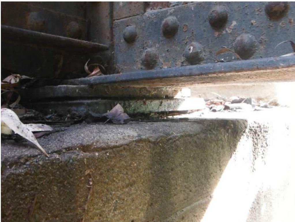
410.40 Debris around bearings. Abutment 1 & 2
