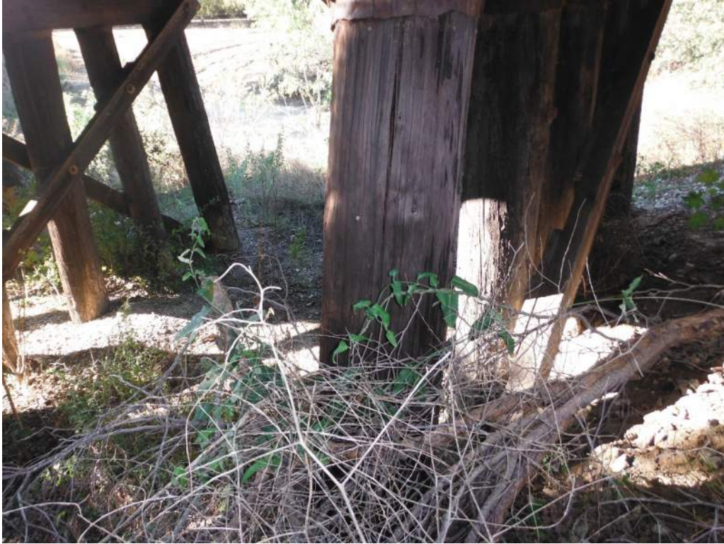
420.46 Pile 5 vertical split, Bent 6
