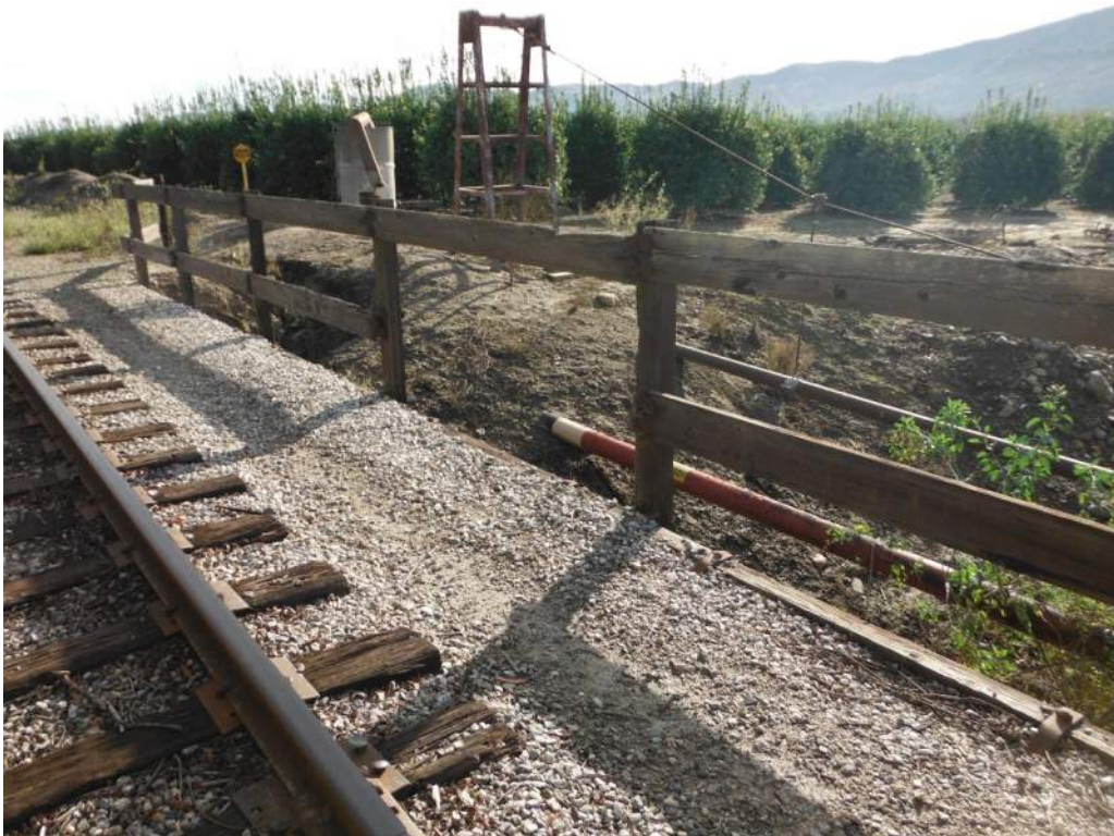
417.24 Handrail mid-rail failed in two locations
