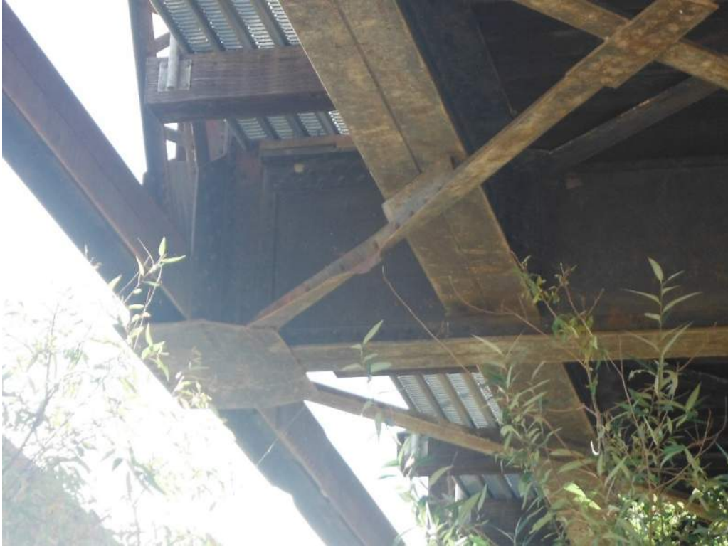
415.59 Minor impact damage – typical bottom cross bracing
