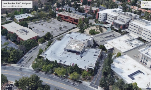
Aerial Image of Existing Heliport at Los Robles Regional Medical Center
